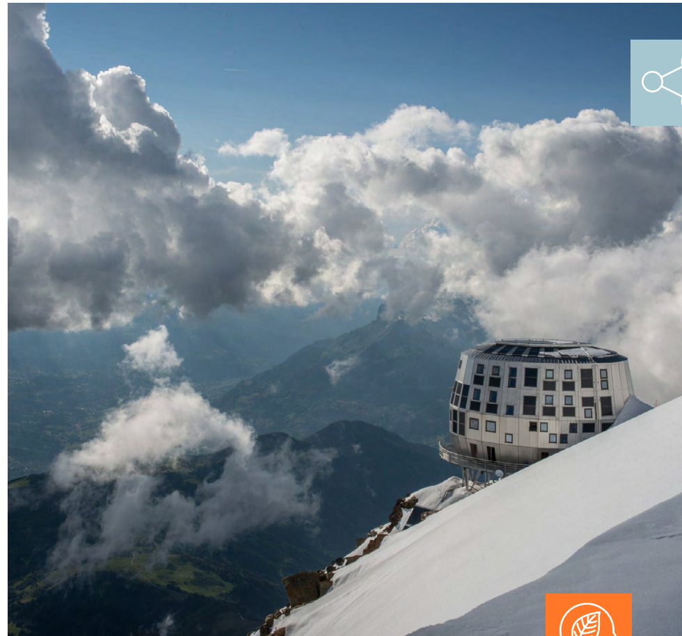
Refuge du Goûter is the highest mountain refuge in the Alps, close to the summit of Mont Blanc. Located at 3,800 M, it routinely faces extreme conditions. Distech Controls was called in to implement an interoperable, sustainable, optimized, reliable solution open to the latest connected technologies.
