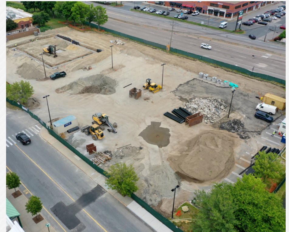
OUTPARCEL CONSTRUCTION AT SHOPPERS WORLD FRAMINGHAM, MASSACHUSETTS
