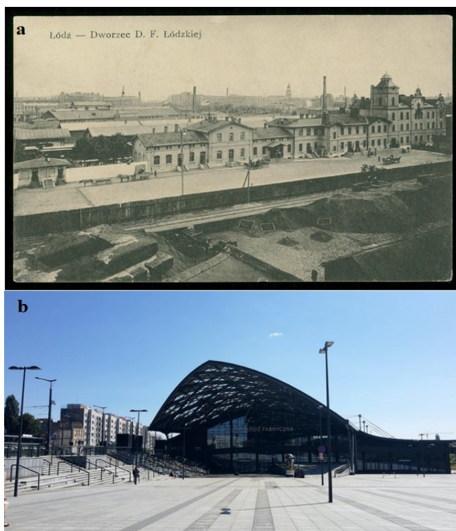
Fig. 7. Łódź Fabryczna railway station: a. postcard from the beginning of the 20th century (Polish National Library, Public Domain, ref. DŻS XII 8b/p.10/14); b. Current appearance of the Łódź Fabryczna railway station. Photo by: D. Rutkowska-Siuda
