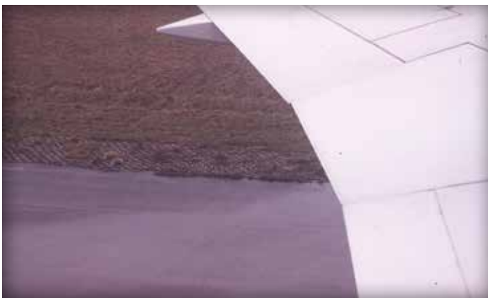
Figure 11. Airfield taxiway shoulder
