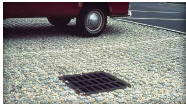
Figure 16. Concrete grids with aggregate in the openings
