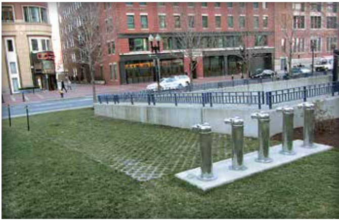
Figure 7. Emergency access lane for fire trucks
