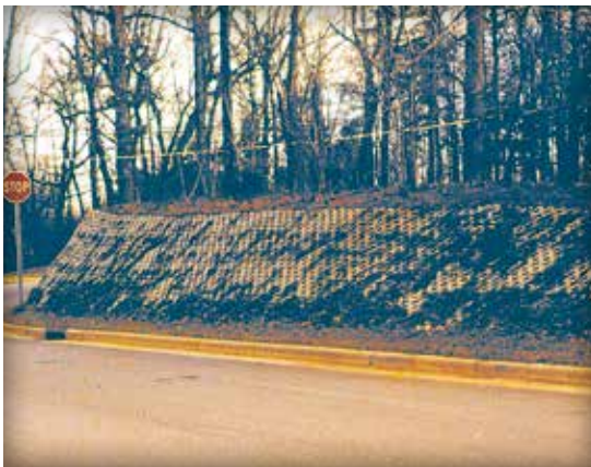
Figure 9. Embankment stabilization
