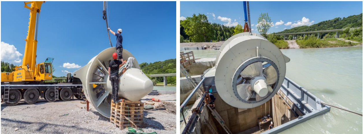
Figure 7: Mounting of the turbine in the dry shaft. (Ch. Bäck/TUM)
