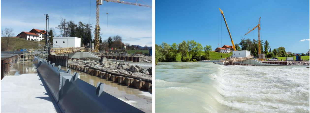
Figure 6: Hydraulic stands on top of the former block ramp, after mounting (left) and with overflow (right). (Ch. Bäck/TUM)
