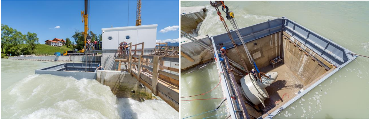
Figure 8: Mounting of the turbine in the dry. (Ch. Bäck/TUM)
