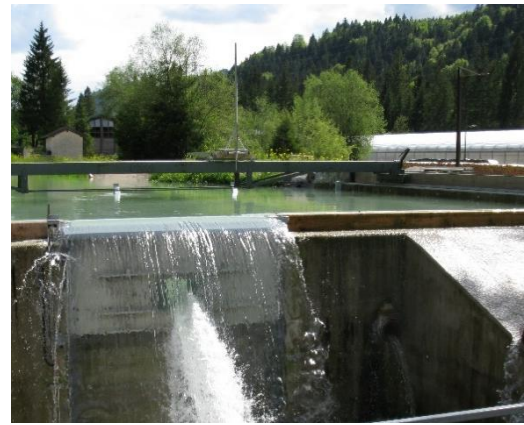
Fig. 5: Prototype plant with technology building (l.), overfall with fish descent window (r.)
