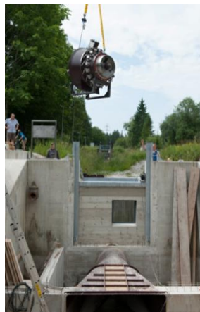
Fig. 6: Turbine installation (l. & m.), view from the Shaft to the top (r.)
