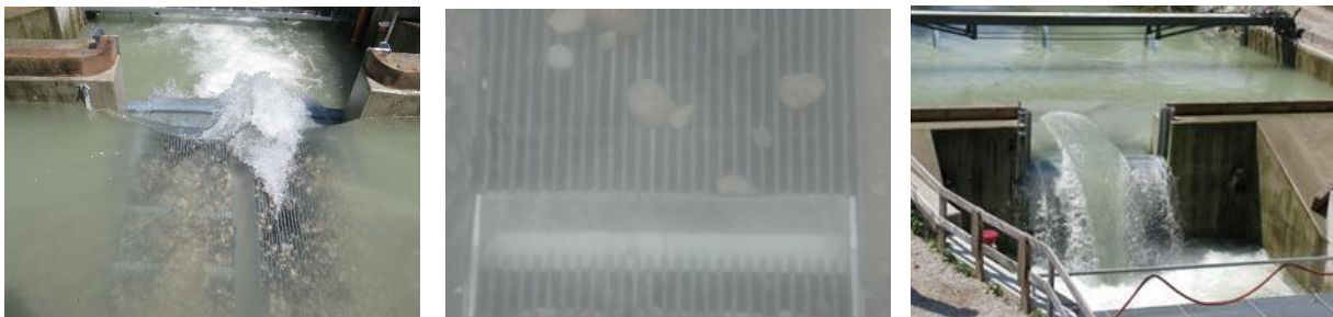
Fig. 7: Sediment flushing with the assistance of the rack cleaning
