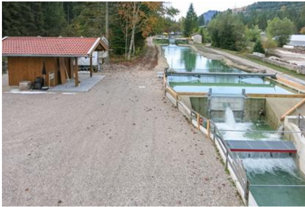
Fig. 5: Prototype plant with technology building (l.), overfall with fish descent window (r.)
