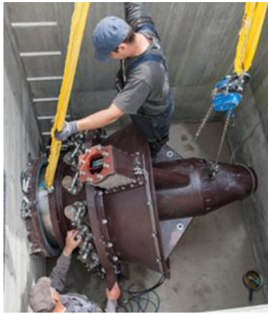
Fig. 6: Turbine installation (l. & m.), view from the Shaft to the top (r.)
