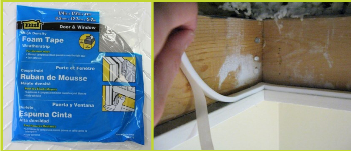
Example of commonly used insulation and where to install. Foam weather-strip is considered single-use. Once you've opened the hatch, you must replace the strip.
