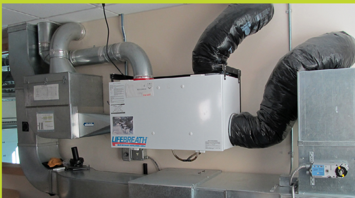
An example of an HRV system you may see in a home.
