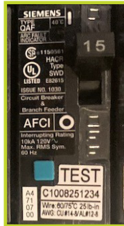
Breaker with Arc Fault Circuit Interrupter
