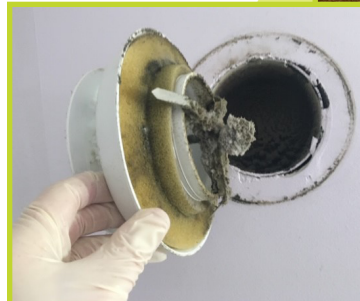
Rinse the cover in the tub/sink to remove any loose dust from the inside.
