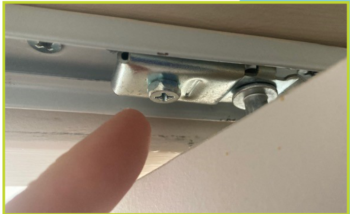
Using a multi-bit screwdriver is necessary to set the top screw that keeps the door aligned.
