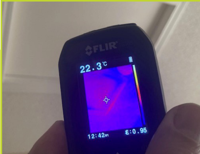
Thermal imaging of an attic. Note: dark purple coloring indicates colder area. Air leak? 0° outside, 20° inside.
