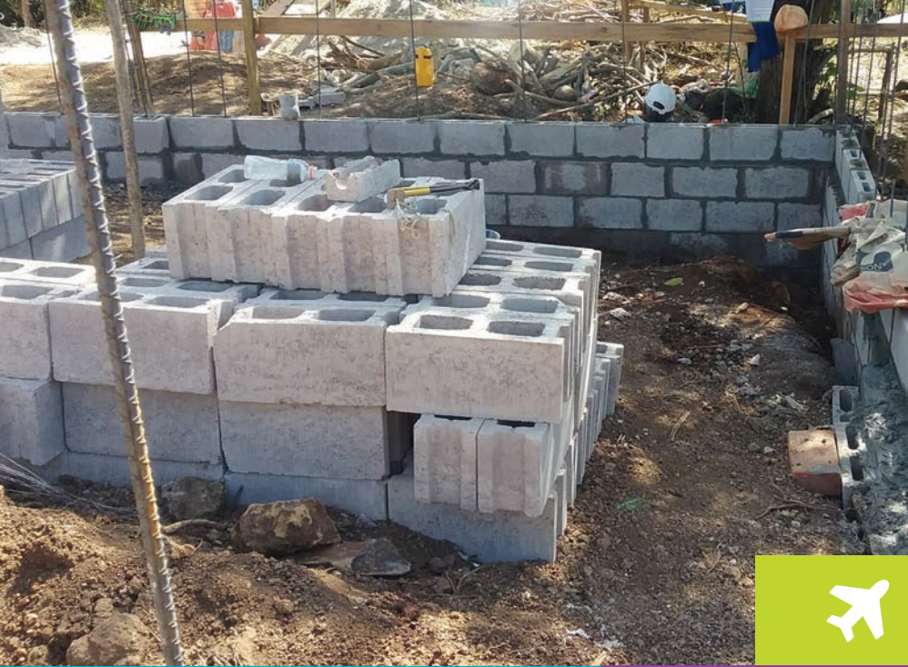
A 2019 Global Village build site in El Salvador.
