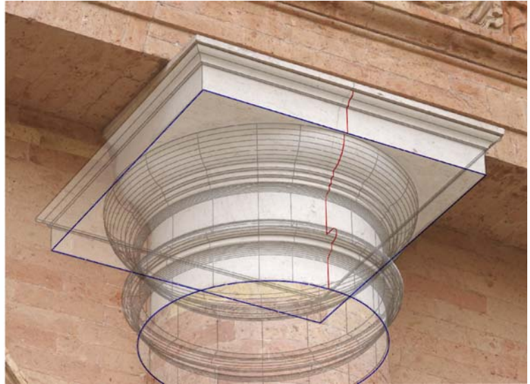
Fig. 19a,b. The primitive instantiated on the point cloud. On the left b , the vertical profile with dimensional information. On the right a , the primitive projected on a photography oriented on the point cloud
