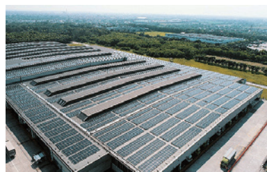
Solar panels installed at TMMIN
