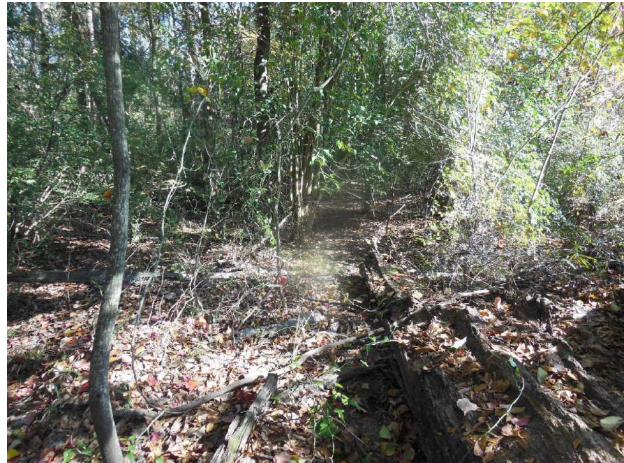
DITCH ADJACENT TO NORTH SIDE OF ROBIQUE ROAD 2
