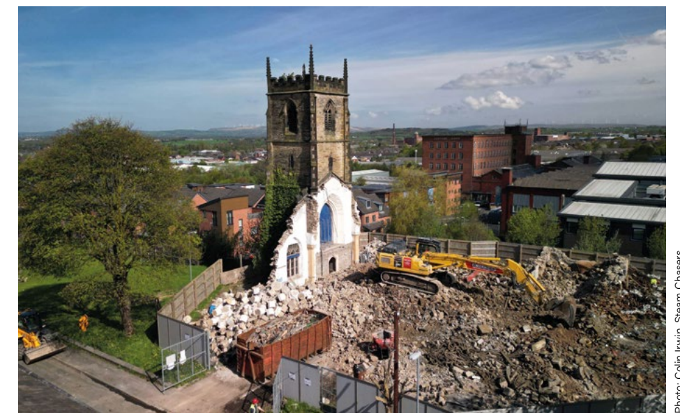
St John's Werneth, which was demolished in May 2023
