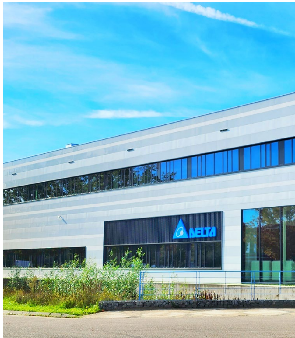
▲ Delta's LEED Gold-certified green building at the Automotive Campus in Helmond, the Netherlands
