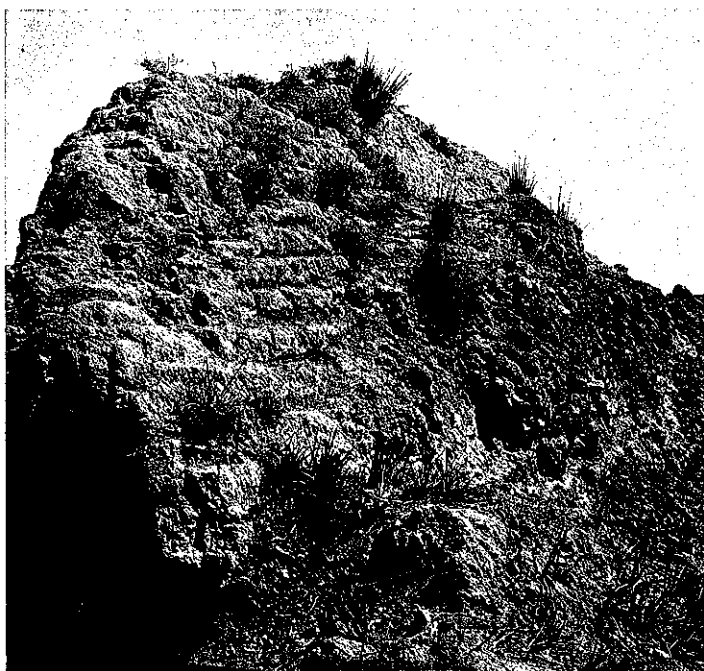
RETAINING WALL INSIDE STUCCO SLOPE.
