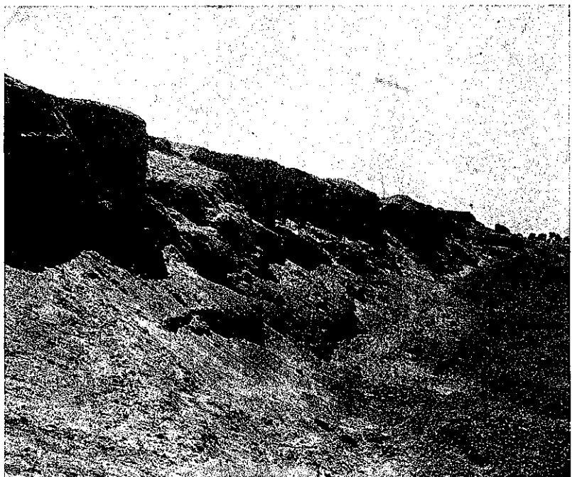
INNER SIDE OF SAND EMBANKMENT.
