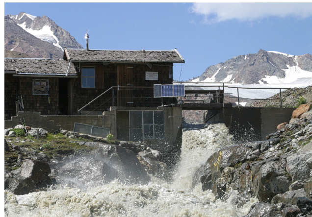
Figure 13. The Vernagtbach gauging station in 2006 (2635 m a.s.l., 46.85675° N, 10.82886° E), view to the northwest. Photo by Ludwig Braun.
