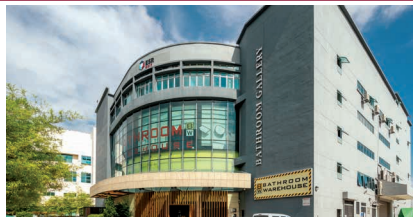
2 25 Changi South Avenue 2
