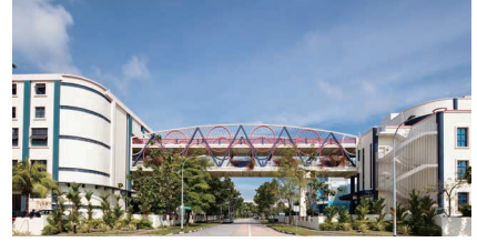
6 1 & 2 Changi North Street 2
