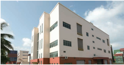
4 79 Tuas South Street 5
