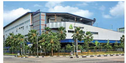
3 81 Tuas Bay Drive
