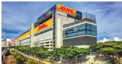
14 1 Greenwich Drive (DHL Supply Chain Advanced Regional Centre)
