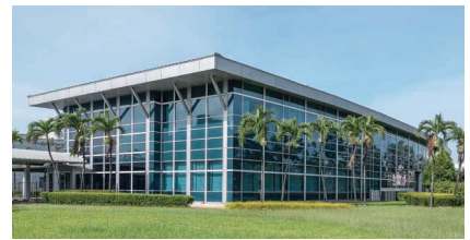
15 3 Tuas South Avenue 4
