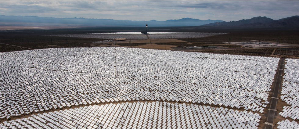
At the Ivanpah Solar Electric Generating System in California, 300,000 mirrors track the sun in two dimensions and reflect the sunlight to boilers atop three tall power towers. Photo by National Renewable Energy Lab (CC BY-NC-ND 2.0)
