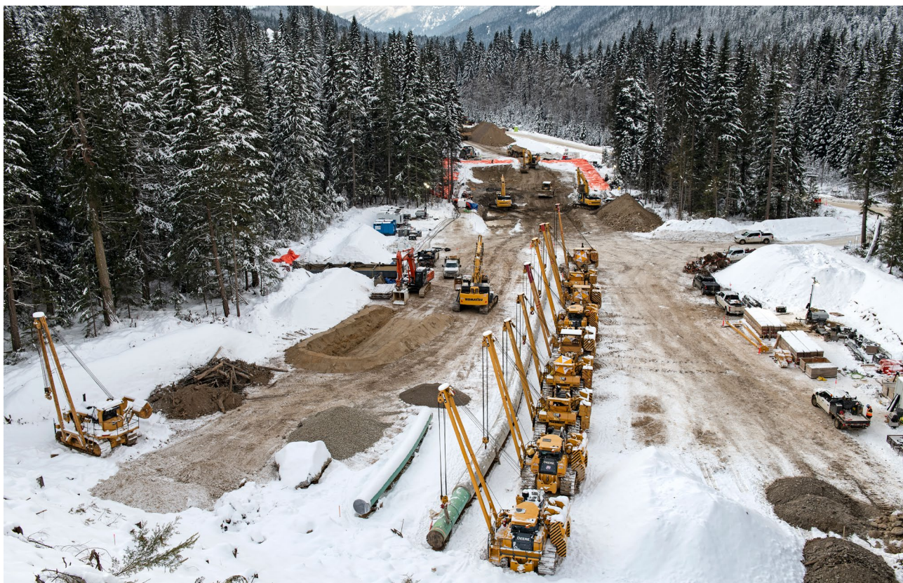
BELOW: Construction continues to advance even in challenging weather conditions.
