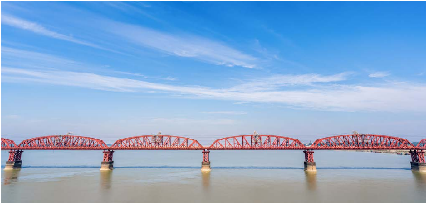
Hardinge Bridge over the Padma River (Ganges) in Bangladesh
