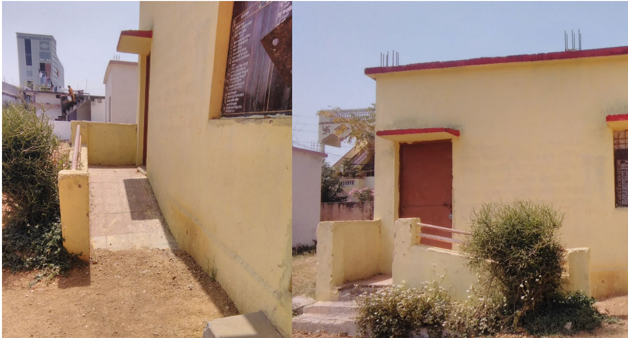
FIGURE 7.B. THE GANDHI SCHOOL, INDIA, WITH AN ACCESSIBLE CLASSROOM ENTRANCE INSTALLED
