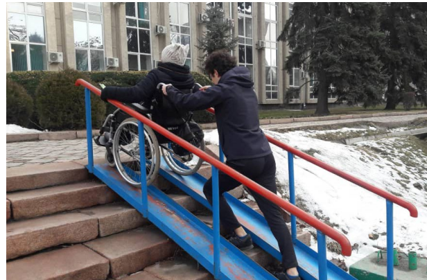
FIGURE 7.1. A WHEELCHAIR USER REQUIRING ASSISTANCE ON A RAMP THAT IS NOT USER-FRIENDLY
