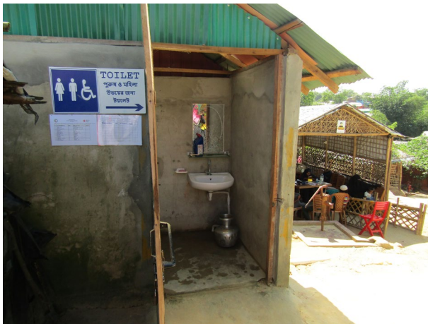
FIGURE 7.G. TOILET FACILITIES MADE ACCESSIBLE
