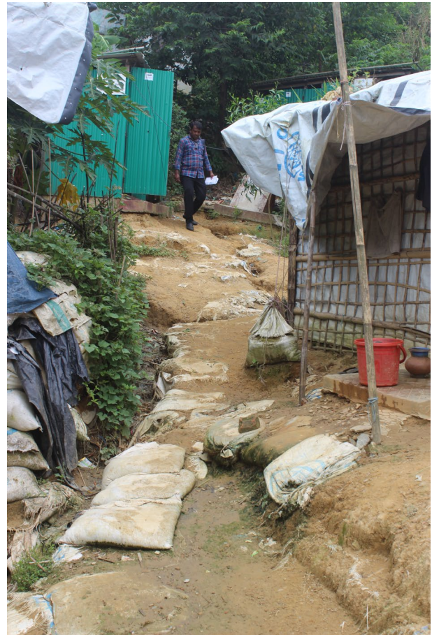
FIGURE 7.F. UNEVEN GROUND IN REFUGEE CAMP
