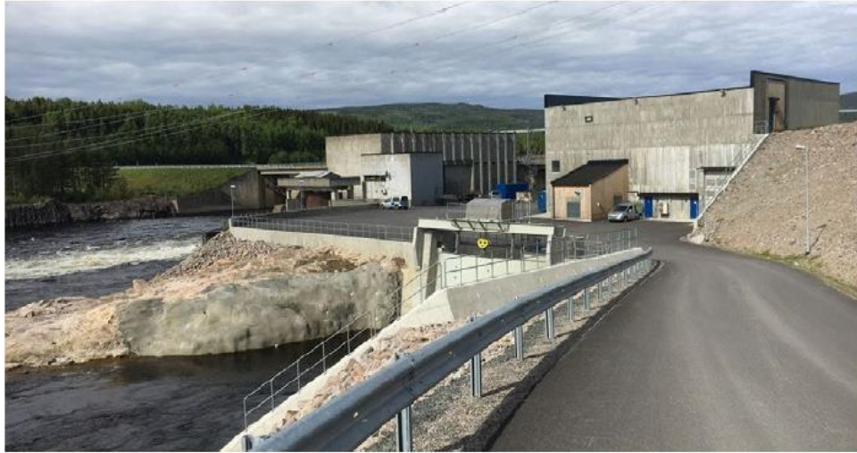
Photo 3: Braskereidfoss Power Station. Generator 1 is in the building on the left, generator 2 is in the building on the right (Photo: HEV)
