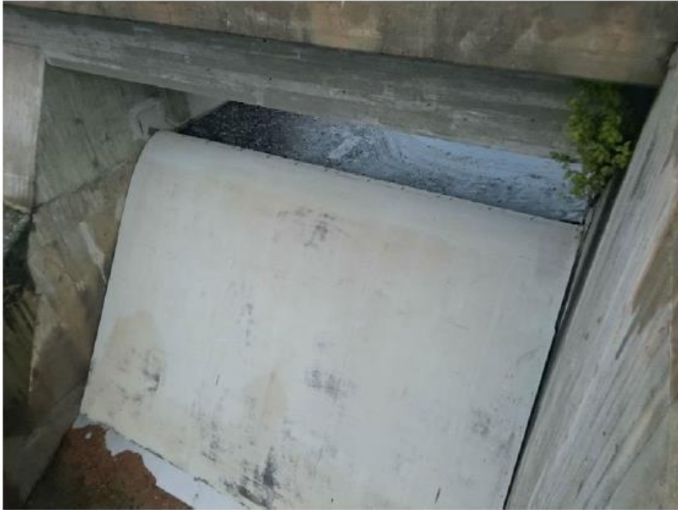
Photo 7: Timber gate (Photo: Sweco)
