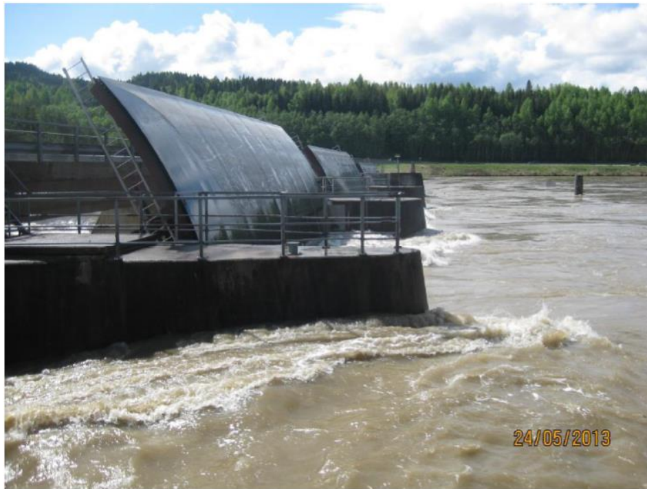
Braskereidfoss Power Station during spring flood, May 2013. Rate of flow approx. 2100 m 3 /s.
