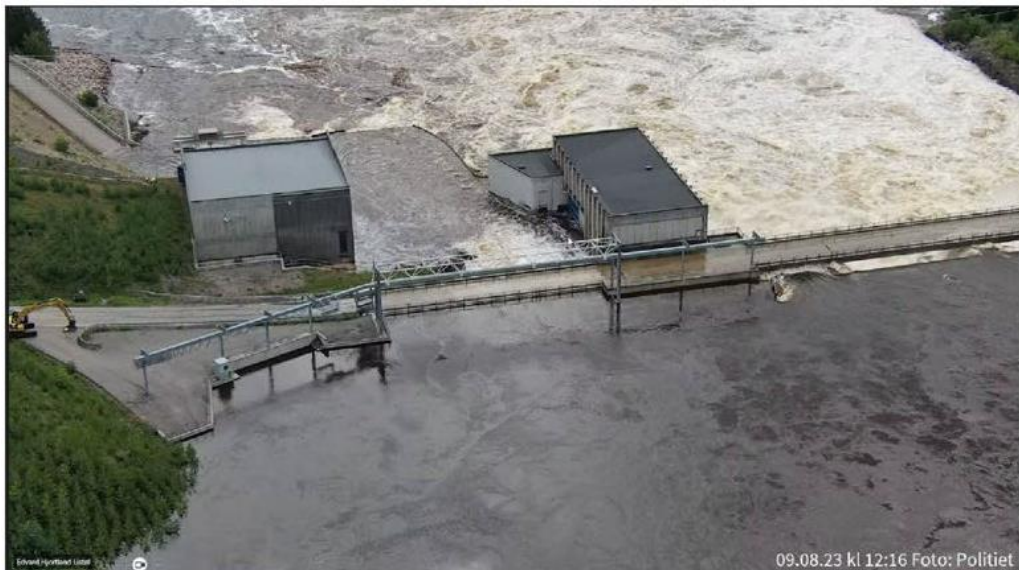
Photo 1: Braskereidfoss Power Station, 09/08/2023 at 12:16. The water is flowing over the floodgates and the buttress dam and into the two power plants (Photo: Police/Source NVE).
