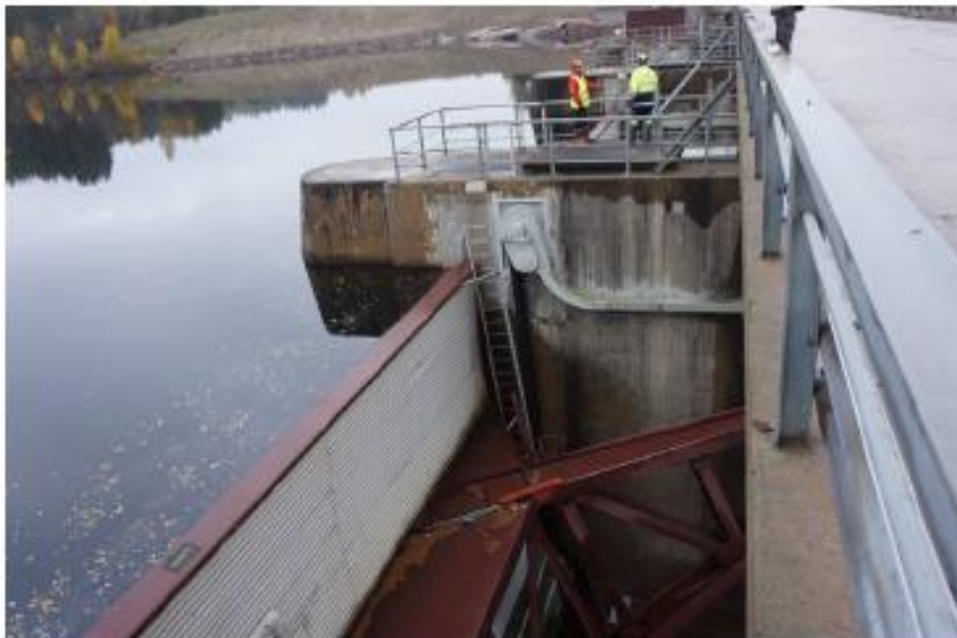
Photo 6: Floodgate, pillar and gatehouse (Photo: Sweco)
