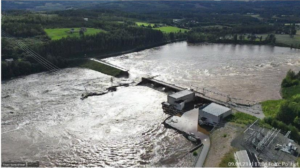
Photo 13: After the failure of the embankment dam at 17:04 (Photo: Police/Source NVE)
