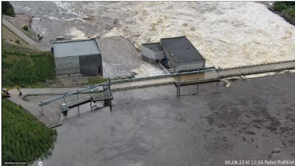
Photo 11: Power plants and gated dam at 12:16 (Photo: Police/Source NVE)
