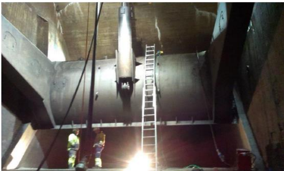
Photo 8: Bottom gate (Photo: Sweco)
