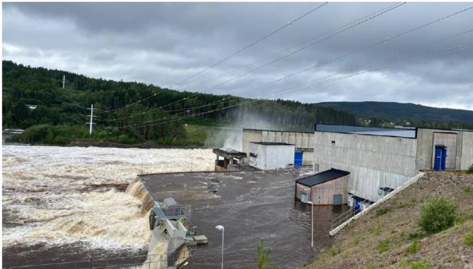
Photo 9: Braskereidfoss Power Station, morning of 09/08/2023 (Source HEV)
