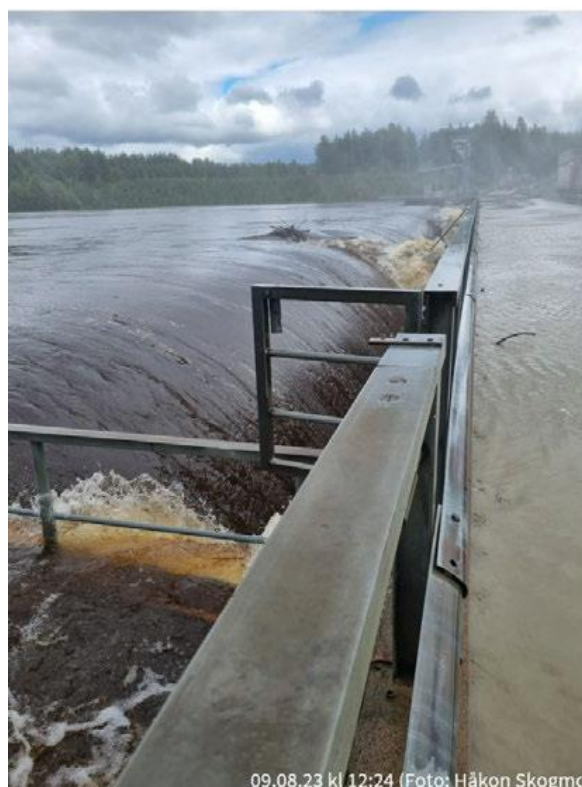
Photo 10: Overtopping of the floodgates at 12:24 (Photo: Håkon Skogmo/Source NVE)
