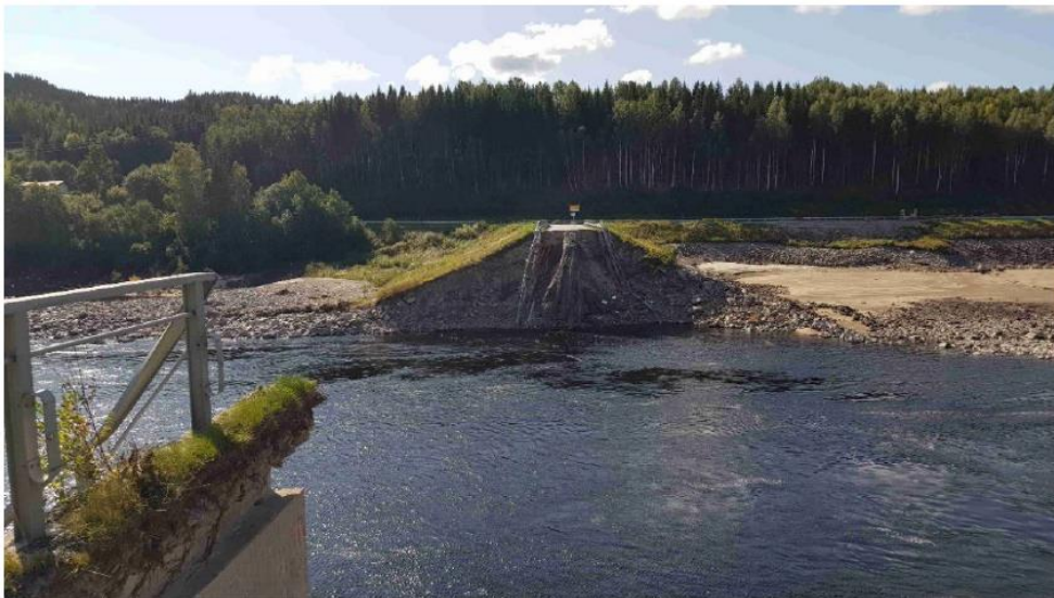
Photo 14: Remains of the embankment dam after dam failure (photo: DNV)
