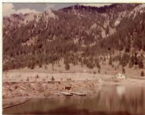
Fig. 4 FAULT IN NORTH ABUTMENT
