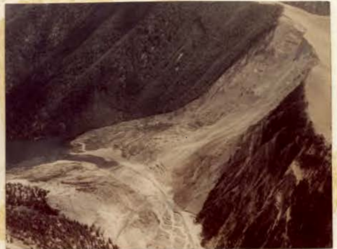
Fig. 19 AIR VIEW OF LANDSLIDE, LAKE, AND EXCAVATED SPILLWAY
