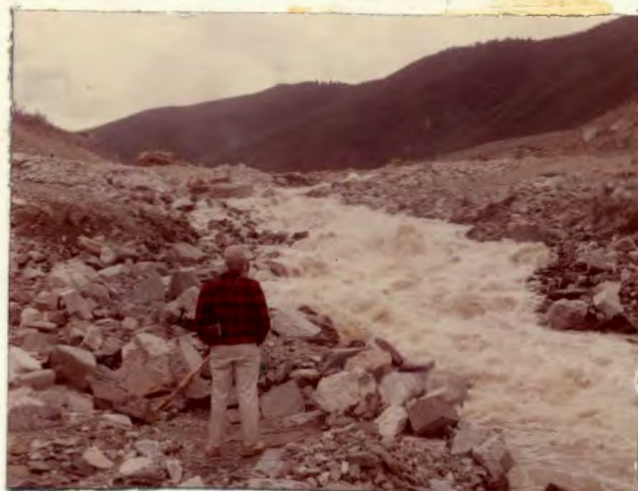
Fig. 22 CHUTE SECTION OF SPILLWAY
