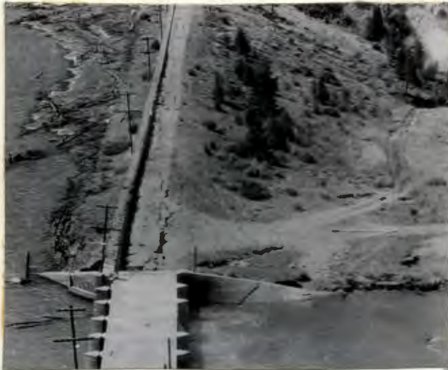
Fig. 7 HEBGEN DAM - AIR VIEW FROM RIGHT ABUTMENT (Montana Power Co. Photo)
