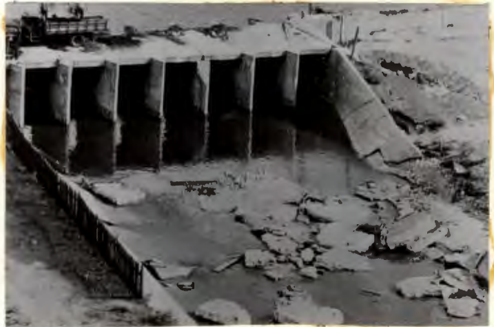
Fig. 10 SPILLWAY CONTROL STRUCTURE (M. P. Co. Photo)
