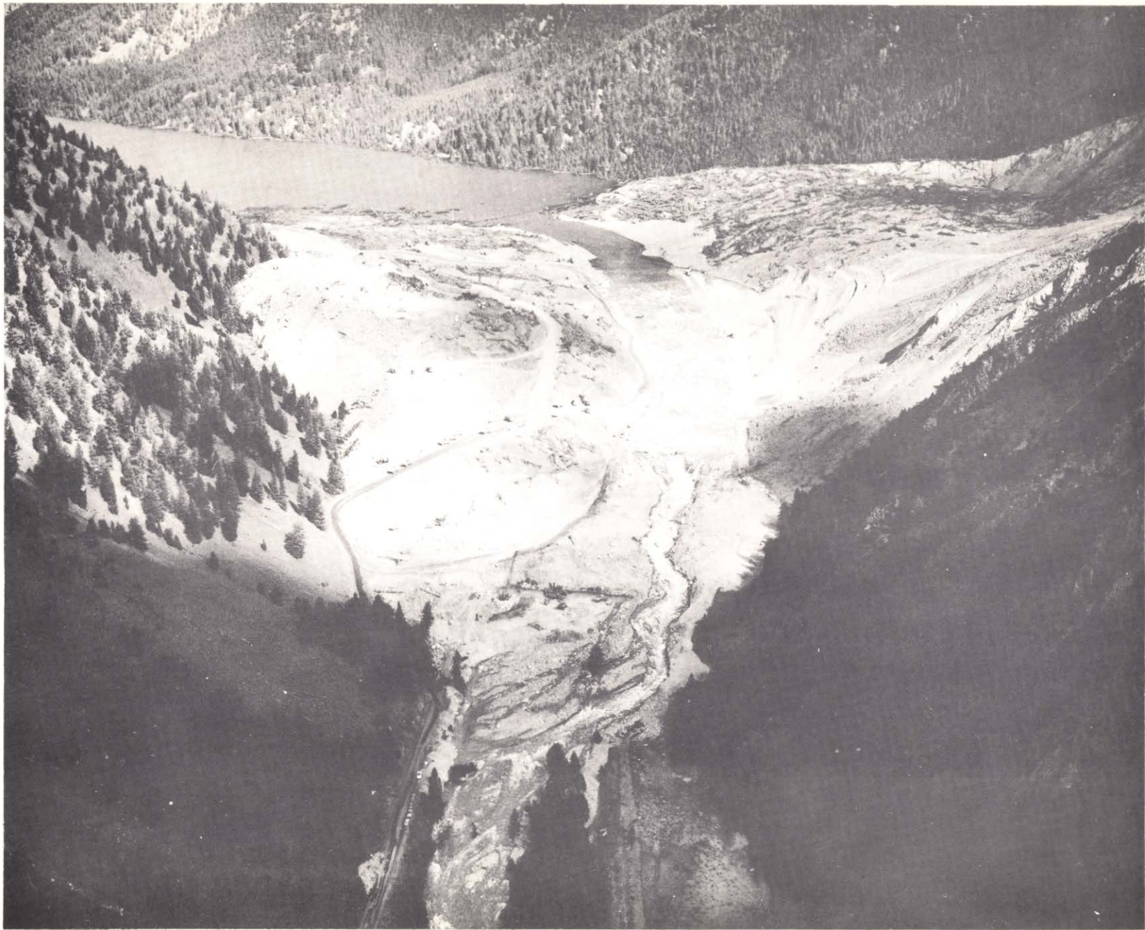
Photo 12. 16 September 1959. Aerial view of slide and spillway.
