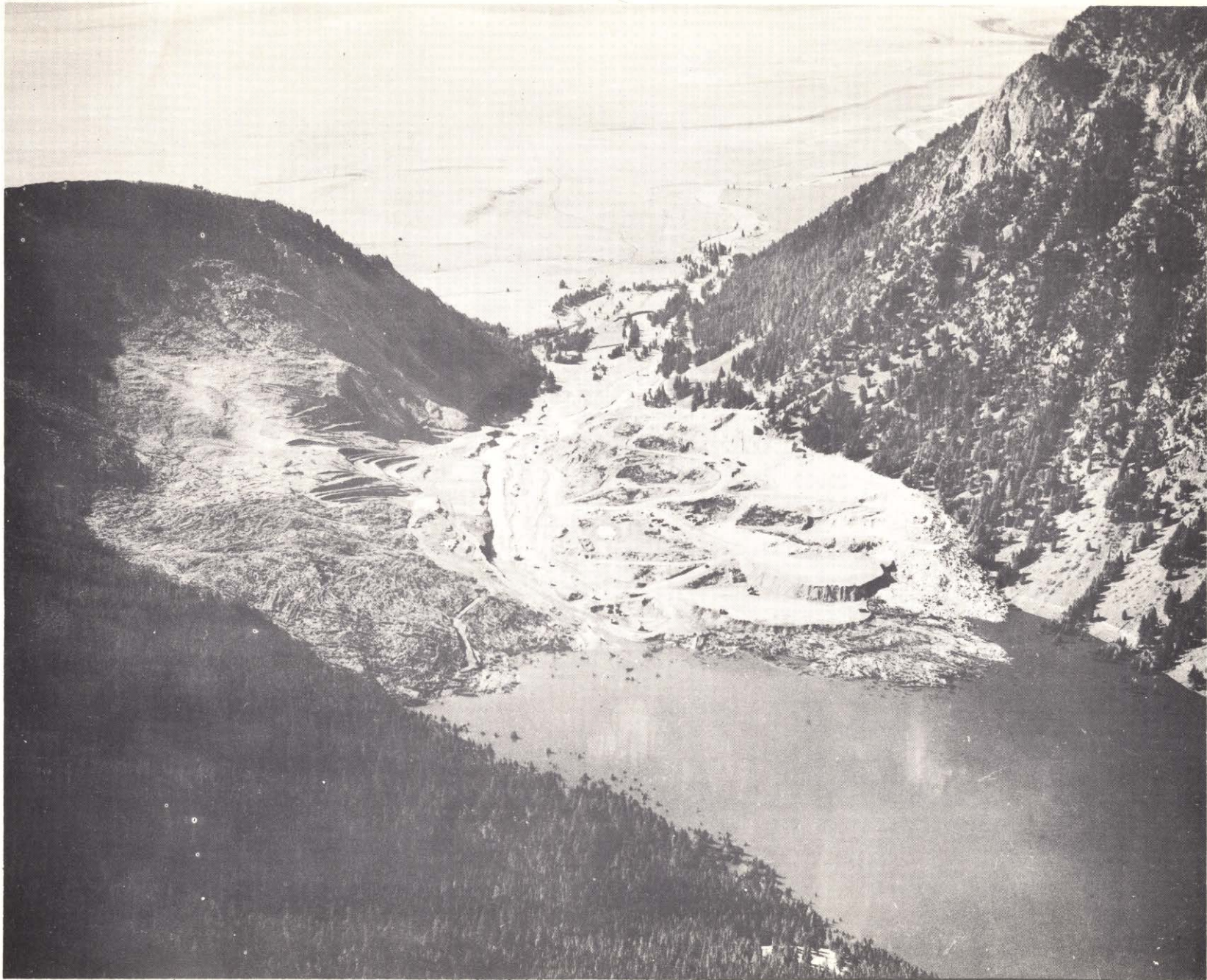
Photo 23. 17 October 1959. Aerial view of slide looking downstream.
