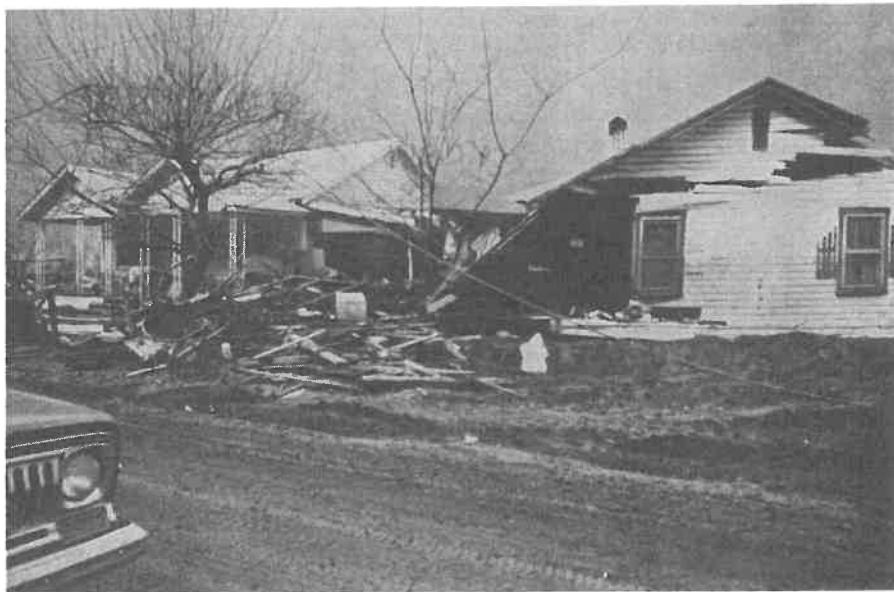
FIGURE 19 Homes 10 Miles Below Dam.
