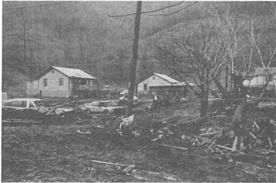
FIGURE 22 Debris 14 Miles Below Dam.
