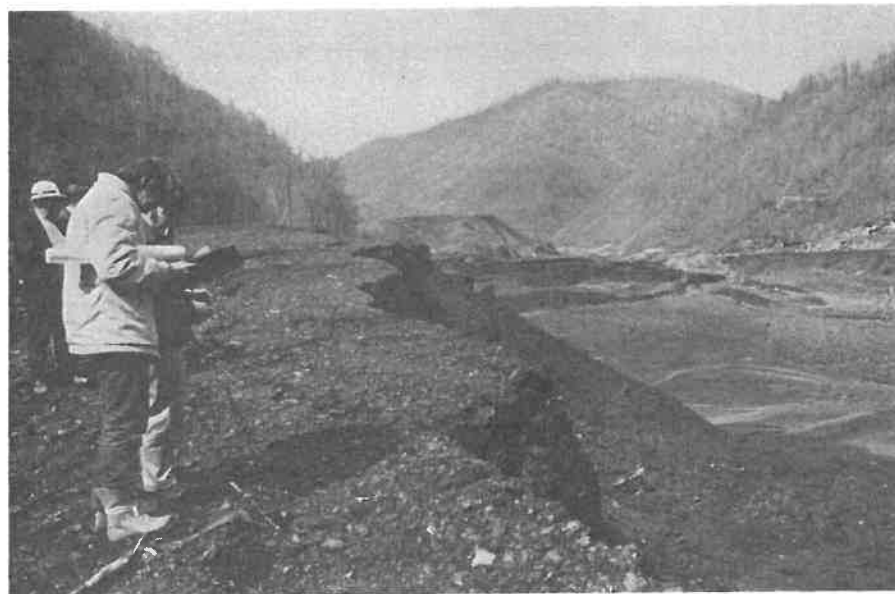
FIGURE 9 Looking Downstream from Left Abutment.
