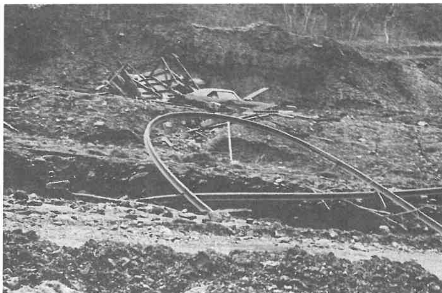
FIGURE 27 Bent Railroad Rails 5 Miles Below Dam.
