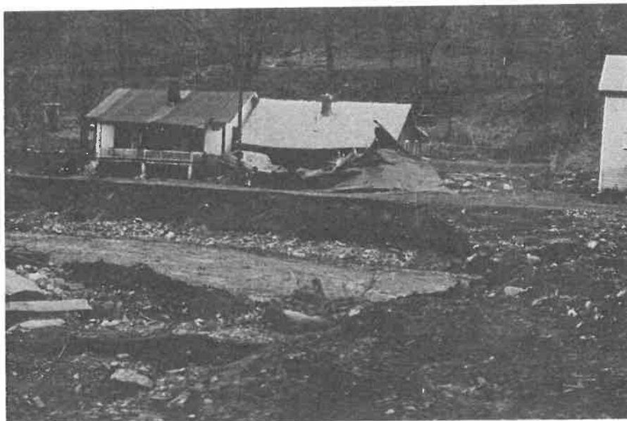
FIGURE 17 Home Removed from its Foundation and Damaged Automobile 5 Miles Below Dam.
