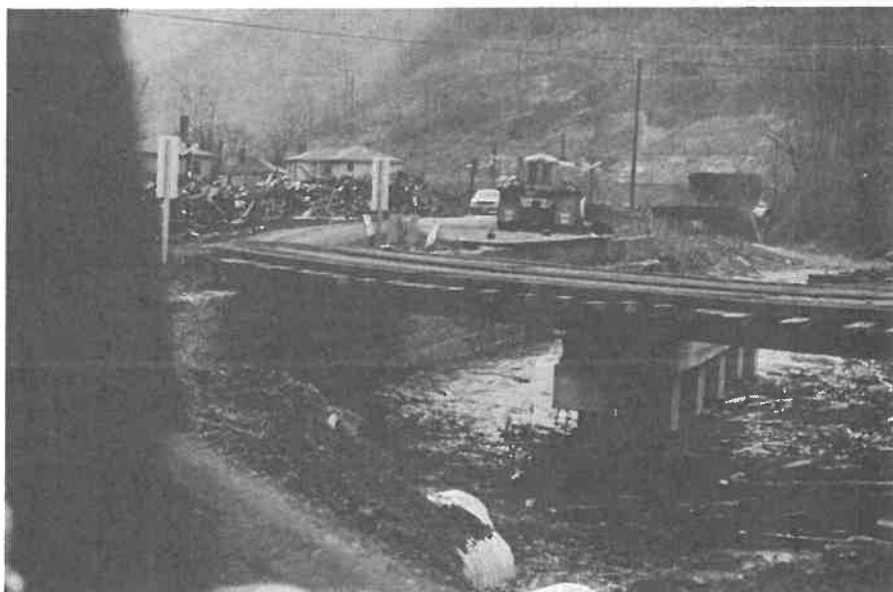
FIGURE 26 Temporary Bridge on Abutments of Destroyed Highway Bridge. Note Debris in Background.
