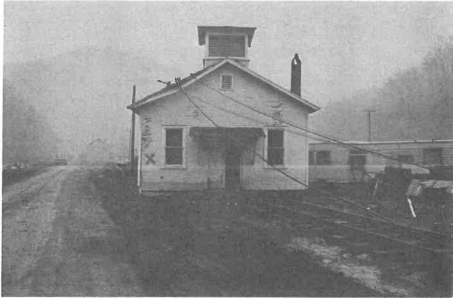
FIGURE 20 Church Removed from its Foundation. (X on Building indicates Condemned.)
