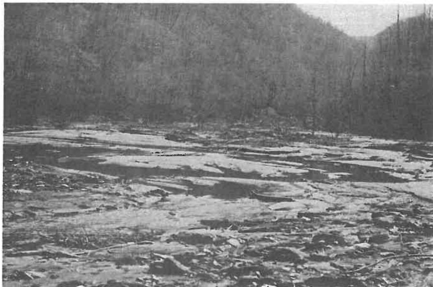
FIGURE 11 Looking Upstream at Reservoir Area from Center of Dam.
