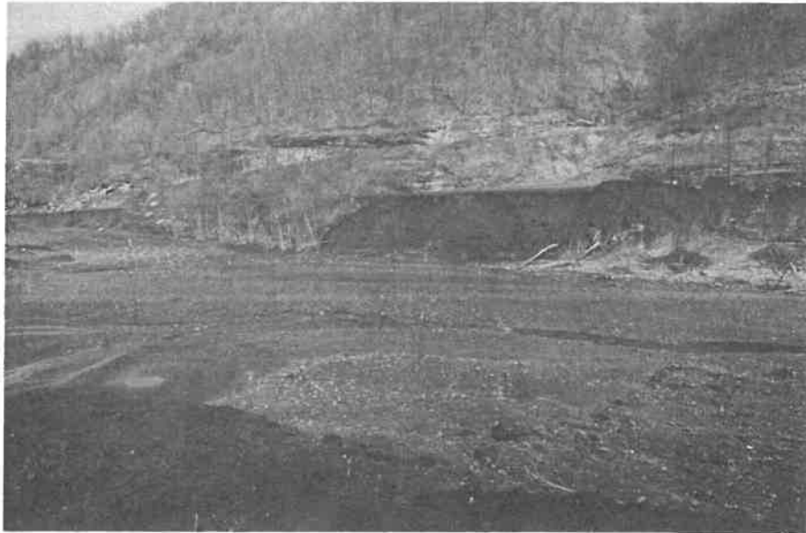
FIGURE 10 Looking at Right Abutment of Dam No. 3 from Left Abutment.
