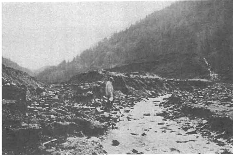
FIGURE 12 Looking up at Left Abutment. Dam No. 2 Formerly in Foreground.
