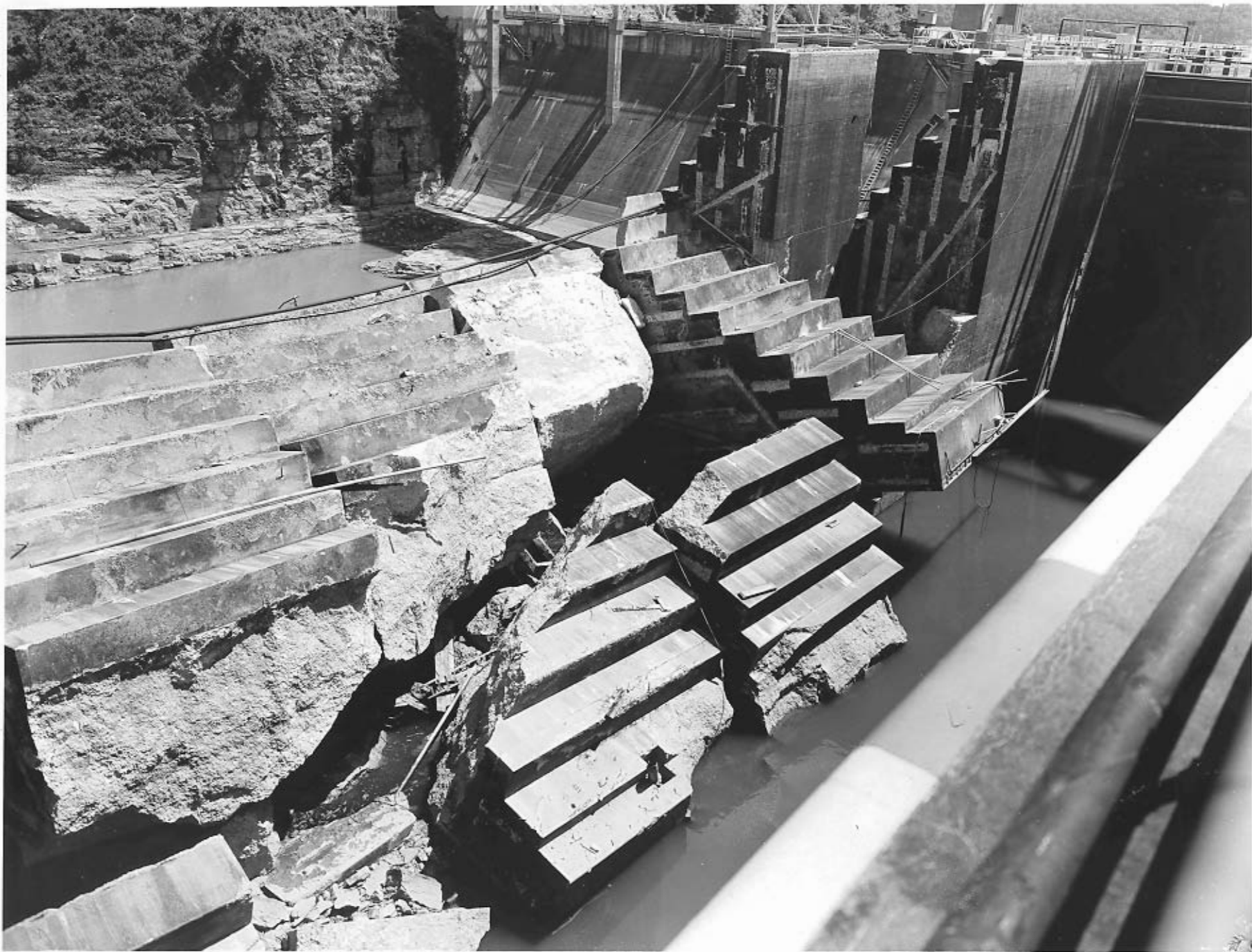
WHEELER LOCK Tennessee Valley Authority 3L1082 June 14, 1961 C. Quillen, Wilson Dam
