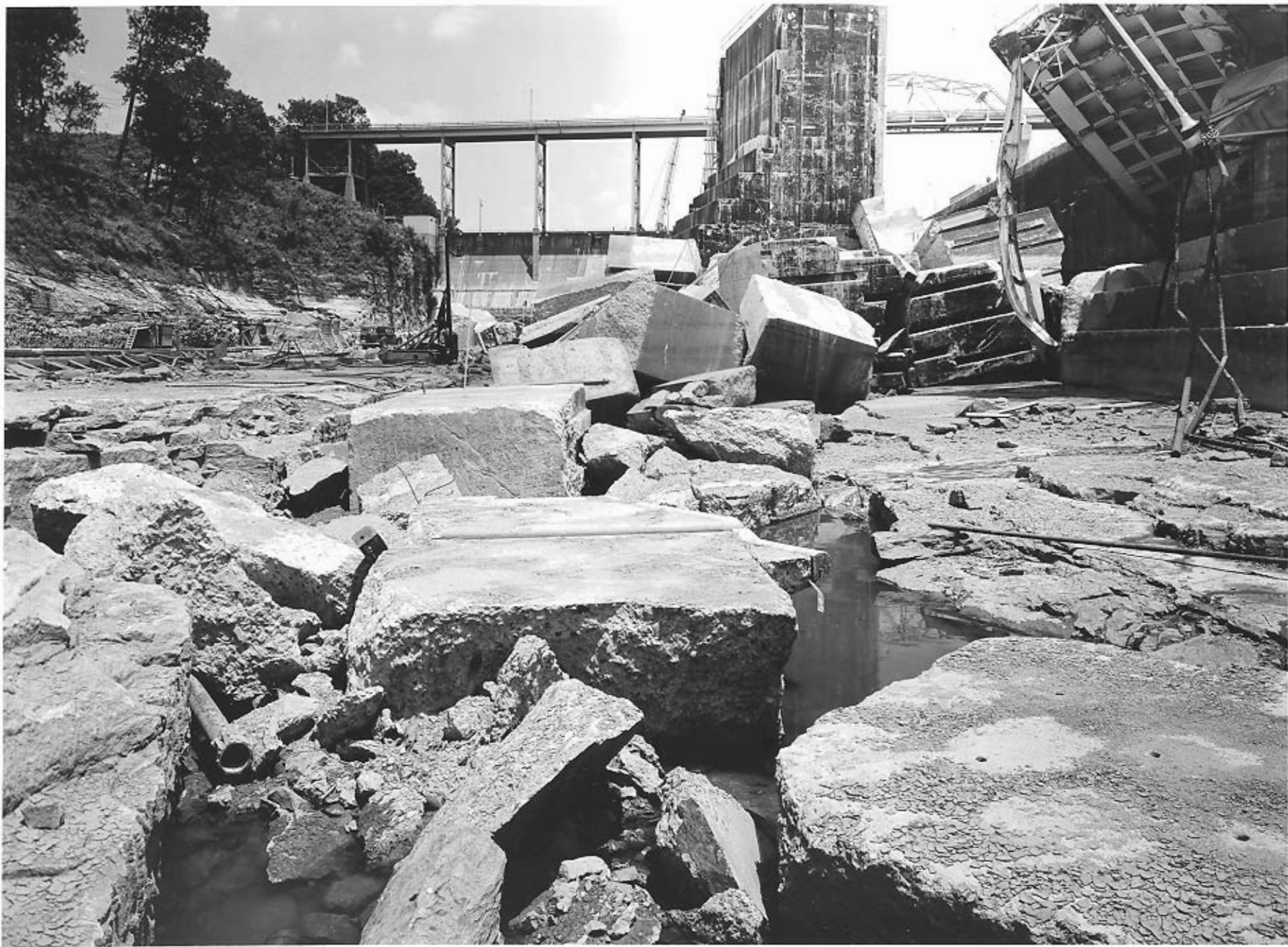
WHEELER LOCK Tennessee Valley Authority 3L1129 June 28, 1961 C. Quillen, Wilson Dam
