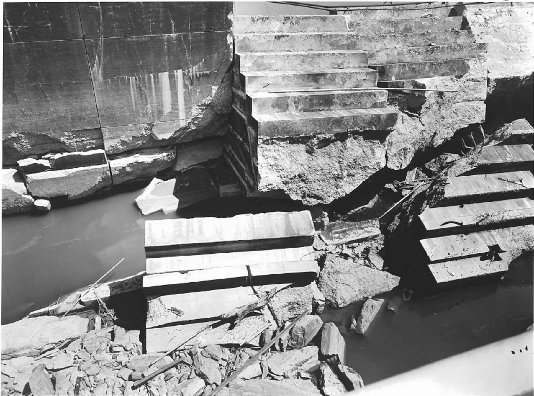
WHEELER LOCK Tennessee Valley Authority 3L1081 June 14, 1961 C. Quillen, Wilson Dam
