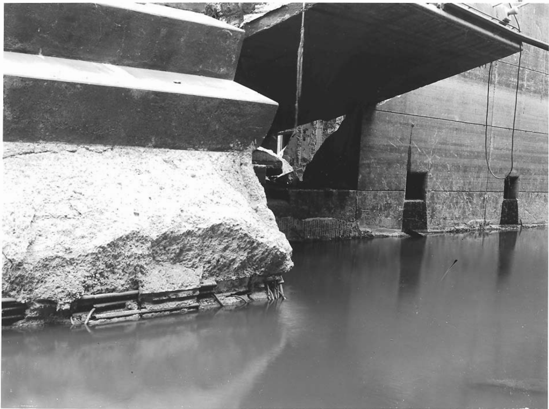
WHEELER LOCK Tennessee Valley Authority 3L1117 June 16, 1961 C. Quillen, Wilson Dam
