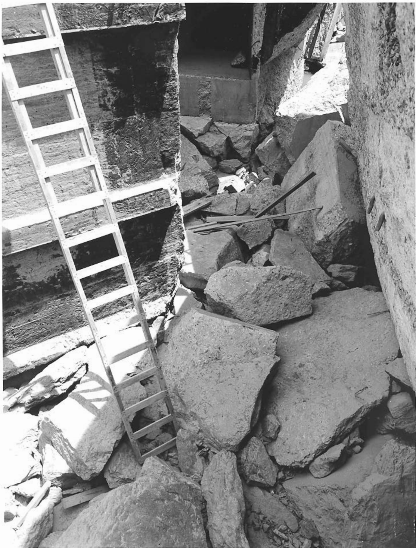
WHEELER LOCK Tennessee Valley Authority 311141 July 5, 1961 C. Quillen, Wilson Dam
