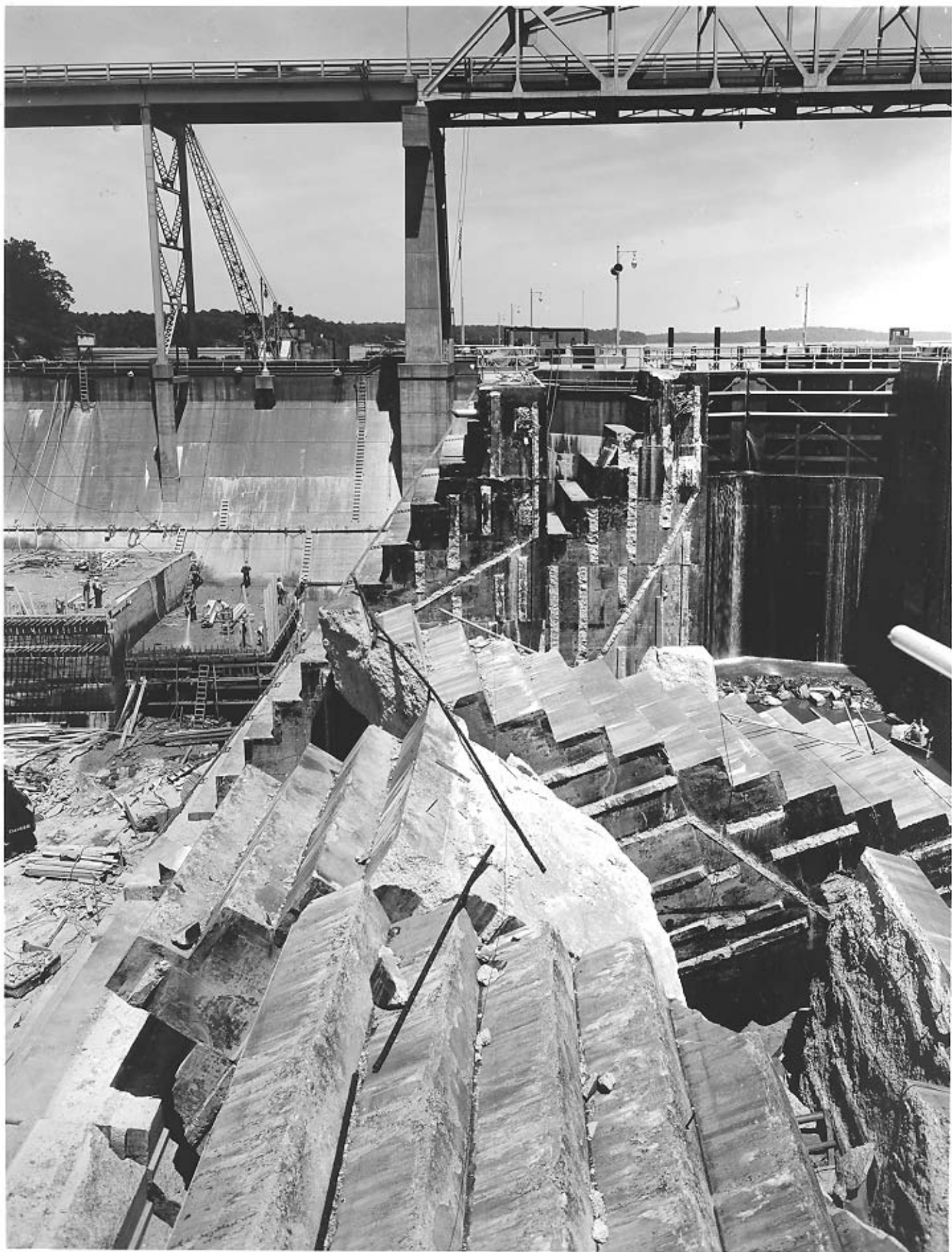
Auxiliary lock, looking upstream from top of block 7.
