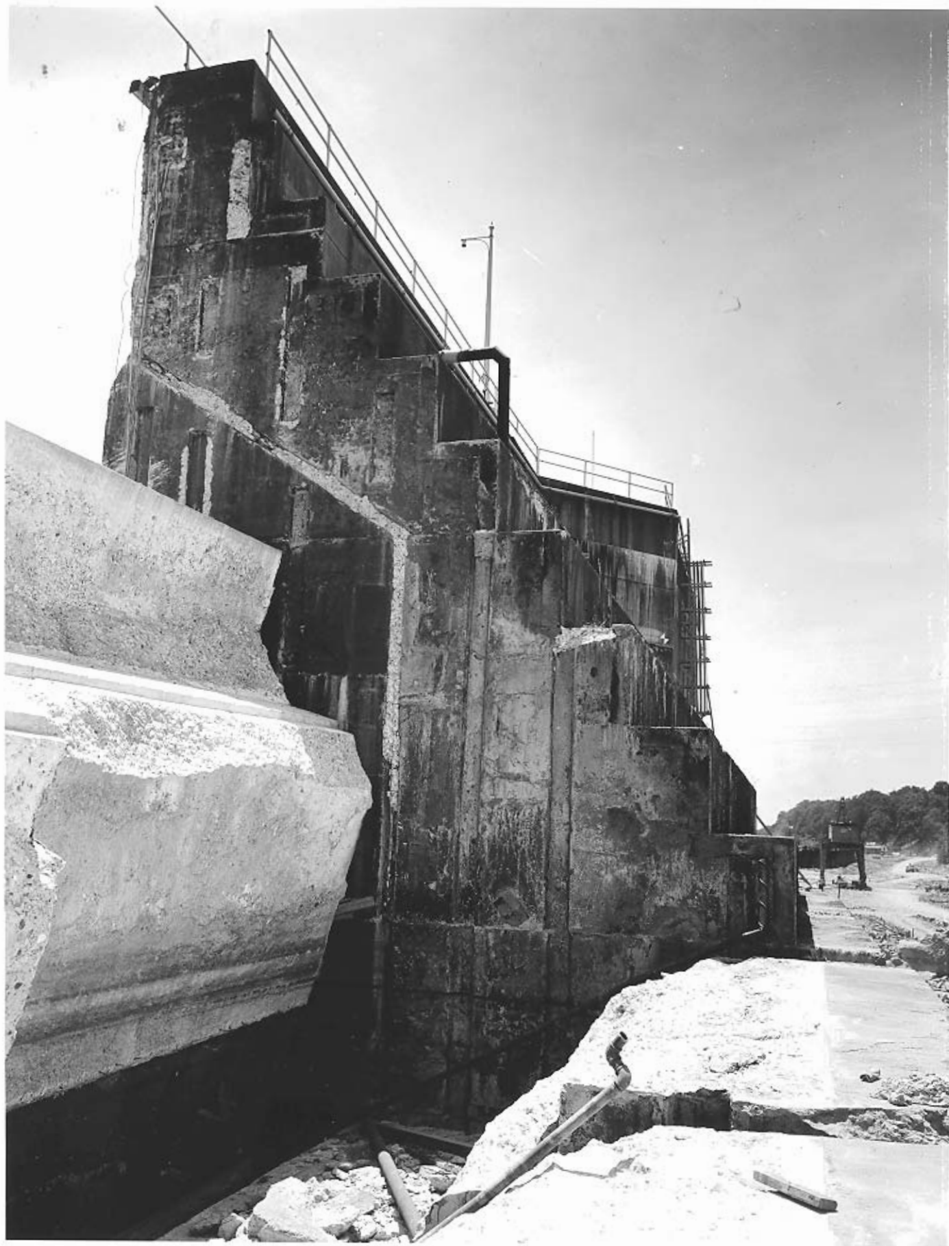
Auxiliary lock, upstream face of block 7.
