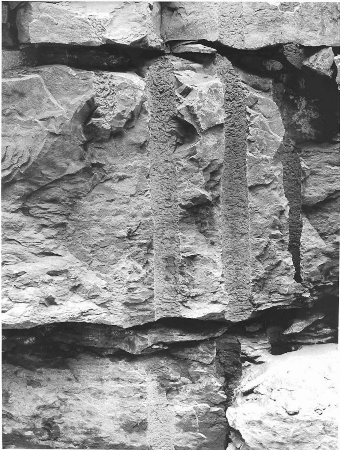
WHEELER LOCK Tennessee Valley Authority 3L1099 June 15, 1961 C. Quillen, Wilson Dam
