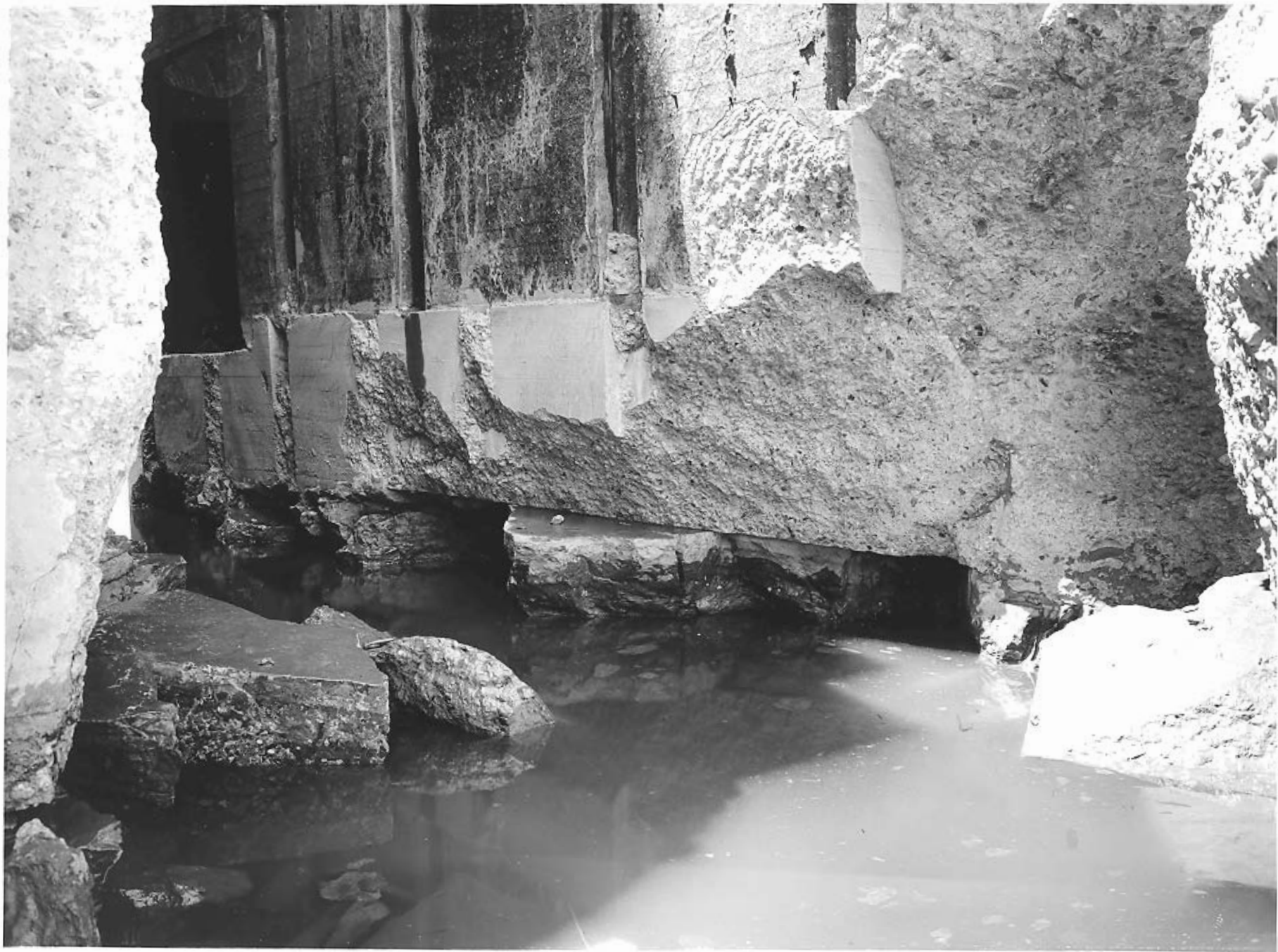
WHEELER LOCK Tennessee Valley Authority 3L1105 June 15, 1961 C. Quillen, Wilson Dam
