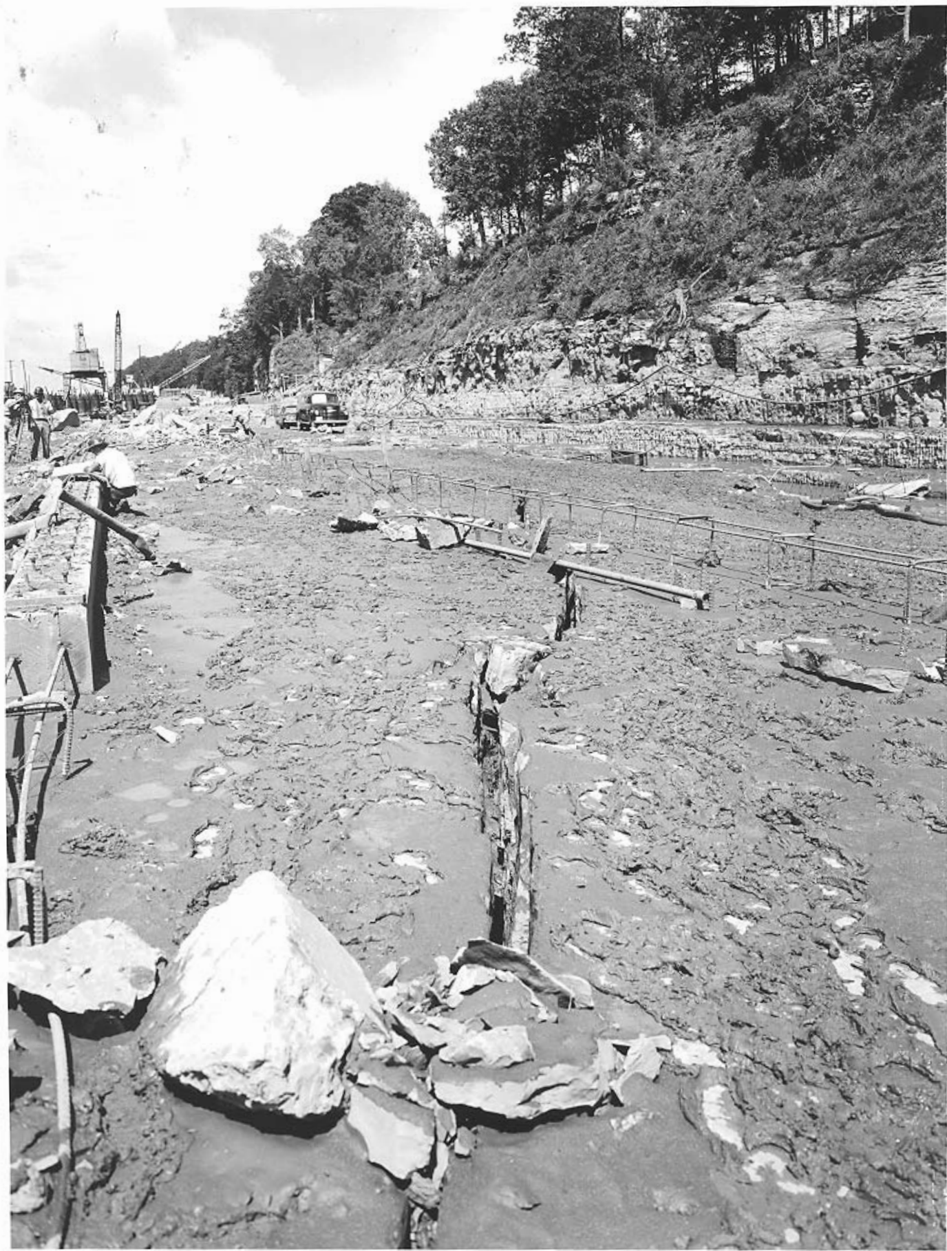
Looking downstream at crack in rock.
