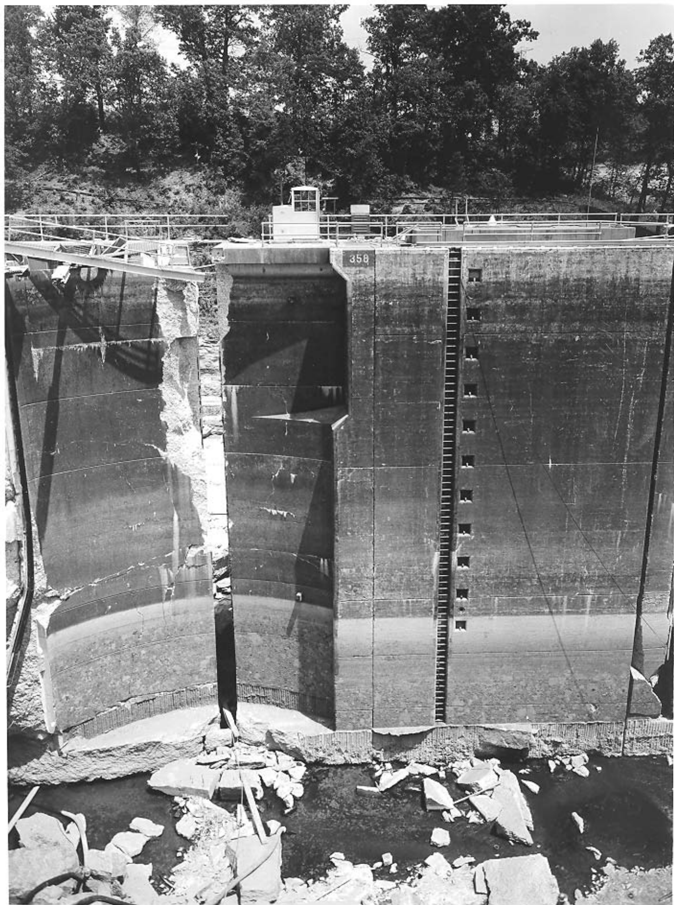
WHEELER LOCK Tennessee Valley Authority 311152 July 6, 1961 C. Grillen, Wilson Dam
