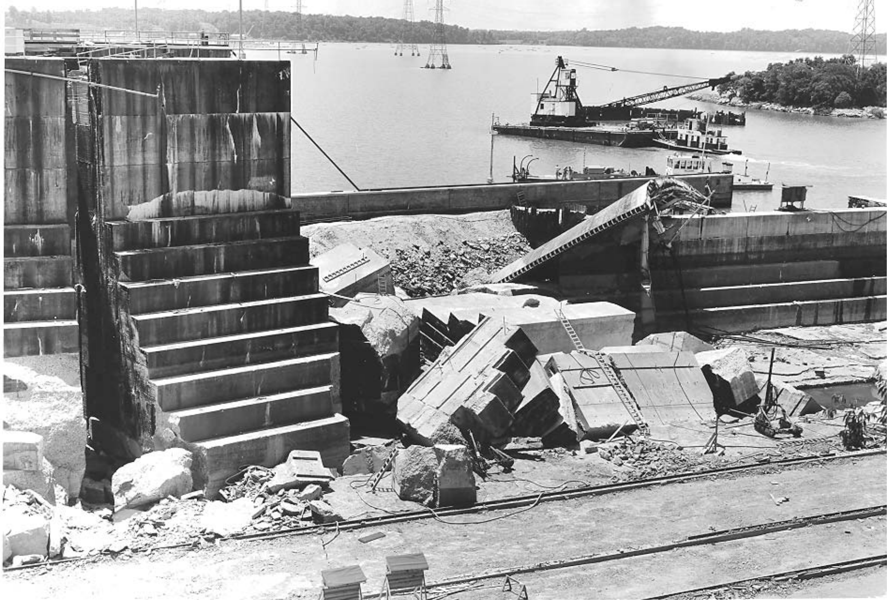
WHEELER LOCK Tennessee Valley Authority 3L1127 June 28, 1961 C. Quillen, Wilson Dam
