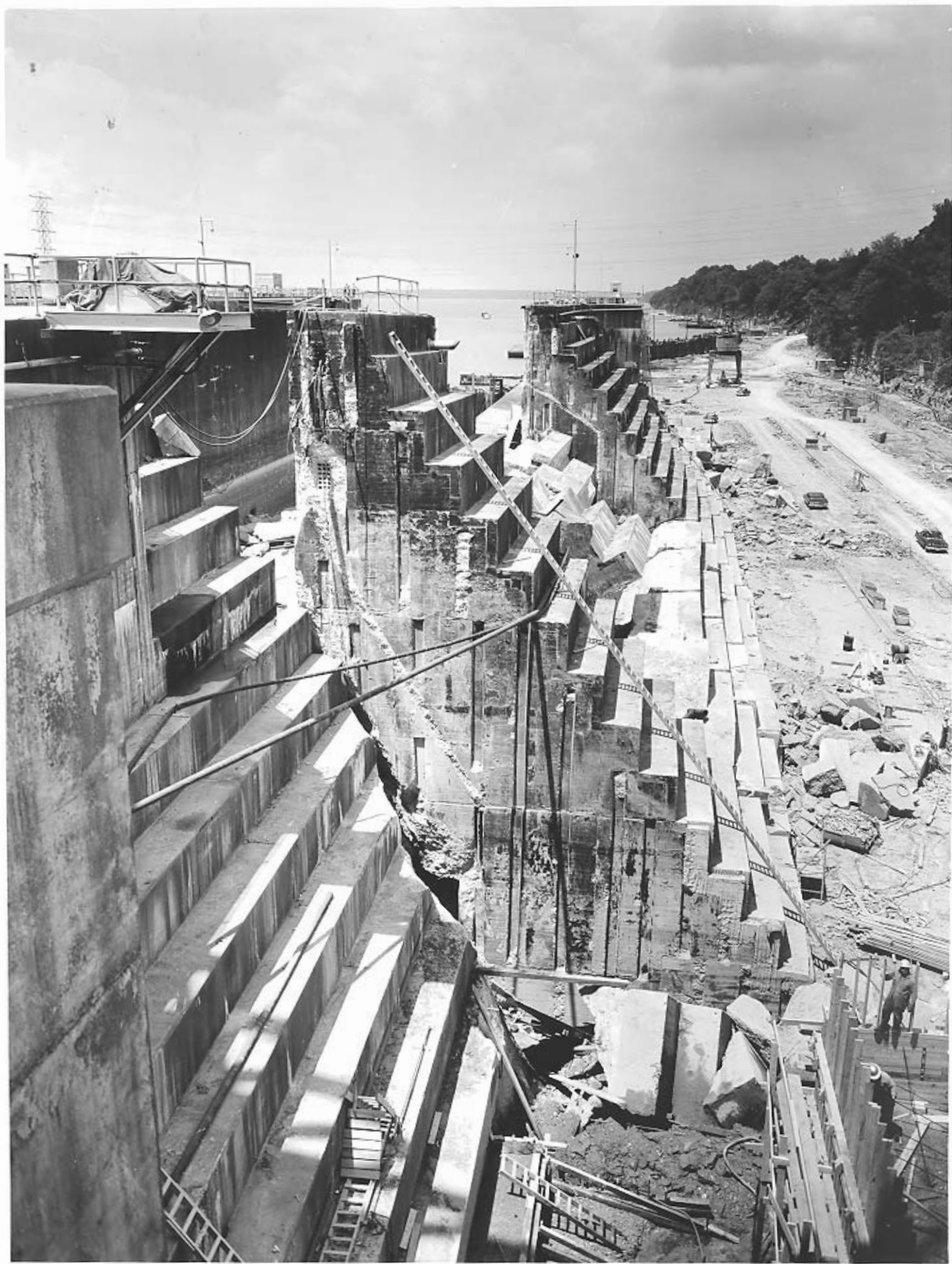
Auxiliary lock, looking downstream from dam non-overflow section.
