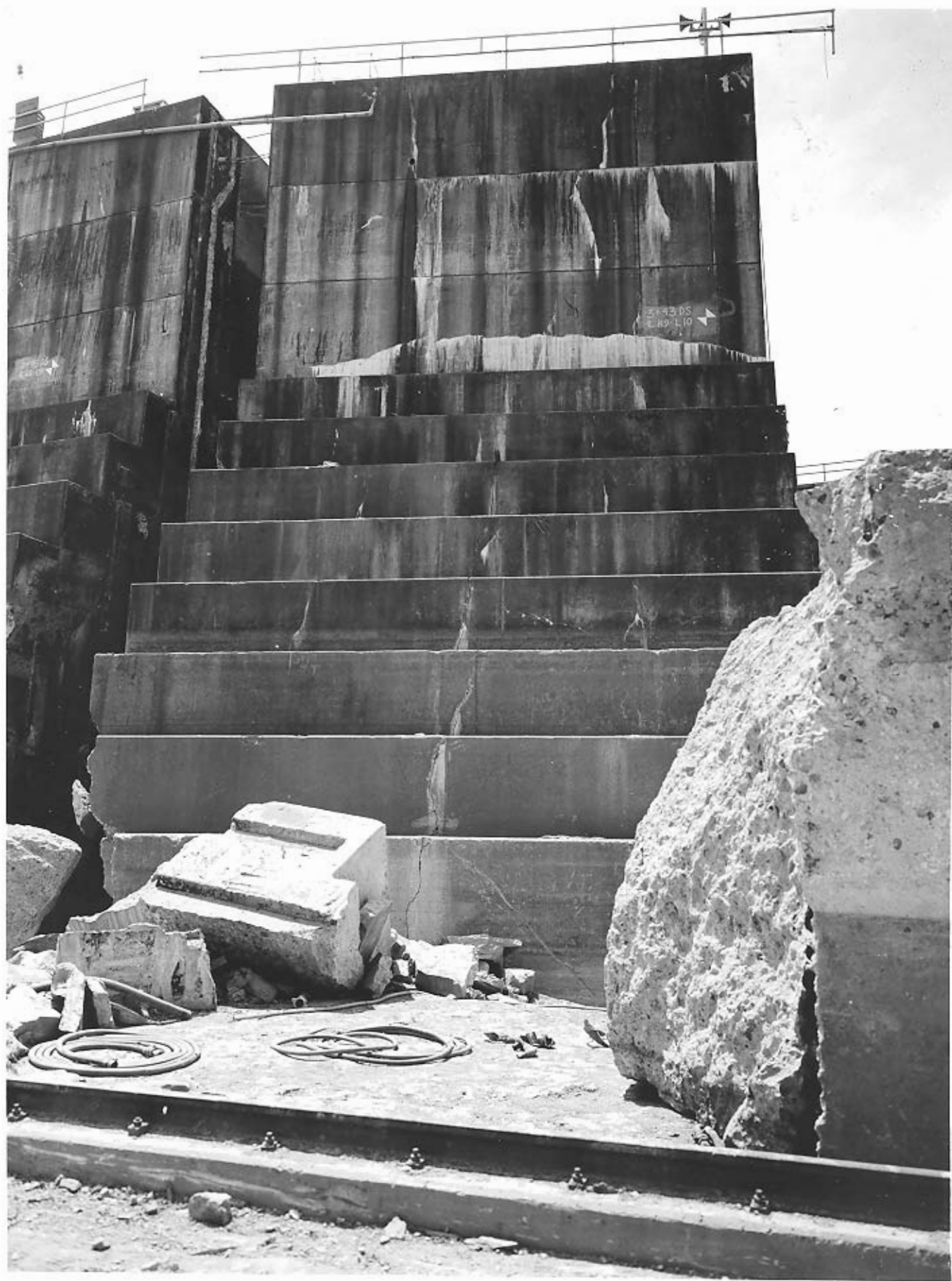
WHEELER LOCK Tennessee Valley Authority 311149 July 5, 1961 C. Quillen, Wilson Dam
