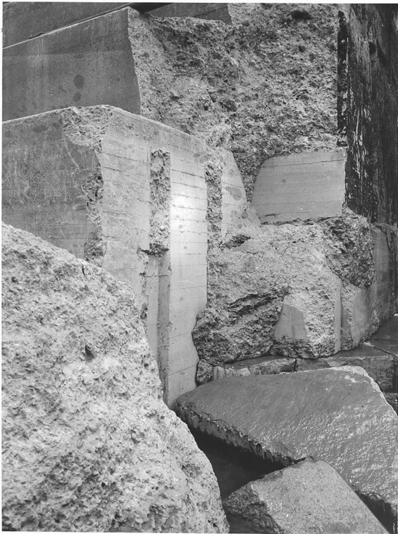
WHEELER LOCK Tennessee Valley Authority 311106 June 15, 1961 C. Quillen, Wilson Dam
