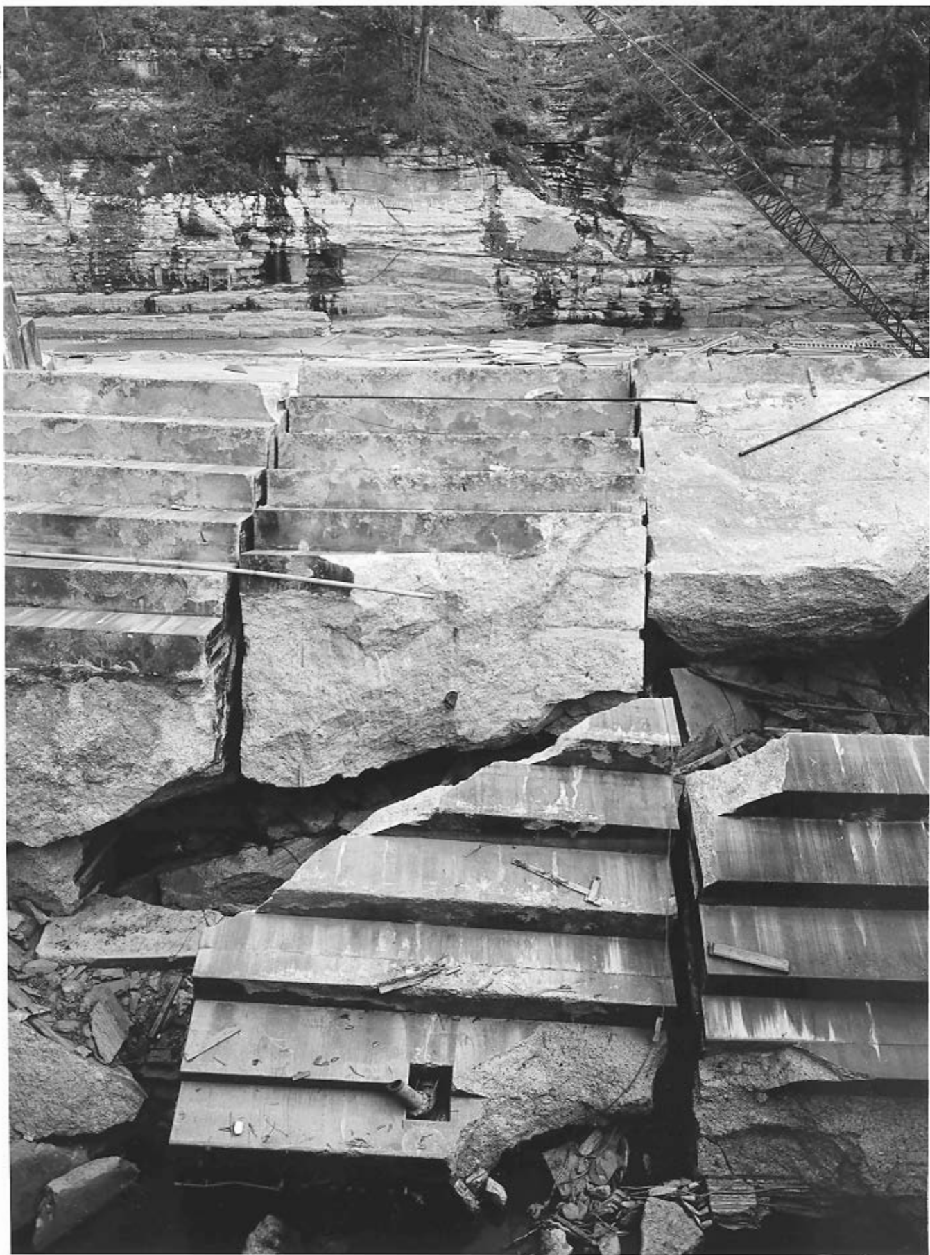
WHEELER LOCK Tennessee Valley Authority 311158 July 6, 1961 C. Quillen, Wilson Dam
