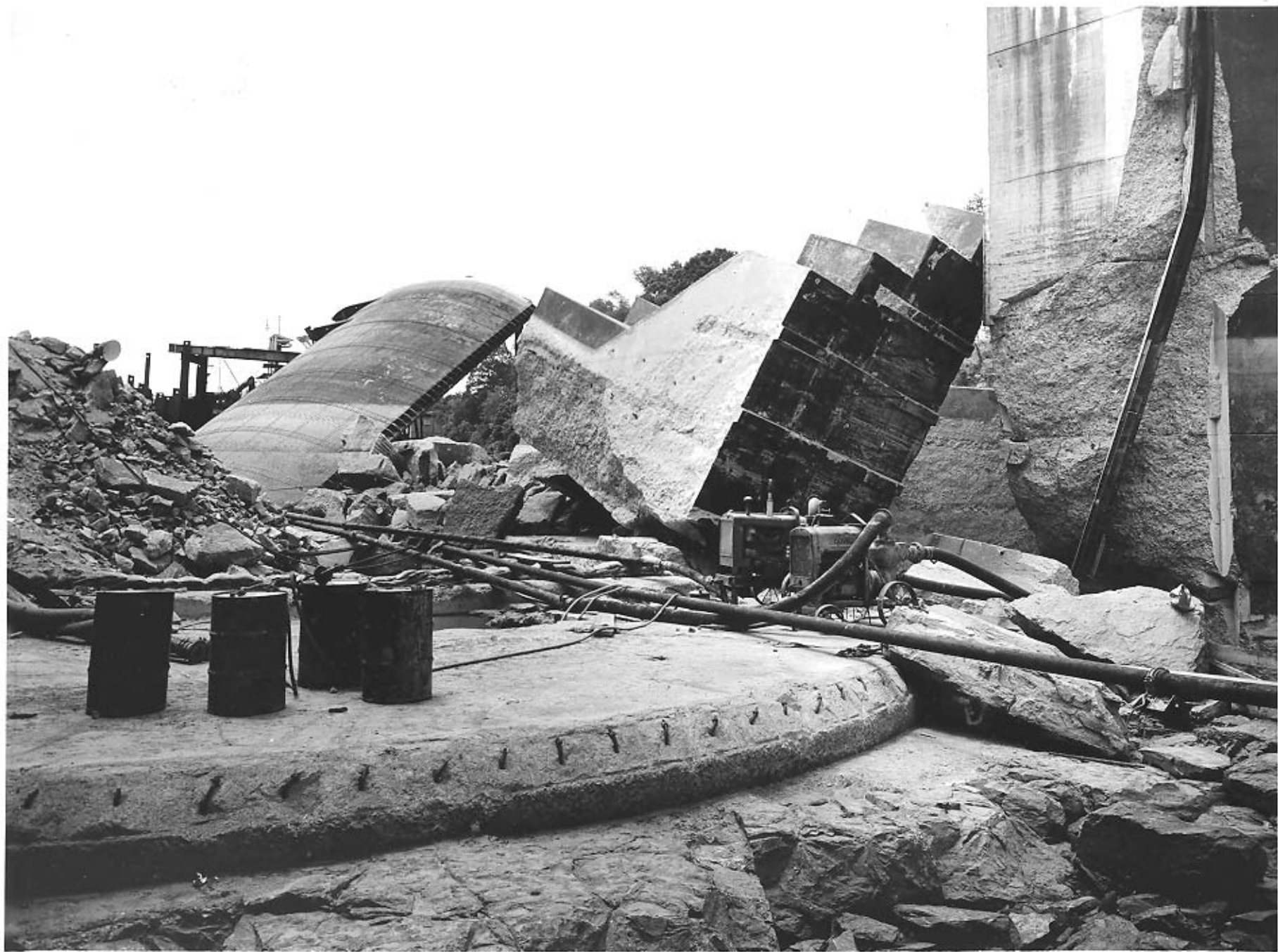
WHEELER LOCK Tennessee Valley Authority 3L1131 June 28, 1961 C. Quillen, Wilson Dam
