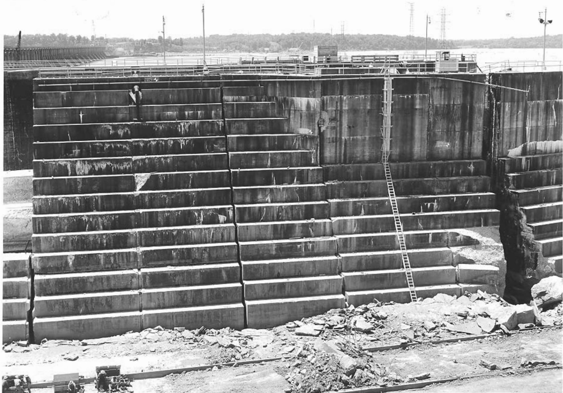
WHEELER LOCK Tennessee Valley Authority 3L1126 June 28, 1961 C. Quillen, Wilson Dam
