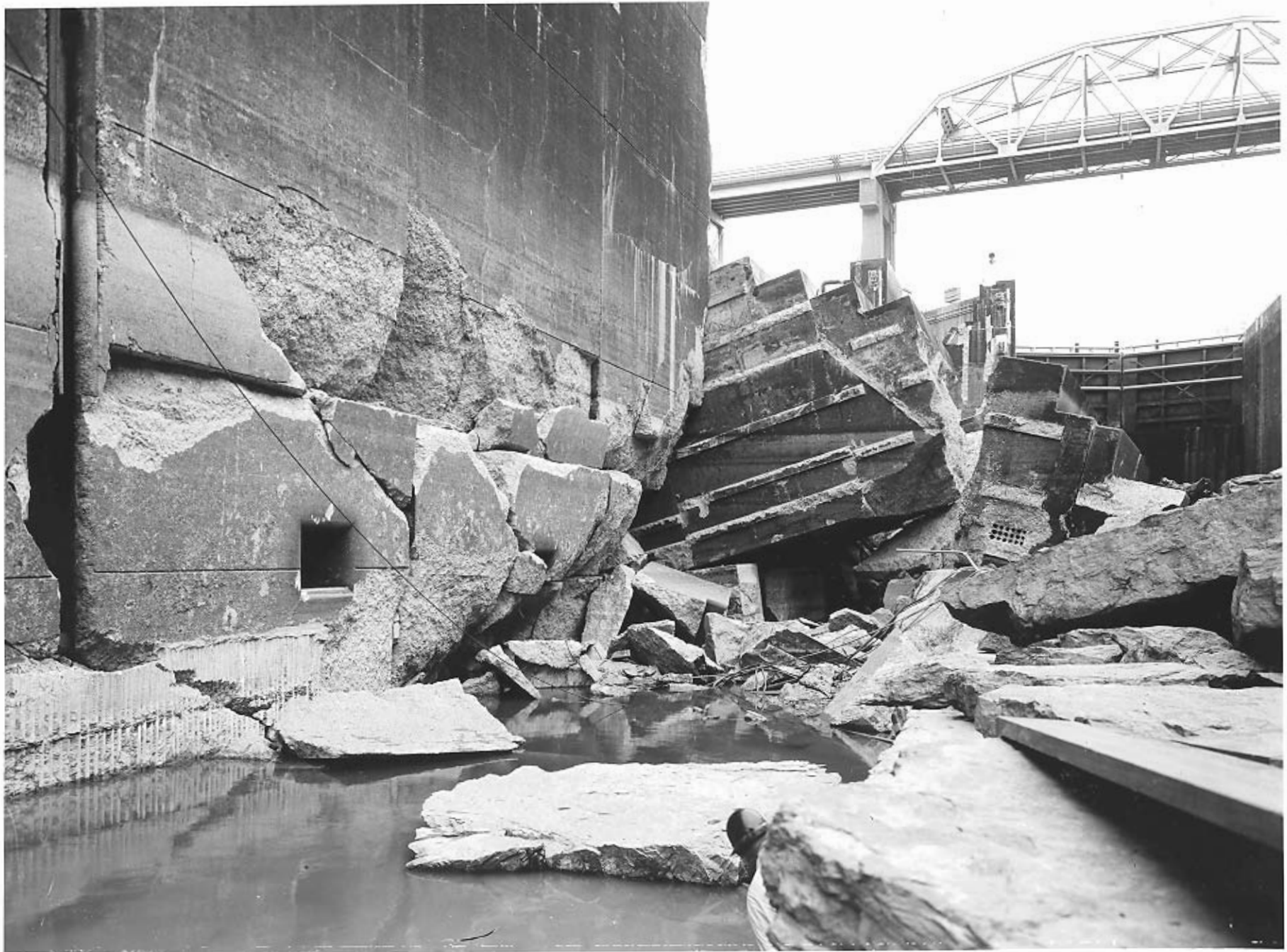
WHEELER LOCK Tennessee Valley Authority 3L1115 June 16, 1961 C. Quillen, Wilson Dam
