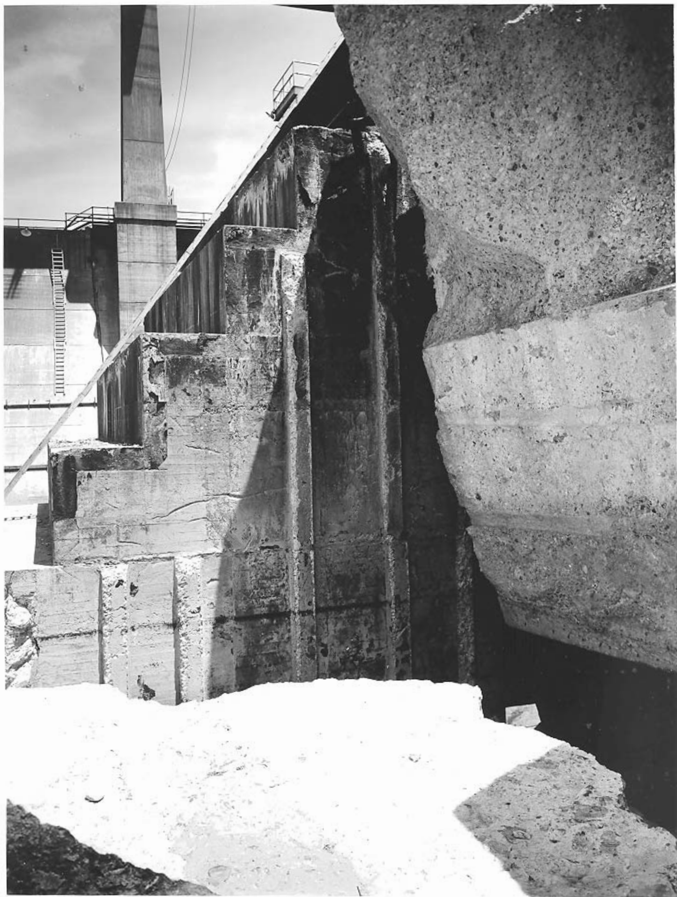
Auxiliary lock, portion of downstream face of block 2.
