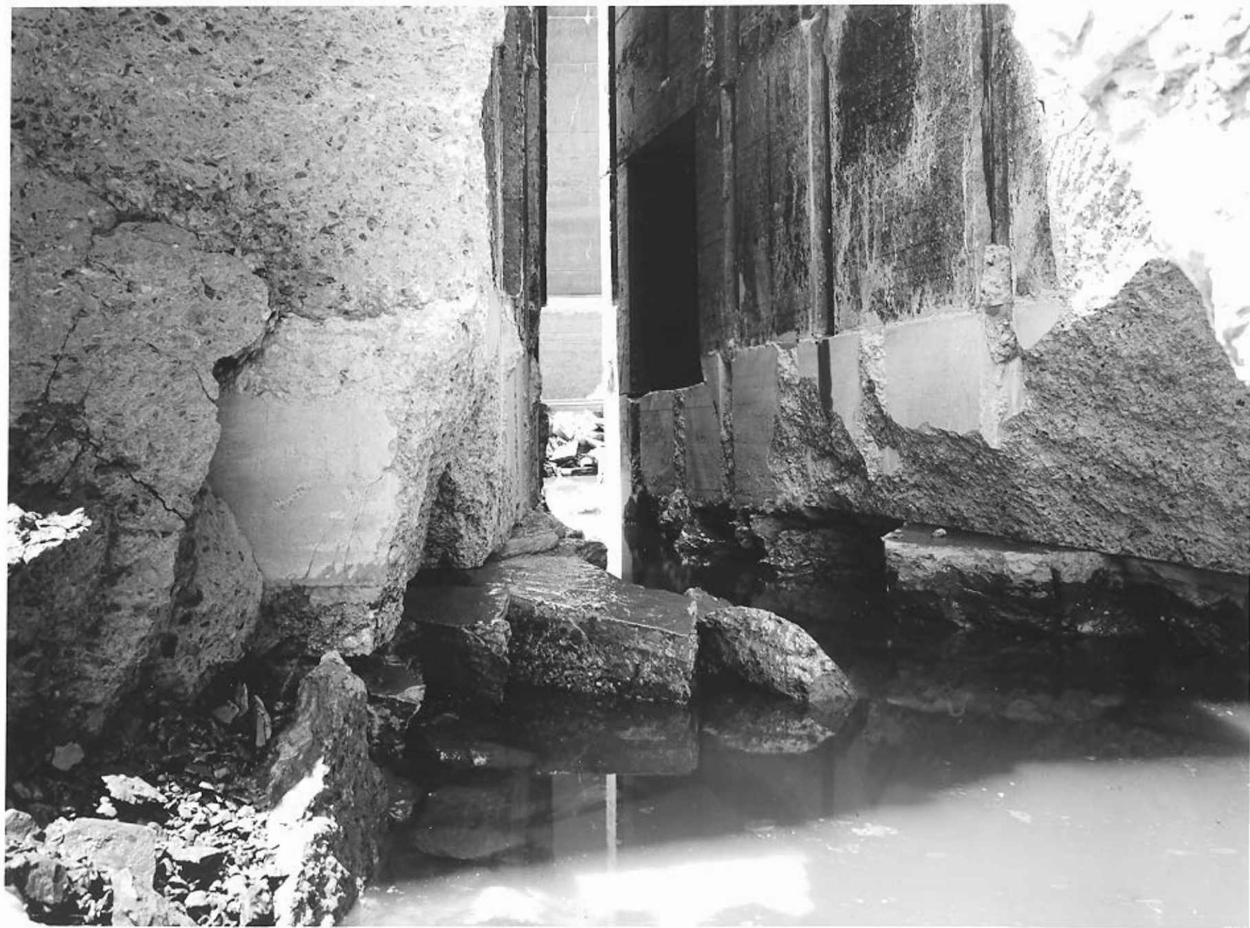
WHEELER LOCK Tennessee Valley Authority 3L1104 June 15, 1961 C. Quillen, Wilson Dam
