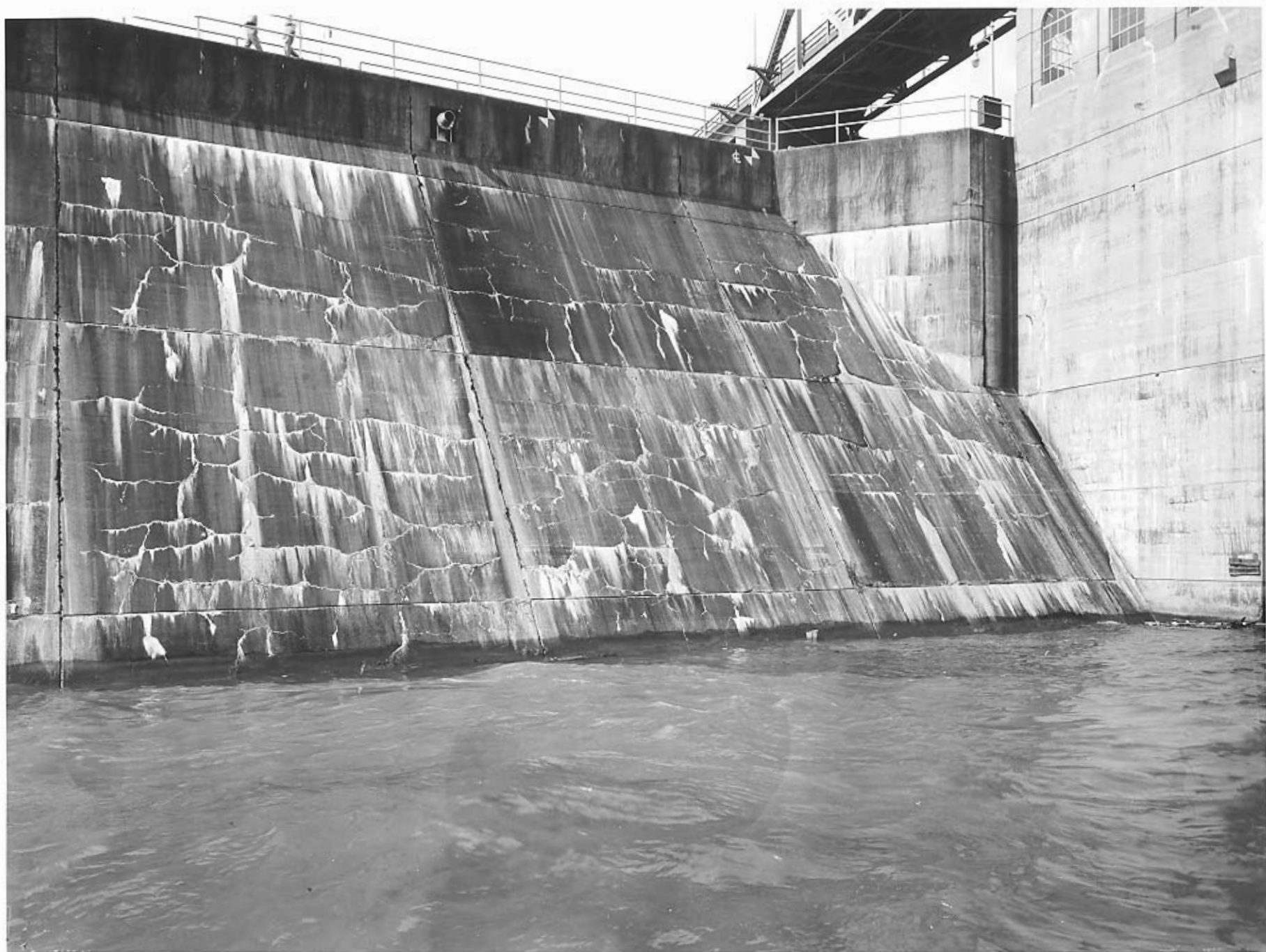
WHEELER LOCK Tennessee Valley Authority 3L1091 June 15, 1961 C. Quillen, Wilson Dam
