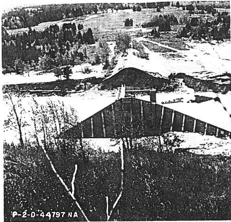
Photograph No. 1 Two Medicine Dam - View from left abutment. 6-11-64
