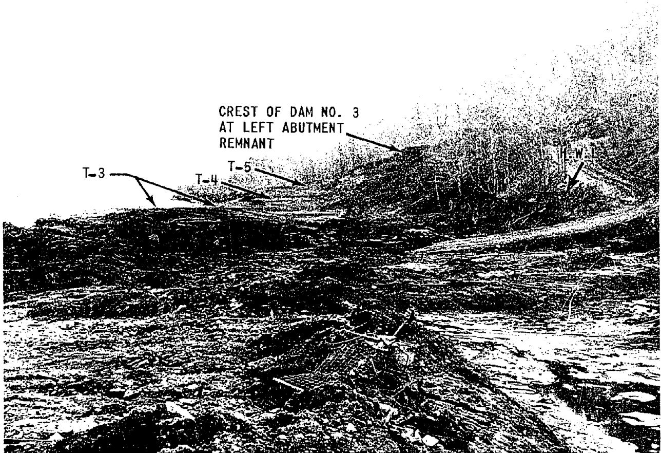
LEFT SIDE OF MIDDLE FORK VALLEY, LOOKING UPSTREAM FROM THE UPPER END OF THE REFUSE BANK. NOTE POOL 2 SLUDGE COVERING THE ROAD TO DAM NO. 3. PHOTO TAKEN FEBRUARY 29, 1972. THE THREE HIGHEST STREAM TERRACES CARVED IN DAM NO. 3 BY THE FLOODWATERS ARE INDICATED BY T-3, T-4, AND T-5. H.W.L. = HIGH WATER LINE FROM FLOOD
