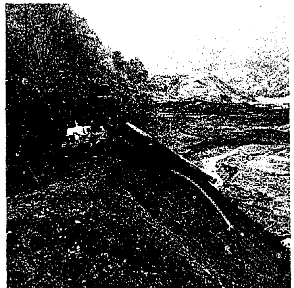
PHOTO D. UPSTREAM PIPE JUST AFTER PULLING IT TO THE EXPLORATORY BULLDOZER TRENCH ON THE LEFT ABUTMENT OF DAM NO. 3.
