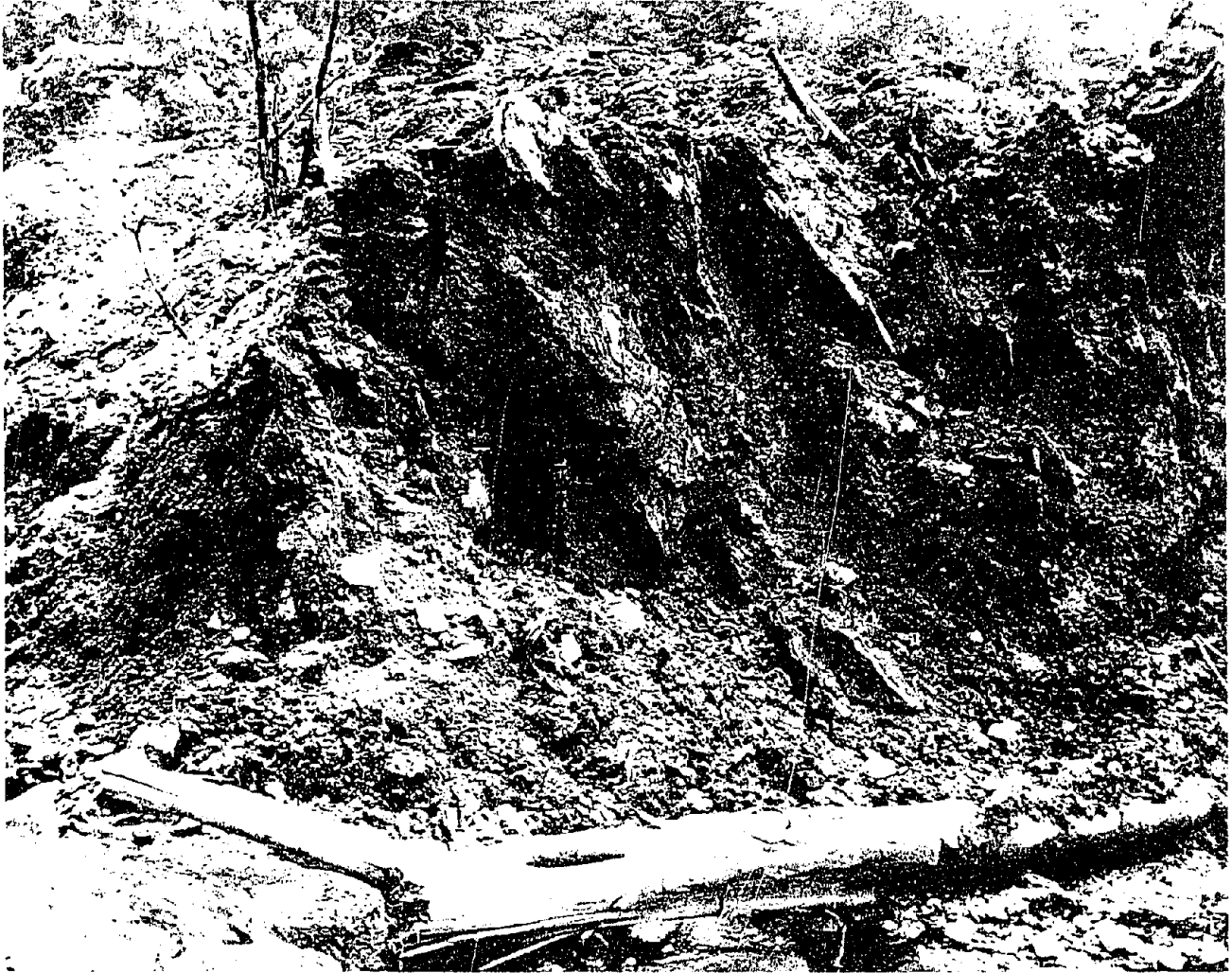
STEEPLY DIPPING CONTACT OF POOL 2 SLUDGE AND DAM NO. 3 EMBANKMENT GRAVELS AREA IS AT THE 82° DIP SYMBOL UPSTREAM FROM THE DAM NO. 2 BREACH ON FIGURE VI-20.
