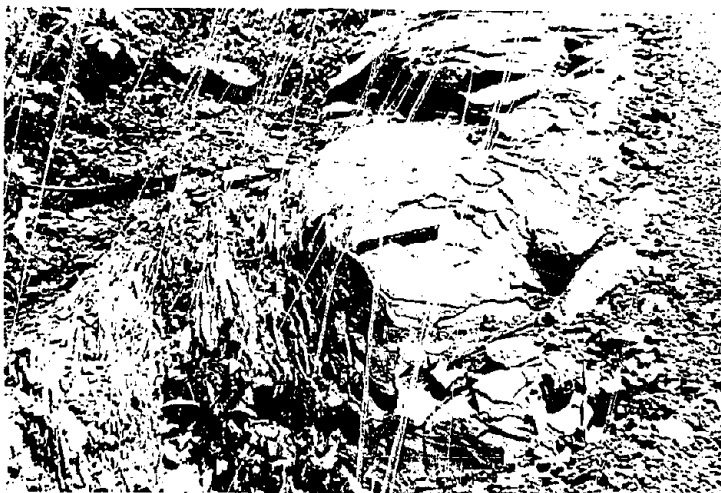
PHOTO B. SHALE ALONG NO. 5 MINE ROAD ABOVE POOL 2. THE FOLDING RULE LIES ON A BEDDING PLANE. LEFT OF THE RULE IS AN AREA OF VERY CLOSELY SPACED NEAR-VERTICAL JOINTS.
