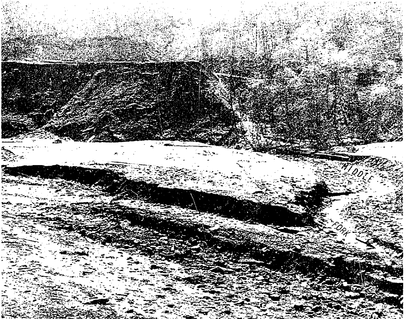
DOWNSTREAM PORTION OF LEFT ABUTMENT REMNANT OF DAM NO. 3, FEBRUARY 29, 1972. THE LOW, SCoured MOUND IN THE CENTER EXTENDED TO THE RIGHT DURING THE FIRST STAGES OF THE FAILURE. IN THE FINAL EMPTYING OF POOL 3, THE MOUND WAS DISSECTED BY MIDDLE FORK AS SEEN HERE.
