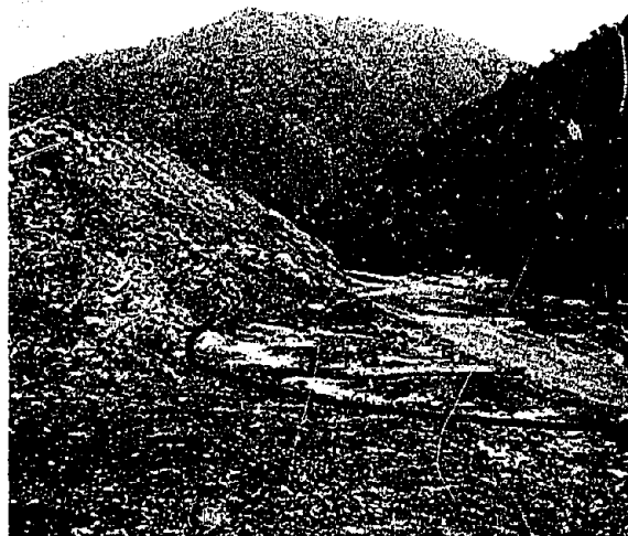
PHOTO C. INCIPIENT STREAM TERRACE DEVELOPED ON REFUSE BANK BY FLOOD WATER, NEAR HIGHEST POOL 2 SLUDGE (FIGURE VI-4). AREA IN FRONT OF LINE IS THE SAME TERRACE, BUT IS COVERED WITH A LAYER OF POST-FLOOD FILL.
