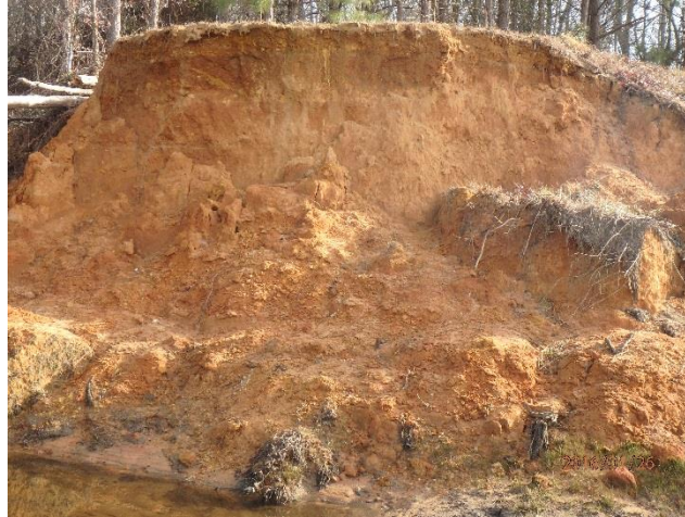
Figure 25: Typical Soil Profile of Failed Dam. Able/Corbett Pond Dam shown (Source: FEMA)
