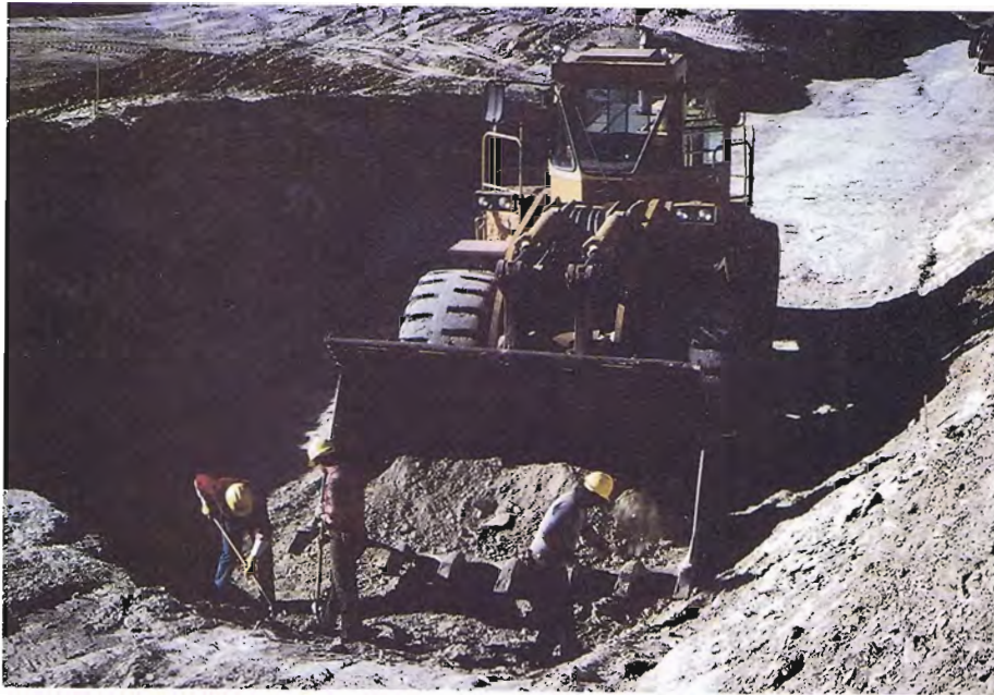
5. Cleaning key trench at about 17 + 50. (1-6-84)
