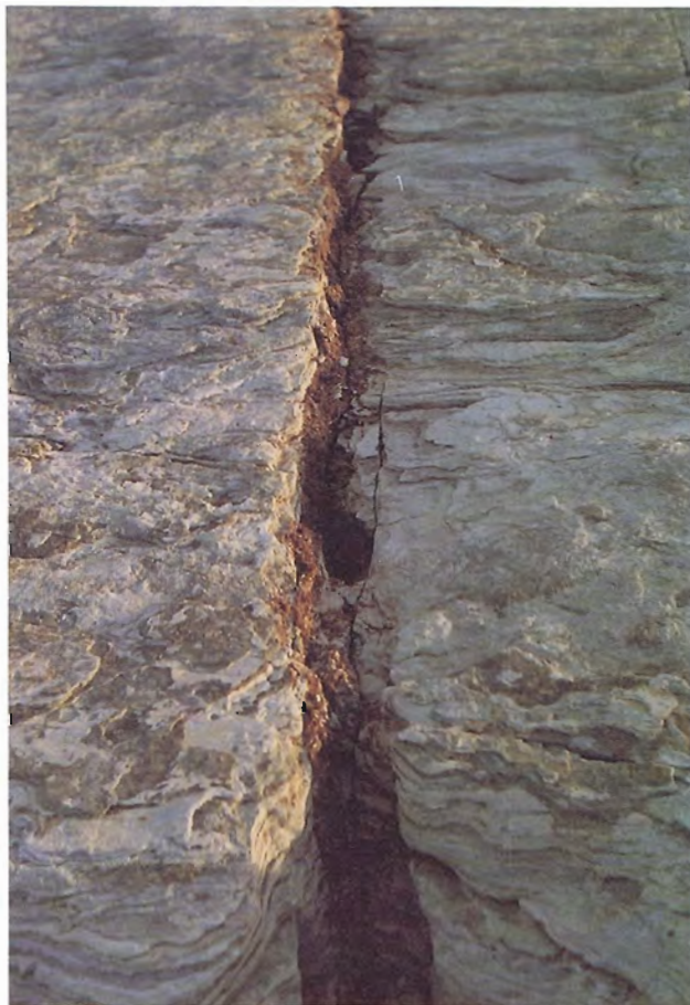
22. Joint with filling downstream of breach.
