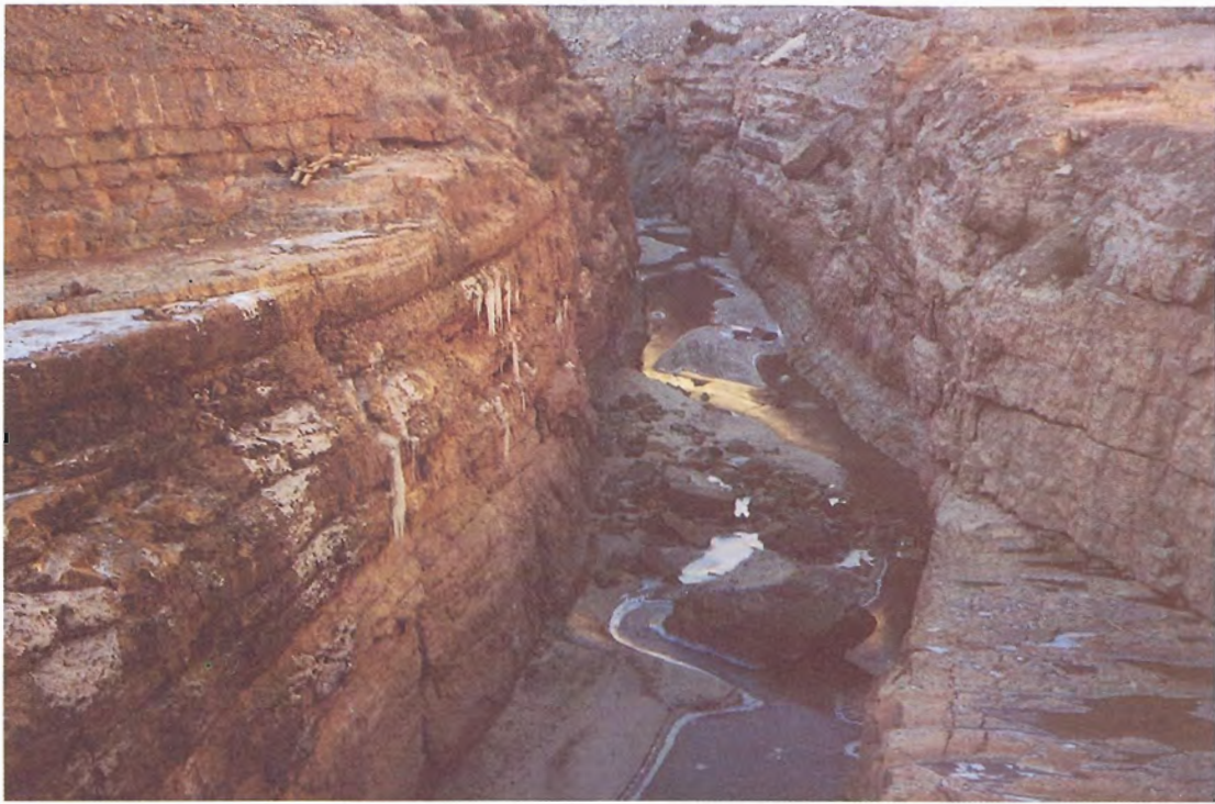
33. Upstream cutoff trench.
