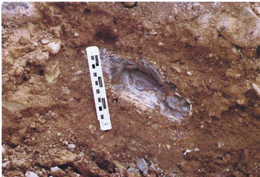
54. Grout plug in Zone I on right side of breach.
