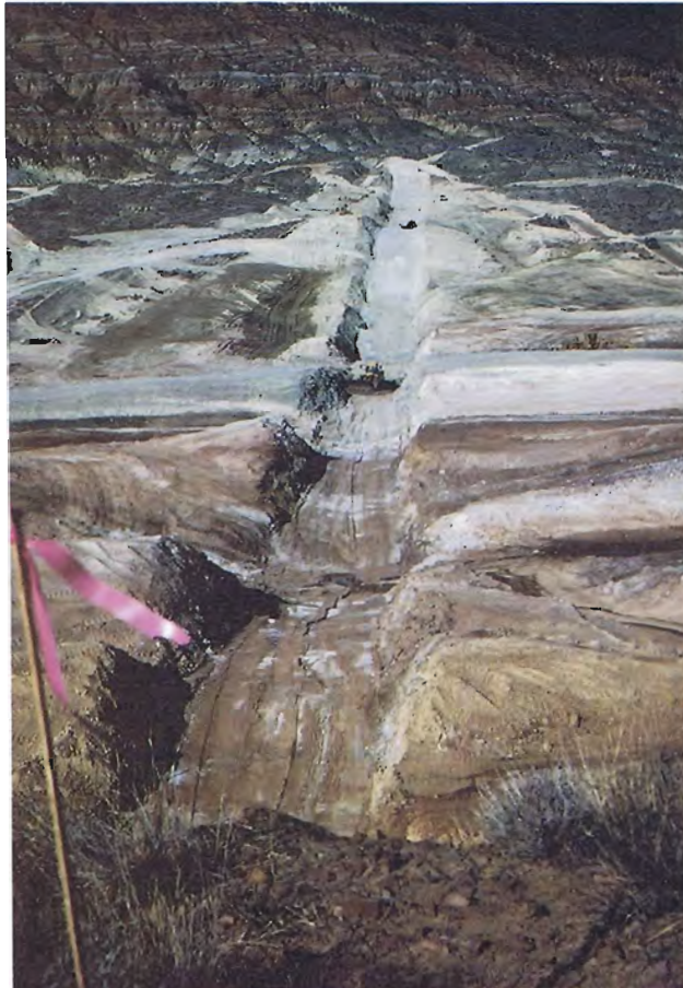
2. View west along key trench from left abutment. (1-6-84)
