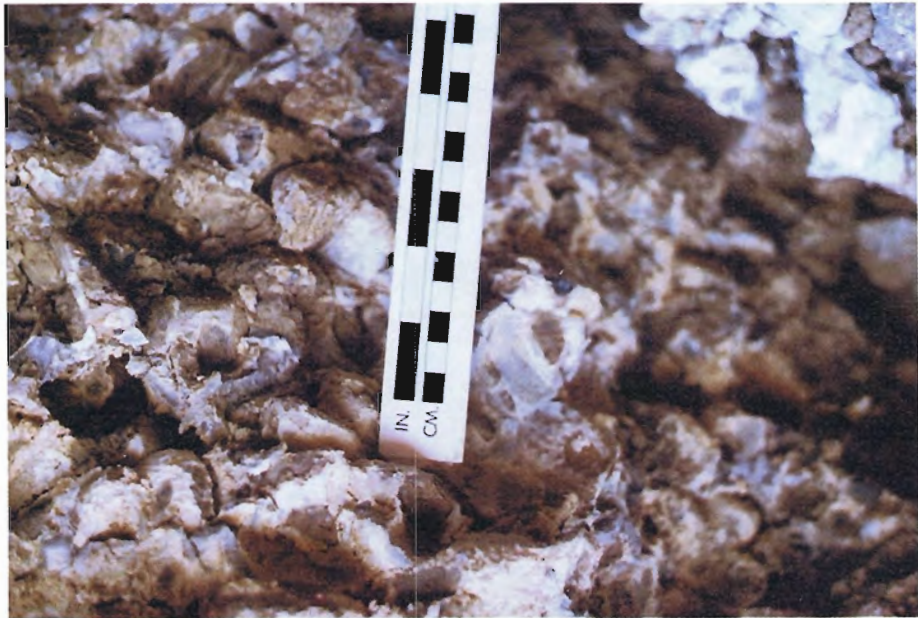
60. Grout-filled toe drains.
