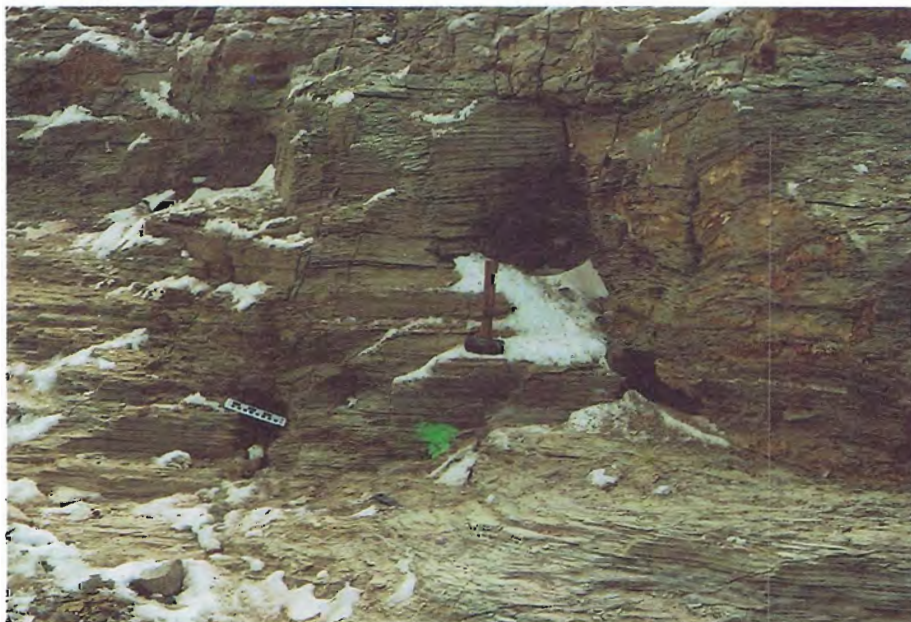
31. View of geologically old solution channels in upstream portion of the breach.
