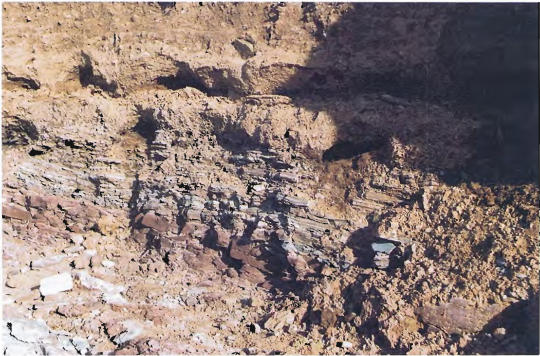
35. Close-up of downstream channels.
