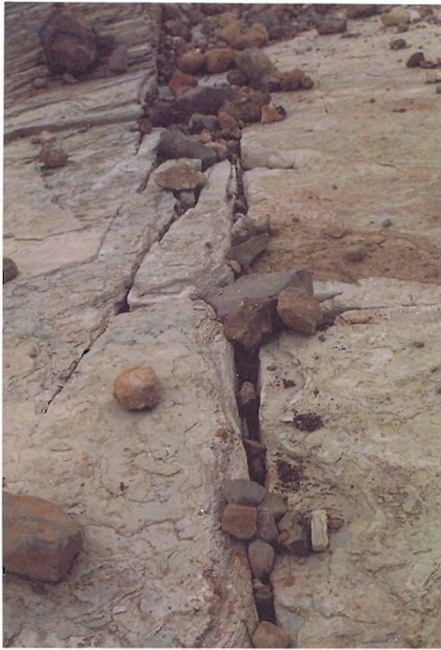
21. Joint exposed in breach section.
