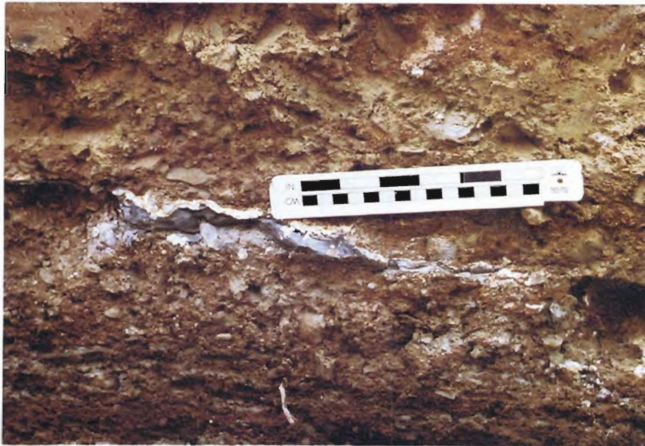
53. Grout intrusion between unit 1 and Zone I fill.
