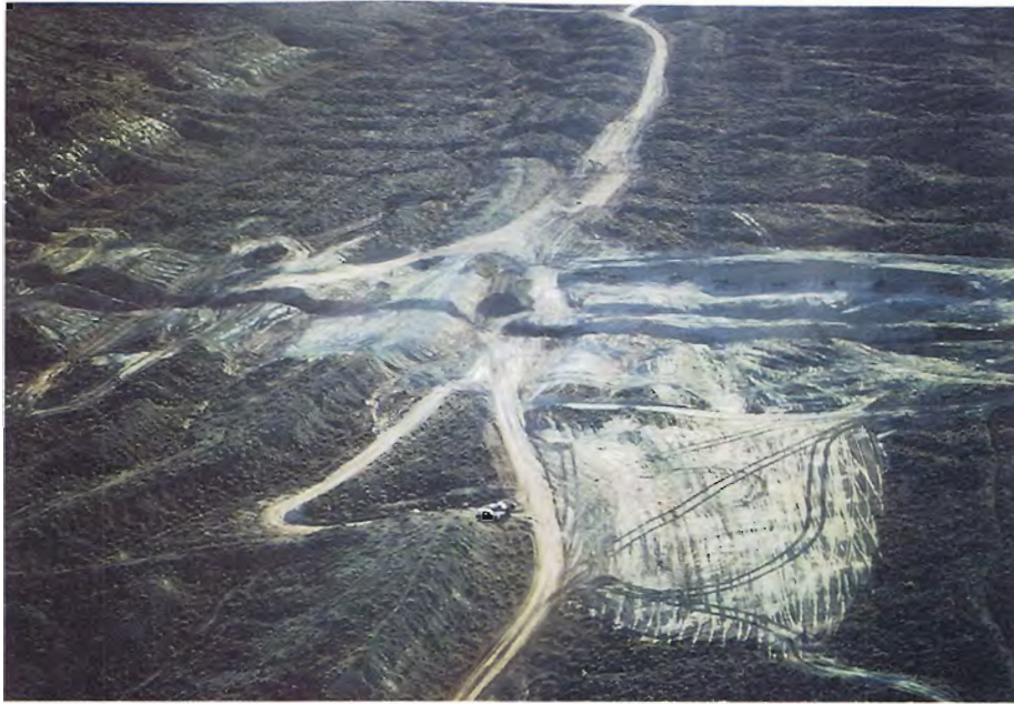
1. Aerial view south showing key trench and footprint of dike. (12-16-83)
