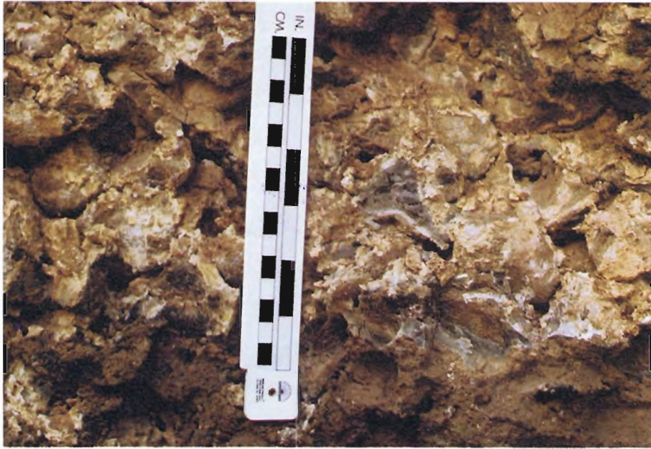
59. Grout-filled toe drains.
