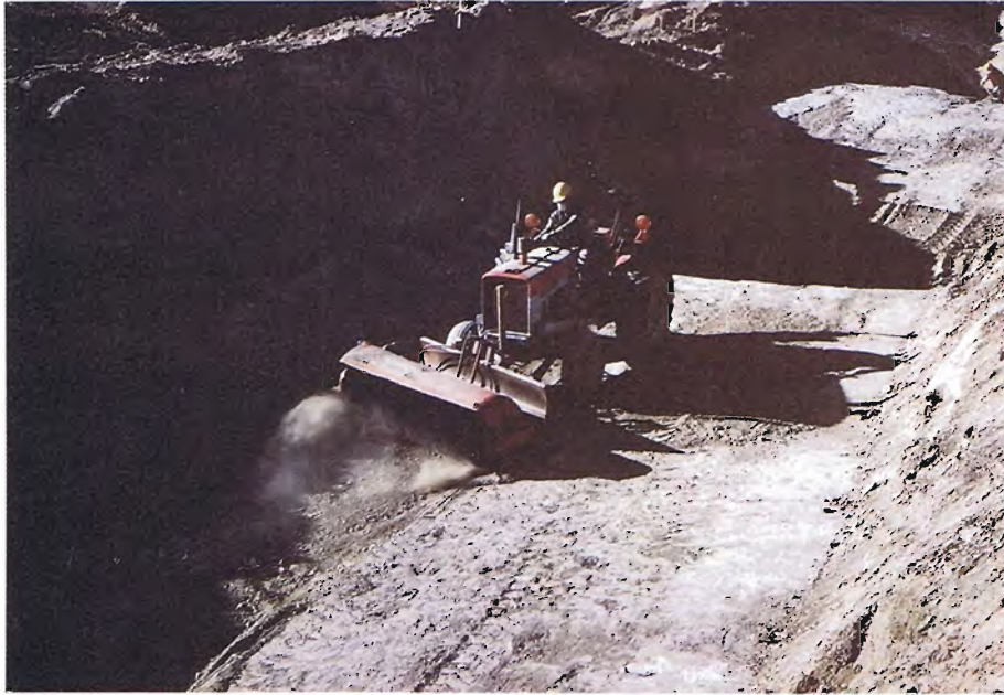
3. Sweeping floor of key trench at 17+00. (1-6-84)
