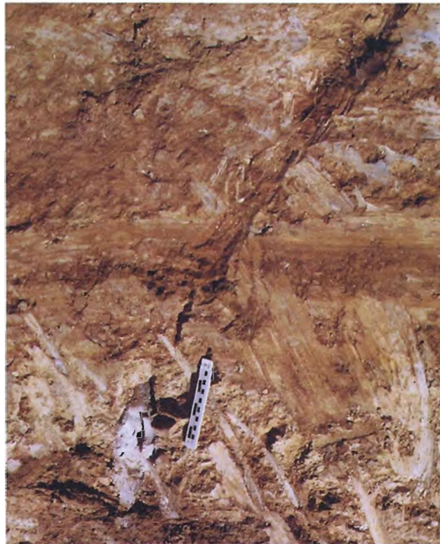
50. Grout contamination in Zone I materials on right side of breach.
