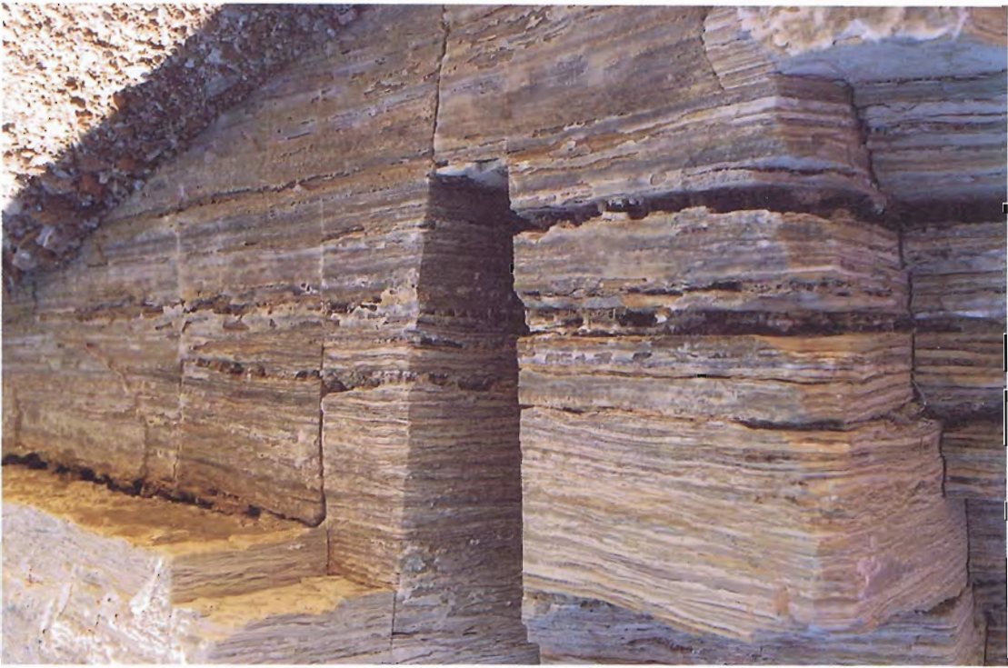
28. View of openings in bedding in breach area.
