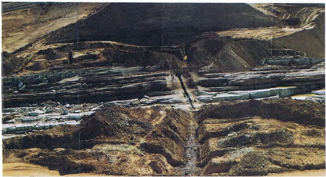
44. View from top of remaining right embankment showing post failure exploratory trenches.
