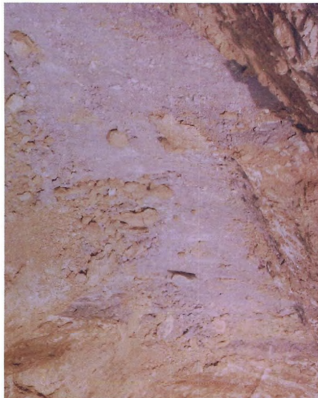
48. Purple clay (Zone II) in bottom of exploratory trench at centerline on left side of breach.
