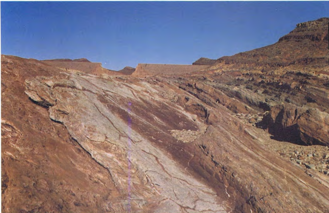
12. Breach from downstream at distance.
