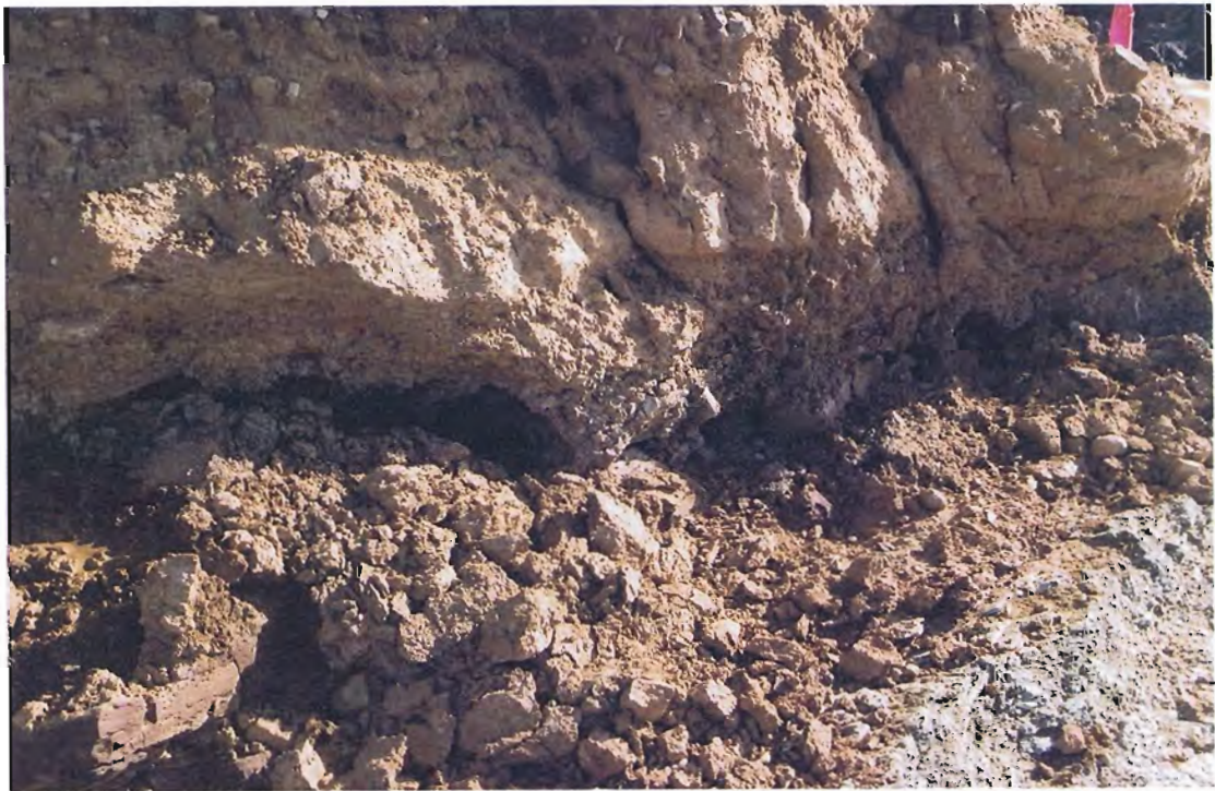
36. Close-up of downstream channels.
