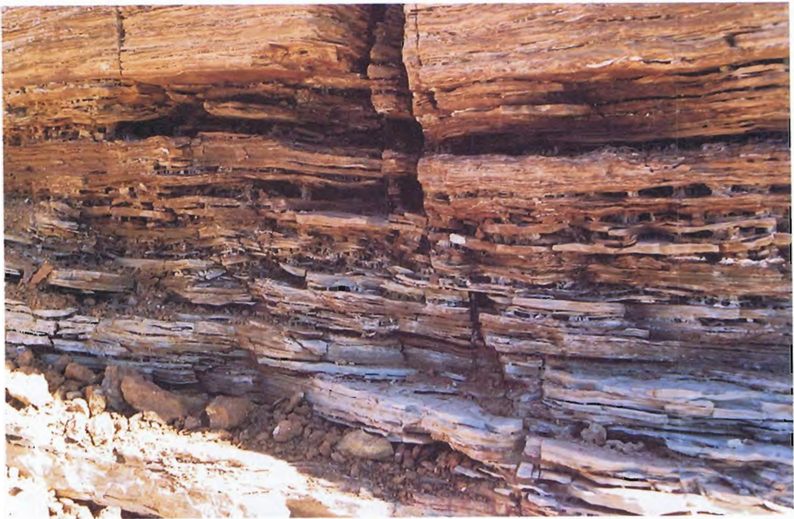
27. View of openings in bedding in breach area.
