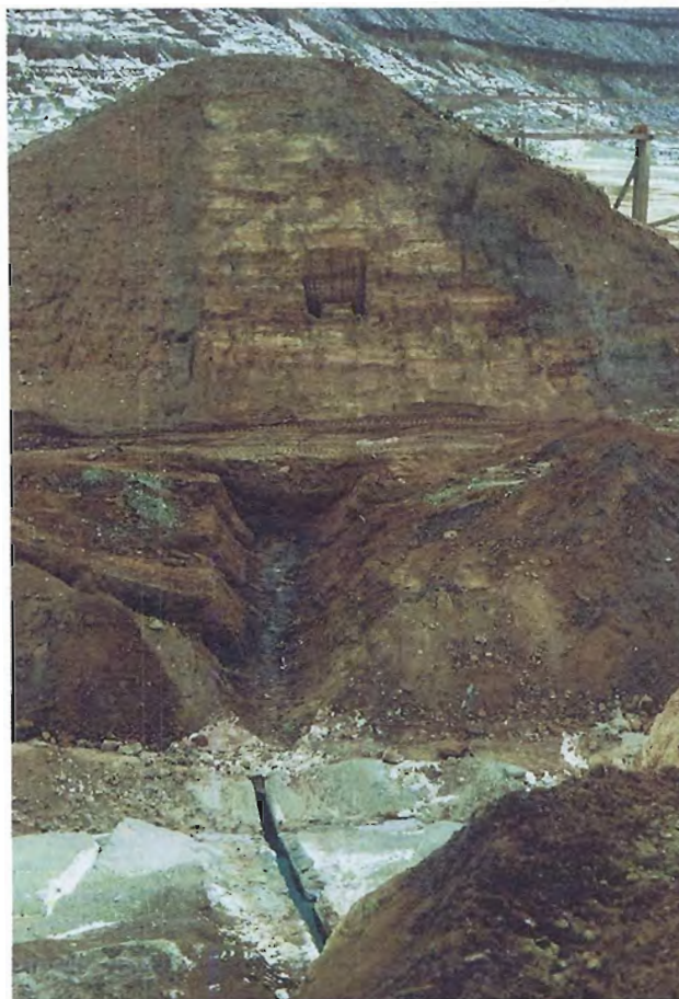
16. Right abutment of breach after excavation of the cutoff trench.
