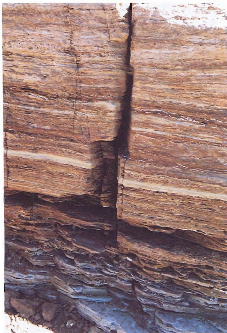
29. View of openings in bedding in breach area.
