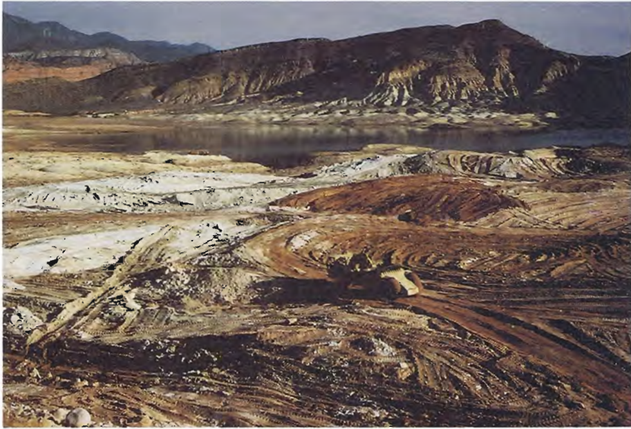
9. Blanketing upstream from center of dike. (10-30-86)
