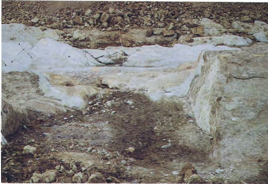
41. View of cutoff trench exposed in breach section. Zone II embankment was present at base of cutoff trench.
