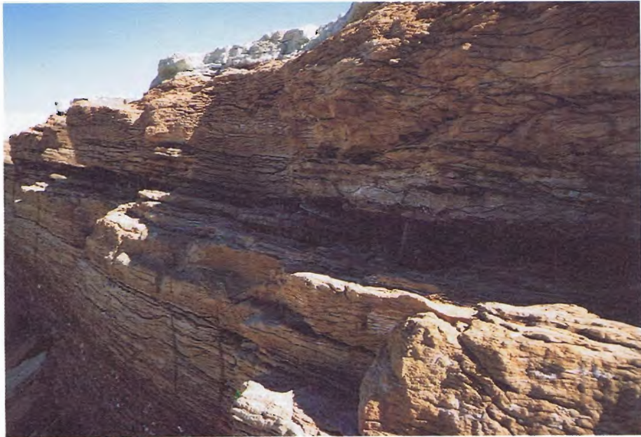
25. Erosion along bedding in breach area.
