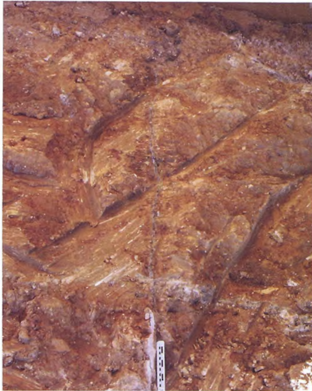
57. Grout-filled seam through Zone I on left side of breach.
