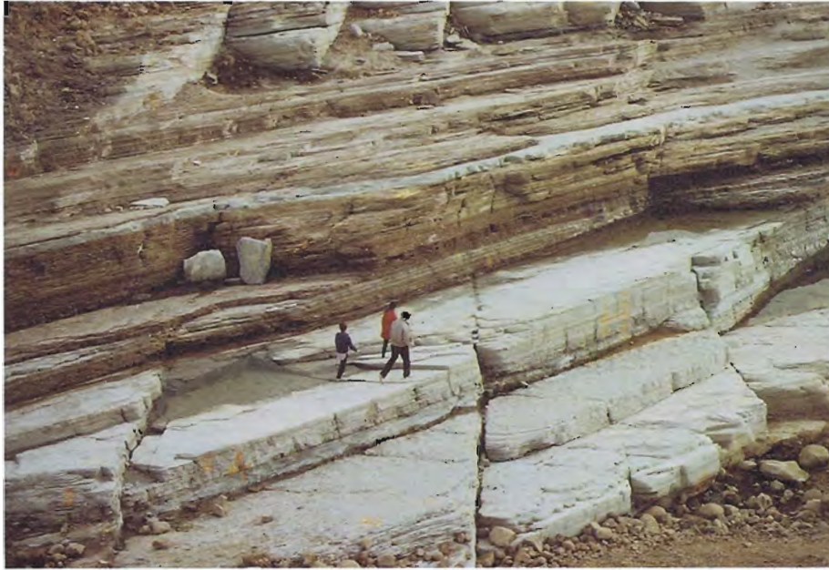
17. Major joint system in units 4 & 5 at site, North 20 degrees West set trends up and down and North 29 degrees East set trends across picture.
