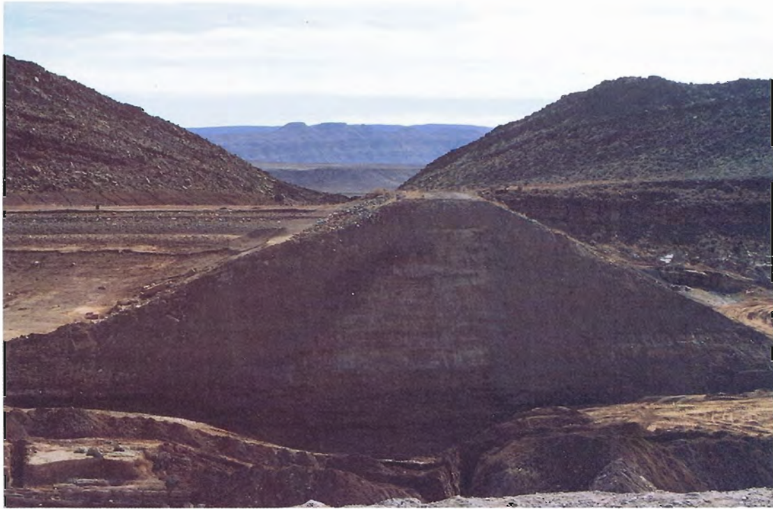
42. View of left embankment showing zoning remaining following sloping of breach side.
