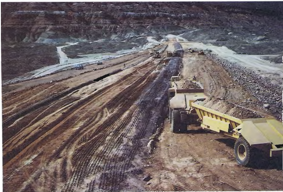
10. View eastward from left abutment showing zones in fill. (4-84)
