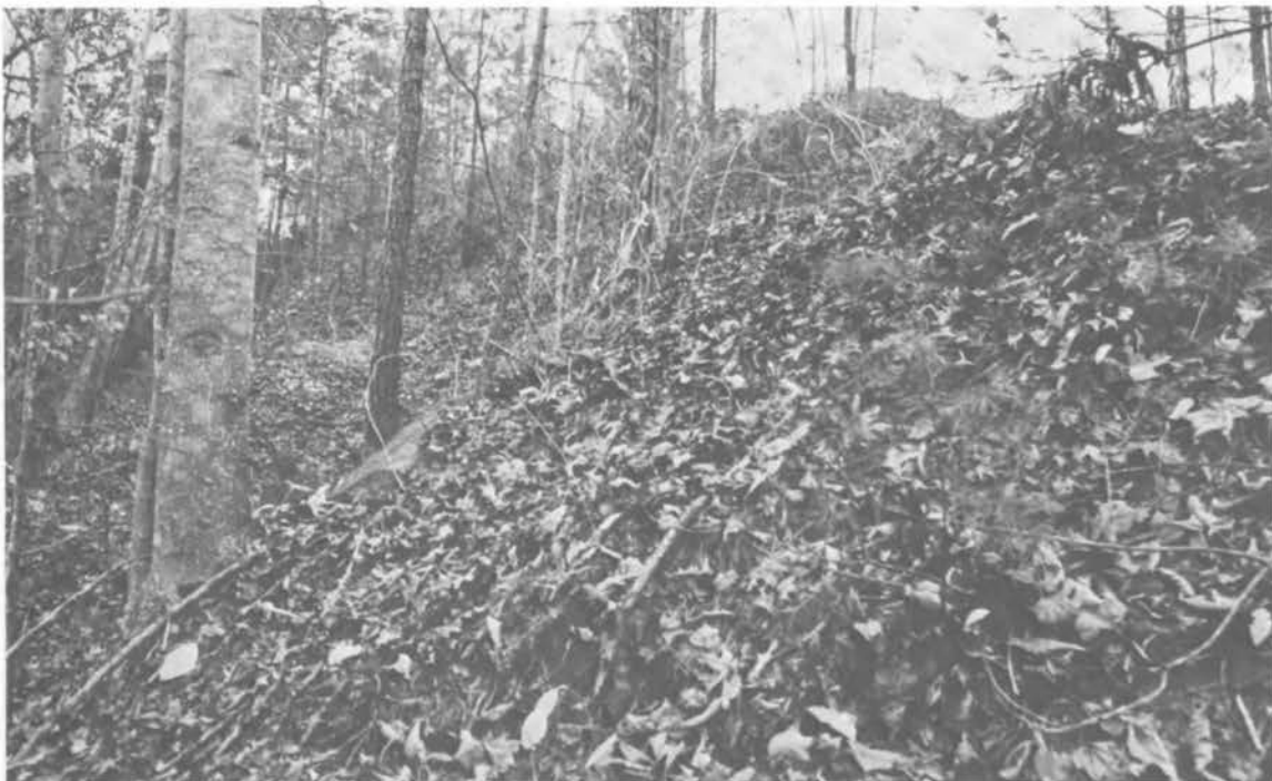
FIGURE 8 Right downstream face, 10-in. tulip poplar, 6 to 8-in. pines, old slide scar
