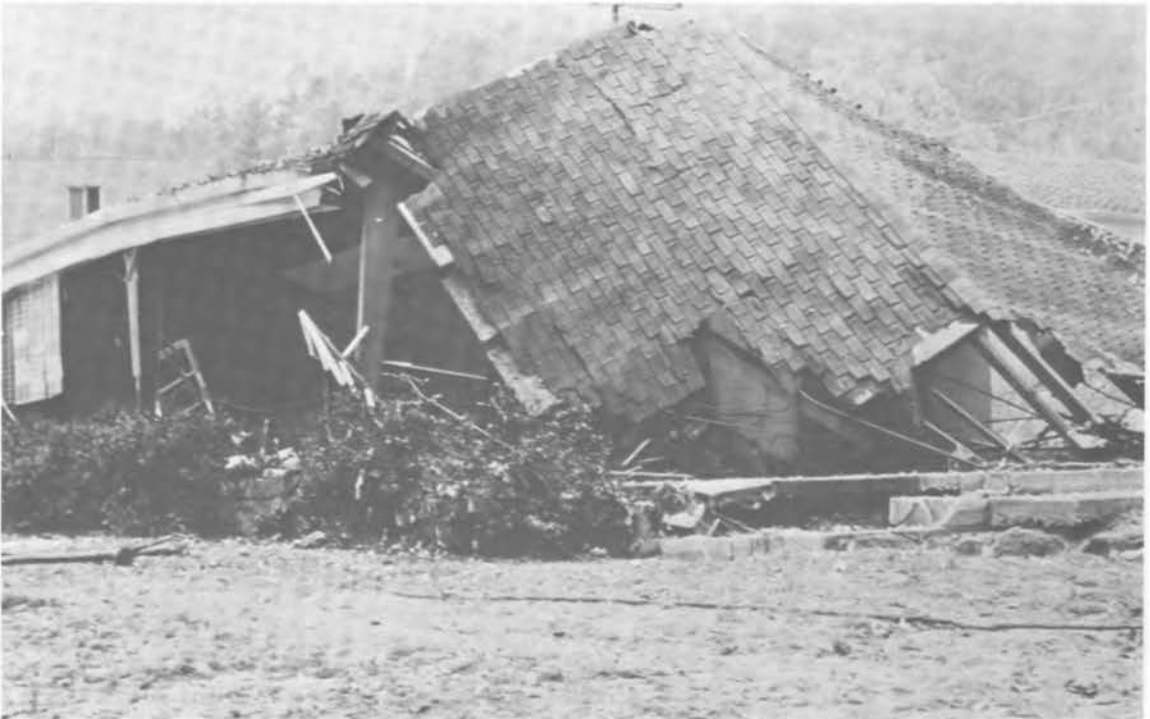
FIGURE 12 Damaged cottage downstream from dormitory
