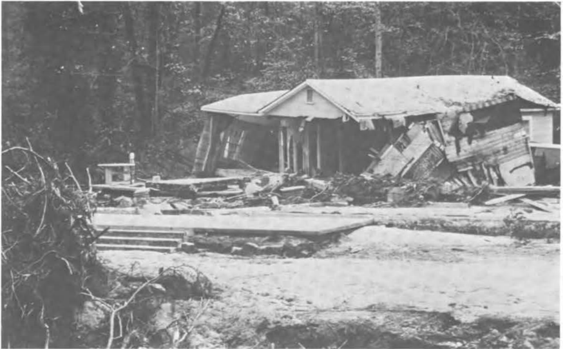
FIGURE 11 Damaged faculty home on right bank across from dormitory
