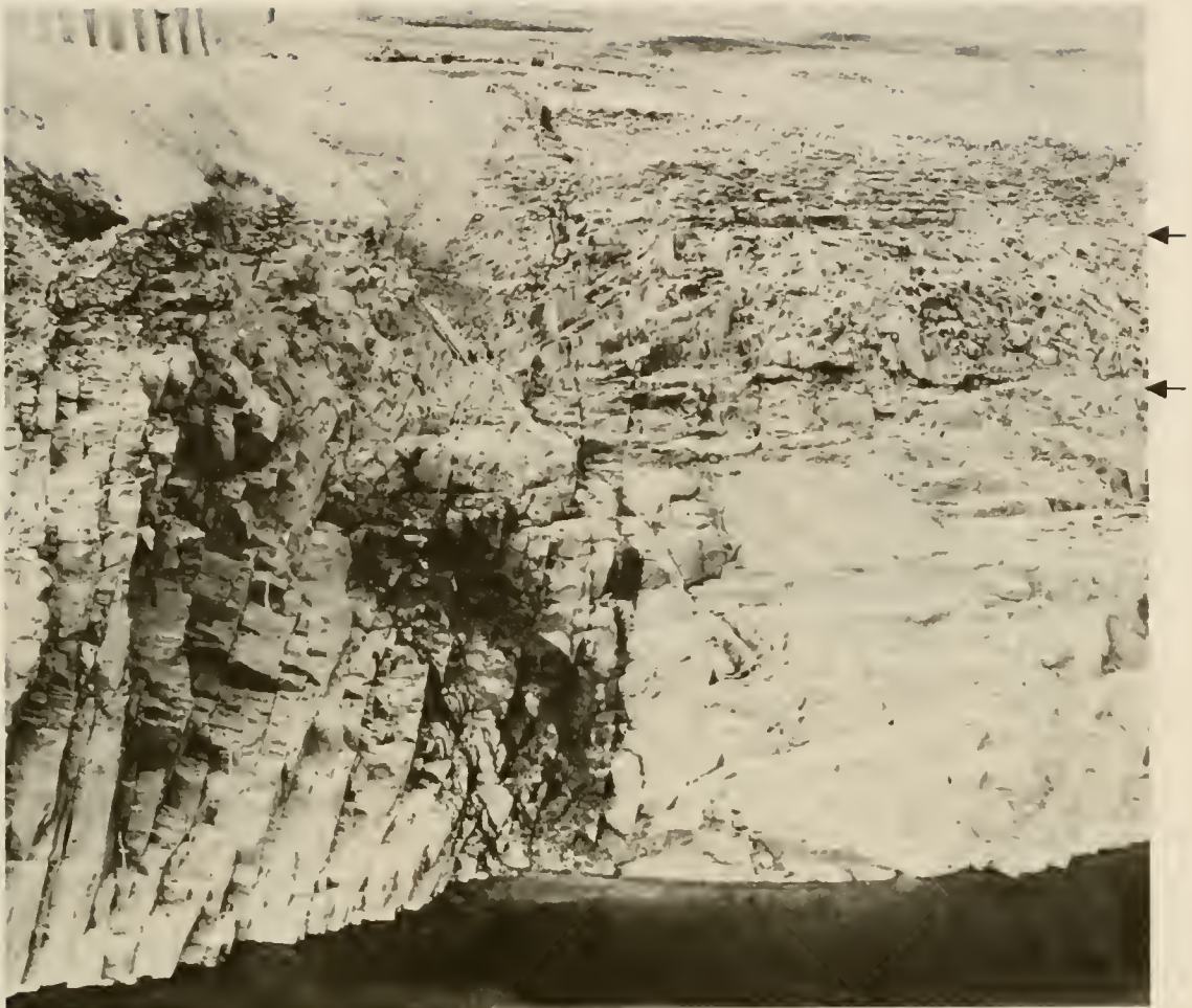
Figure B9.—Aerial view of right abutment in November 1976, after embankment material removed from key trench. Small area of loose fill on bench in right center is temporary stockpile of excavated embankment material. Grout cap extends diagonally across center of photograph. Gap in grout cap between two throughgoing near-vertical joints is at grout cap centerline stations 13+98 to 14+22. The exposed rock is welded tuff. Upper arrow indicates the nearly horizontal contact between unit 1 (above, with platy joints) and unit 2. Lower arrow indicates the unit 2-unit 3 contact, which extends downstream (to the left) about 50 feet beyond the grout cap, where it apparently is abruptly terminated by a high-angle joint. Dark area in lower center is water from abutment cleanup operation. View to north-northwest. Photograph by Bureau of Reclamation.
