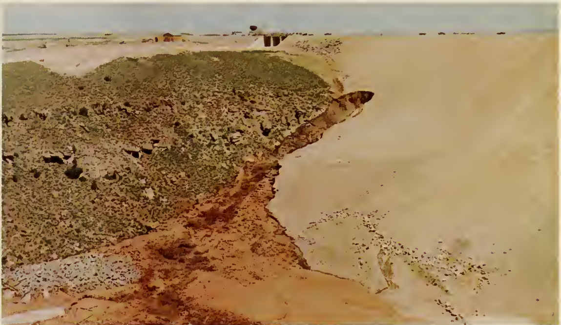
Figure 23.—Dozers lost in leak at El. 5200.
