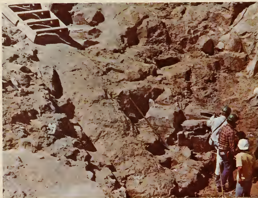
Fig. 3-2 Transverse trenches exposing key-trench invert and grout cap
