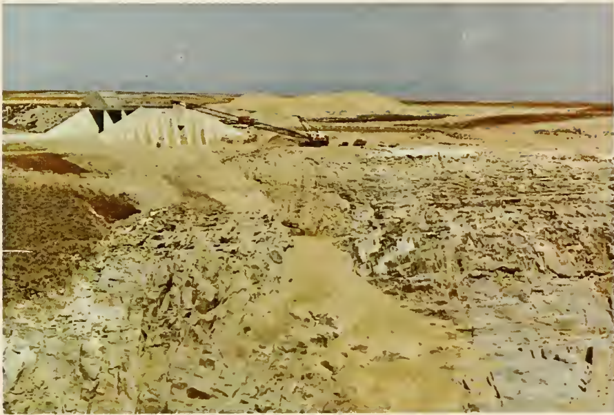
Fig. 3-3 Removal of zone 1 material by crane and skip
