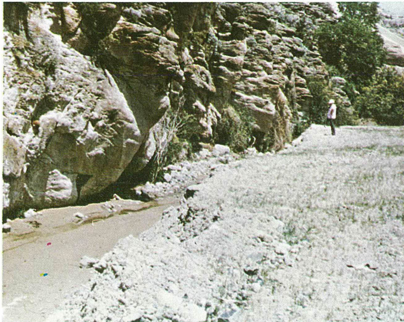
Fig. 2-4. North canyon wall about 1500 feet downstream from Teton Dam. Clear water flowing from rhyolite about 40 gpm. June 3, 1976.
