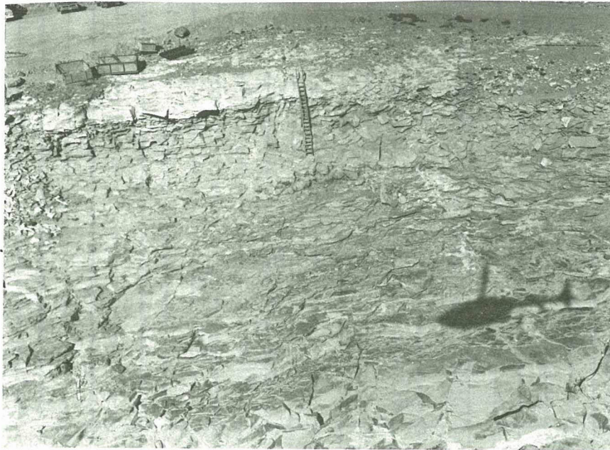
Fig. E-1 Right wall of Teton Canyon upstream of dam axis showing intensive jointing in uppermost rock zone. (post-failure)
