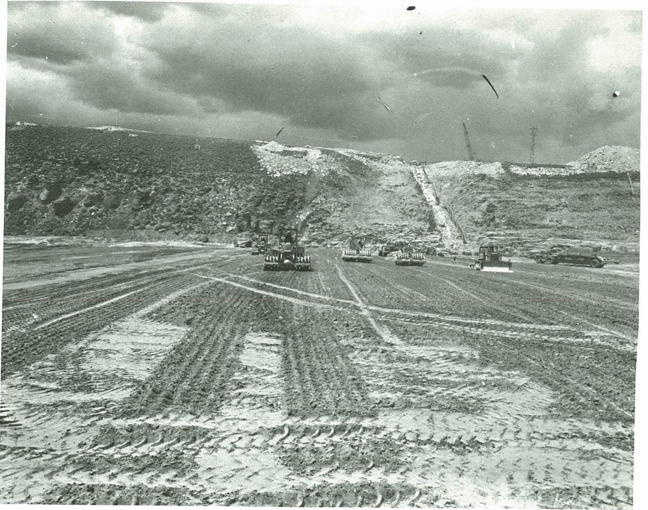
Project Photo P 549-147-5733 NA 5/27/75 Embankment at 5150
