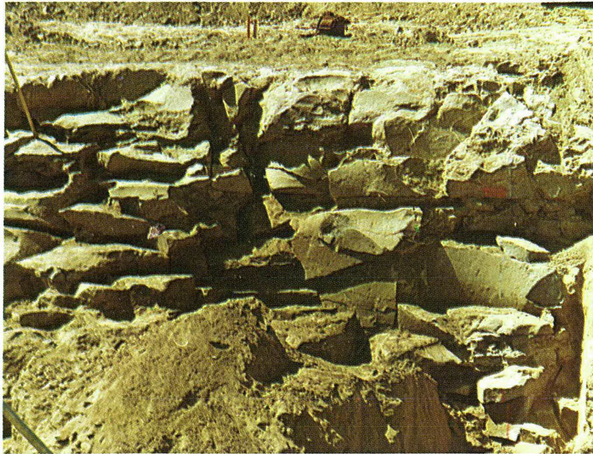
Fig. 5-10 Slab-like structure in Unit 1 of ash-flow tuff exposed in rim of downstream wall of keyway in right abutment. (post-failure photo)
