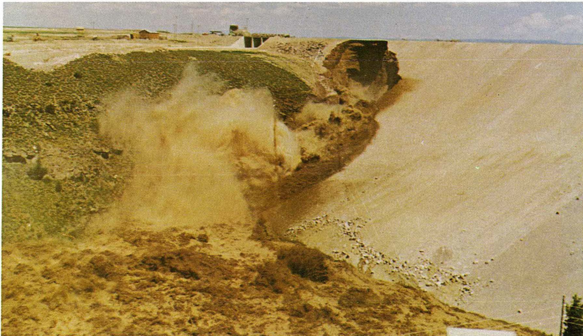
Fig. 2-14. Dam crest breaching. 11:55 a.m. June 5, 1976.
