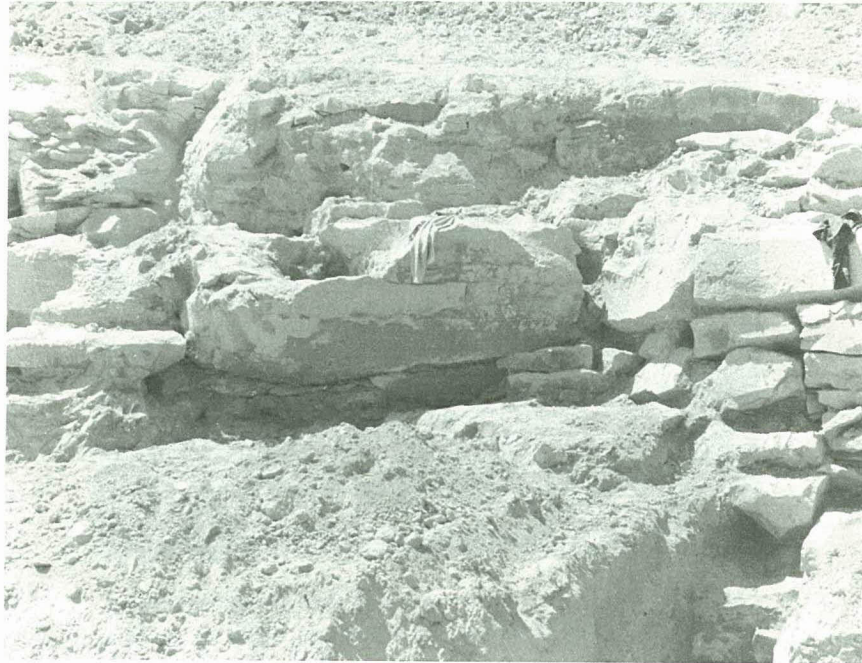
Fig. E-7 Downstream face of key trench in right abutment at El. 5290. (post-failure)
