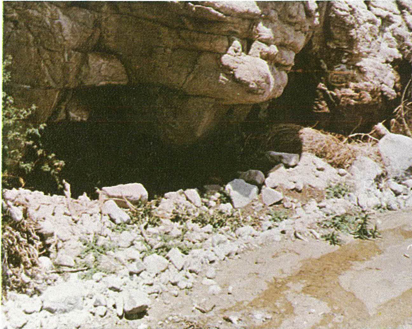
Fig. 2-3. North canyon wall about 1300 feet downstream from Teton Dam. Clear water from several small seeps flowing about 60 gpm. June 3, 1976..
