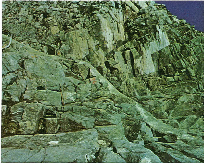
Fig. 3-15 Rock structure along grout cap alignment Stas. 13+30 to 13+96, downstream profile
