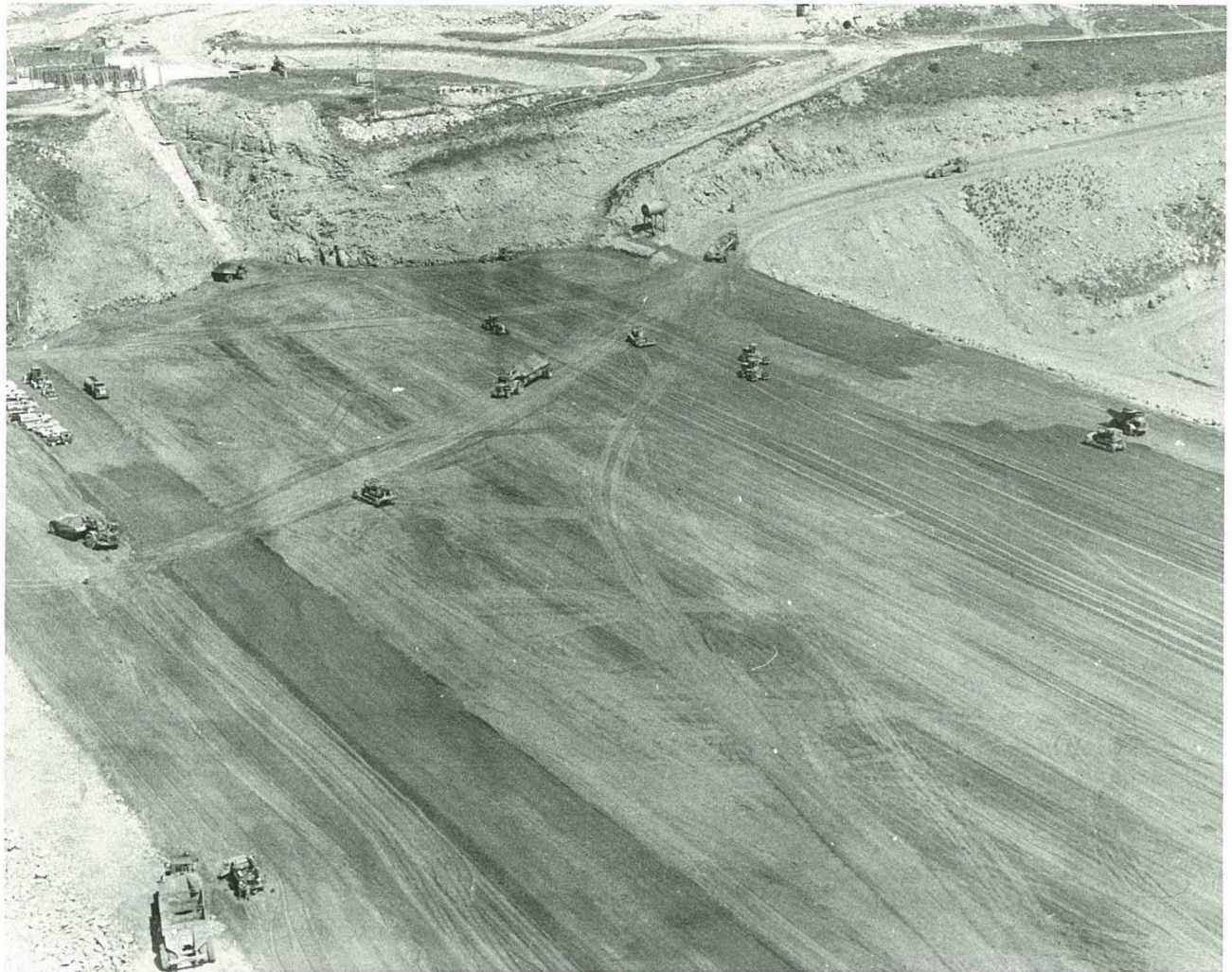
Project Photo P 549-147-5883 NA 7/22/75 Embankment at 5185
