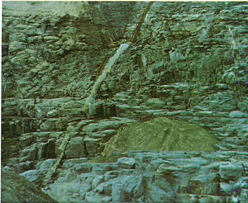
Fig. 3-9 Post-failure exposure of the grout cap
