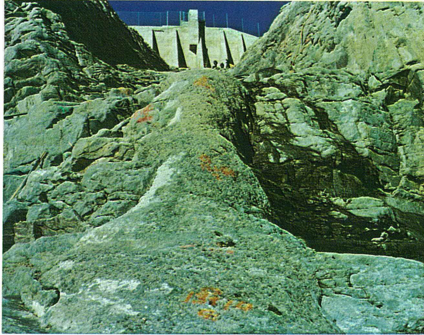
Fig. 3-13 Rock structure along grout cap alignment Stas. 13+30 to 13+96
