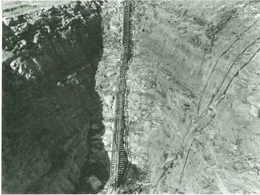
Fig. E-17 Key trench excavation on right abutment. (post-failure)
