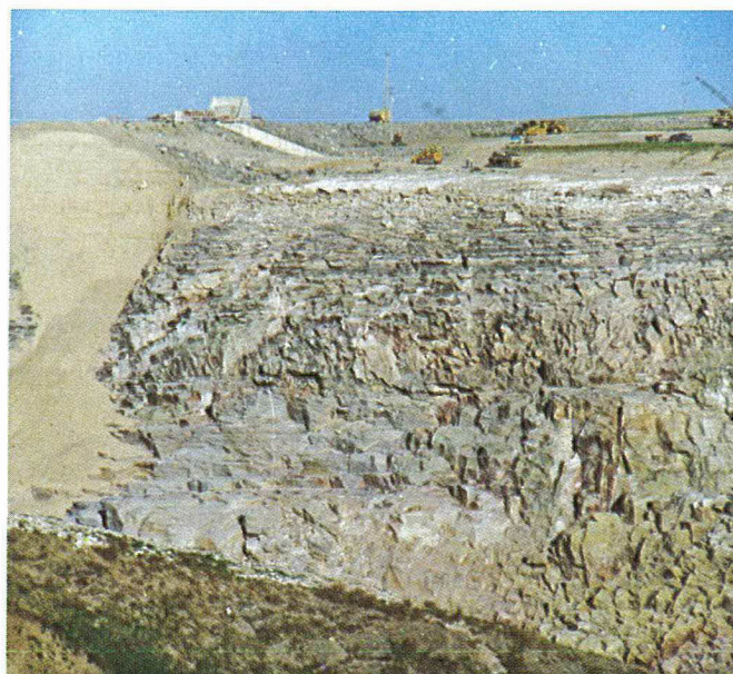
Fig. 5-11 Joint pattern in Unit 2 of ash-flow tuff, right wall of canyon upstream from key trench. (post-failure photo)
