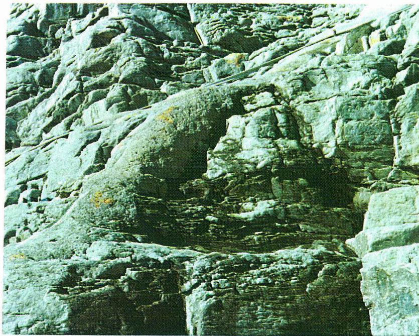
Fig. 3-14 Rock structure along grout cap alignment Stas. 13+30 to 13+96, upstream profile
