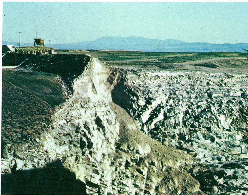
Fig. 9-3 Foundation formation and contact beneath zone 2 and zone 5
