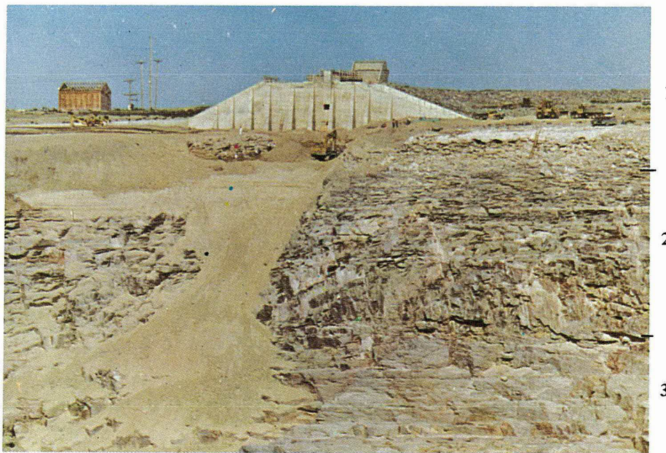
Fig. 5-9 The ash-flow tuff upstream of dam axis is divided into three units (post-failure photo)
