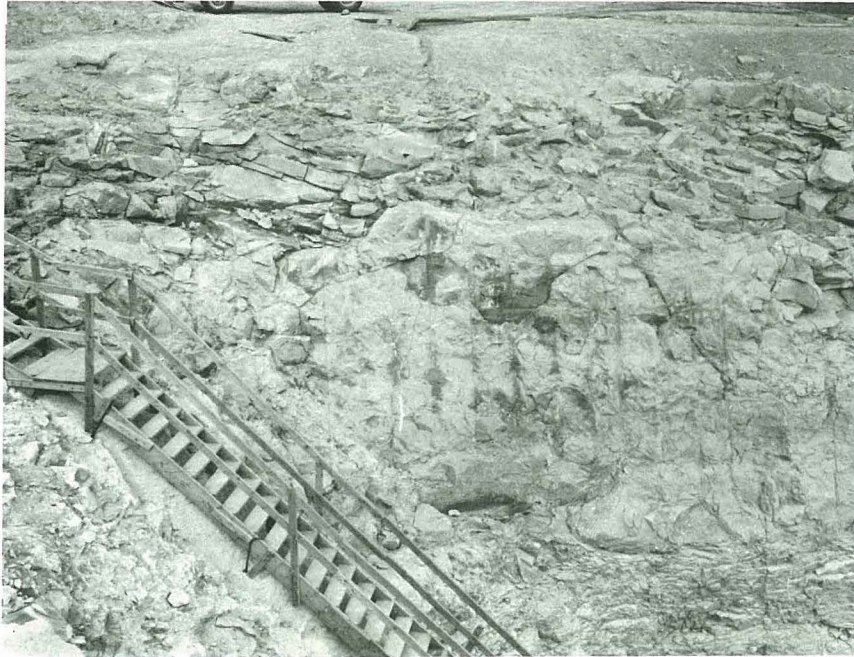
Fig. E-13 Rim of upstream wall of right abutment key trench. (post-failure)
