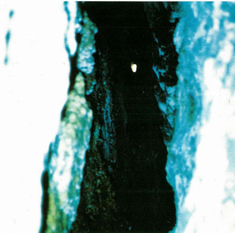
Fig. 5-18 Interior of fissure shown in Fig. 5-17. Photo taken 10 ft from upstream wall of key trench. Spot in background is light from a bulb suspended through a 6-in. vertical drill hole located about 25 ft from camera. (1974)
