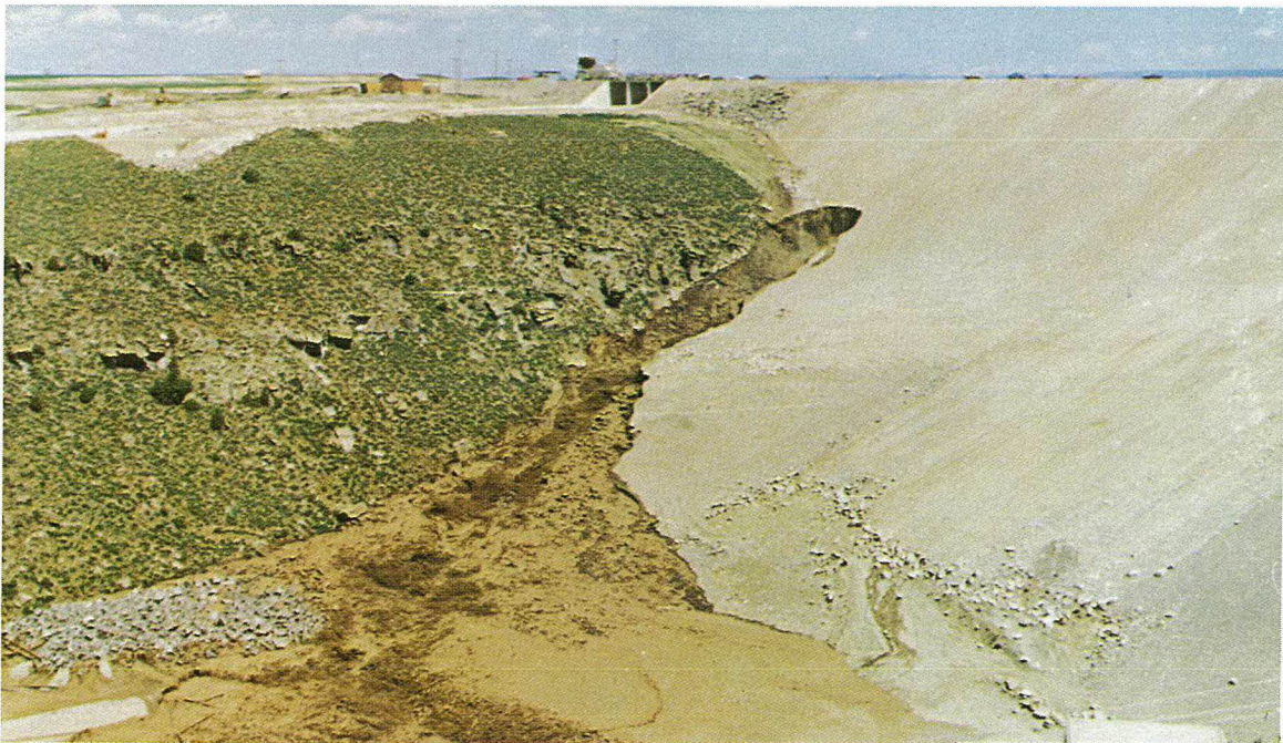
Fig. 2-10. Dozers lost in hole. About 11:20 a.m. June 5, 1976.
