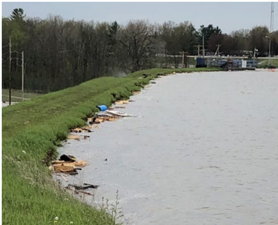
Figure 8: Enlarged photograph showing the upstream side of the Edenville left embankment at 5:31 p.m., Tuesday, May 19, 2020
