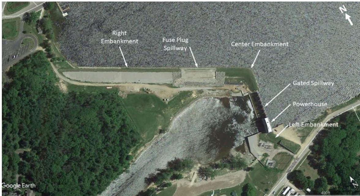
Figure 3: Sanford Dam configuration
