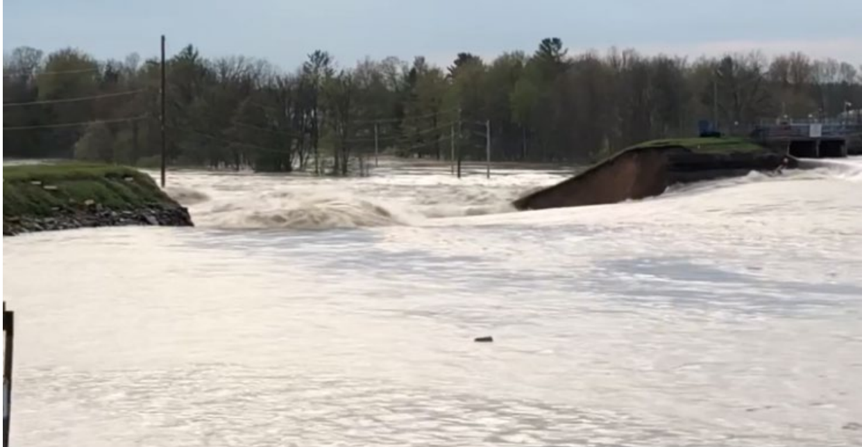
Figure 20: Edenville left embankment breach at 7:13 p.m. on Tuesday, May 19, 2020
