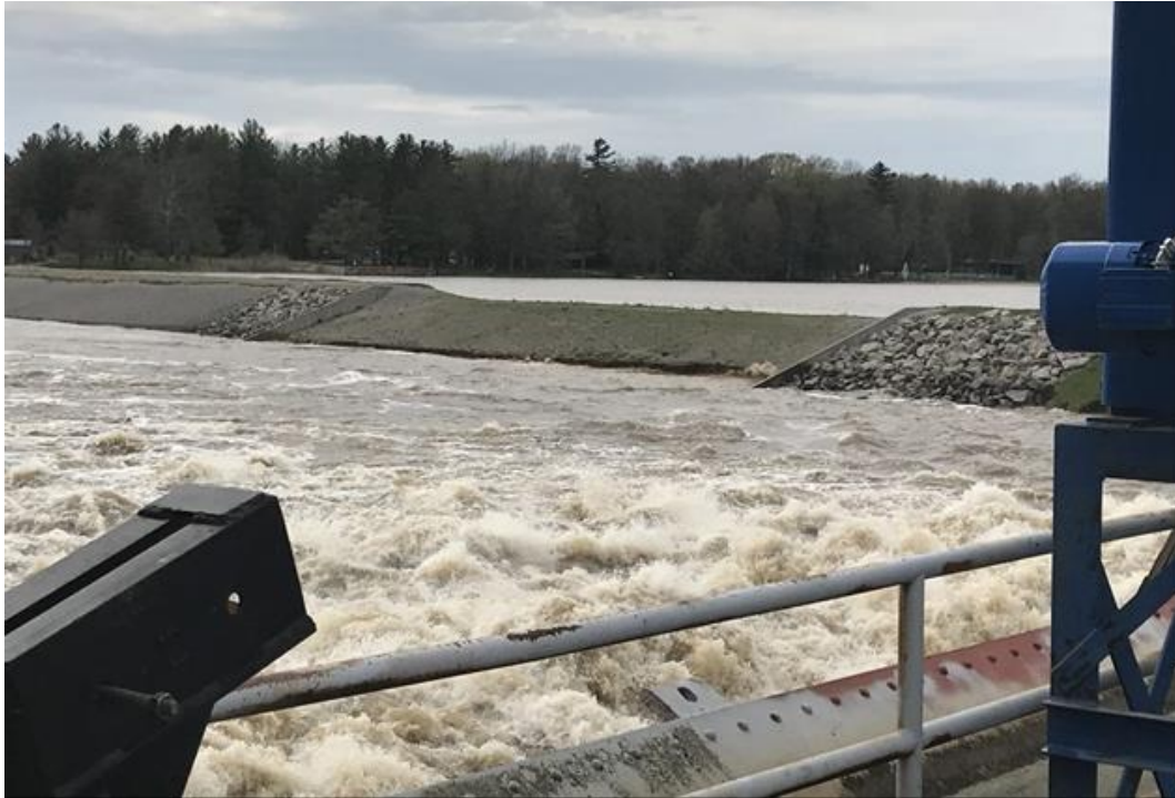
Figure 3-20: Erosion along Toe of Fuse Plug Prior to Overtopping (photo courtesy of EGLE)
