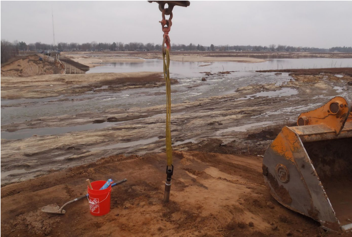
Figure E-7: Shelby Tube Collection from Left Breach Remnant
