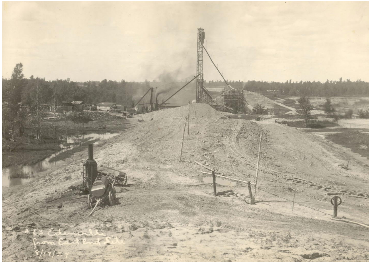
Fill placed in lower portion of Edenville east (left) embankment. Note material in background stockpiled in downstream portion of the embankment. Note the downstream area of the embankment at a slightly higher elevation than the upstream. Aspen poles used for construction utilities are visible [representative of an aspen pole observed in the embankment fill of the remnant right face of the embankment breach] (August 1924)
