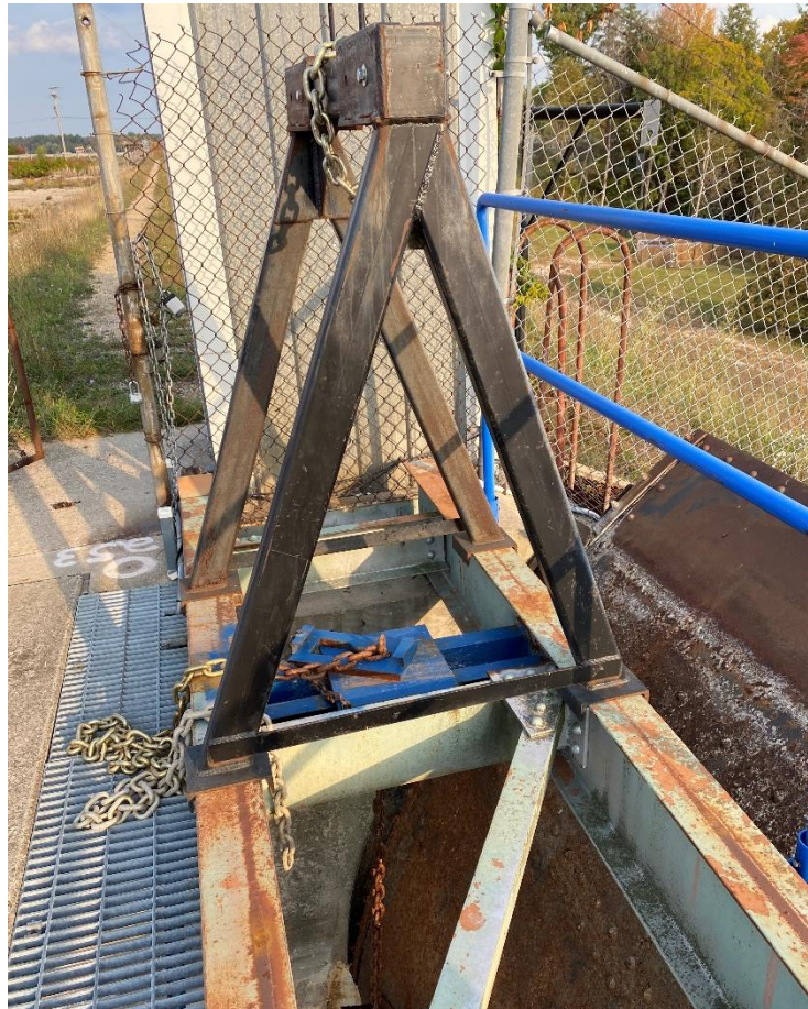
Figure 2-7: A-Frame Hoisting System in Place at Tobacco Spillway
