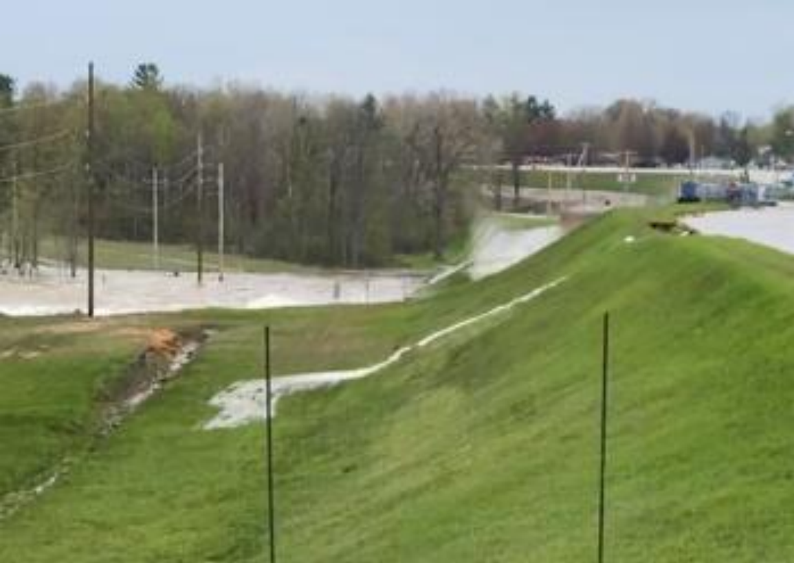
Figure 3-7: Enlarged Still Image from Dam Failure Video at 4 Seconds
