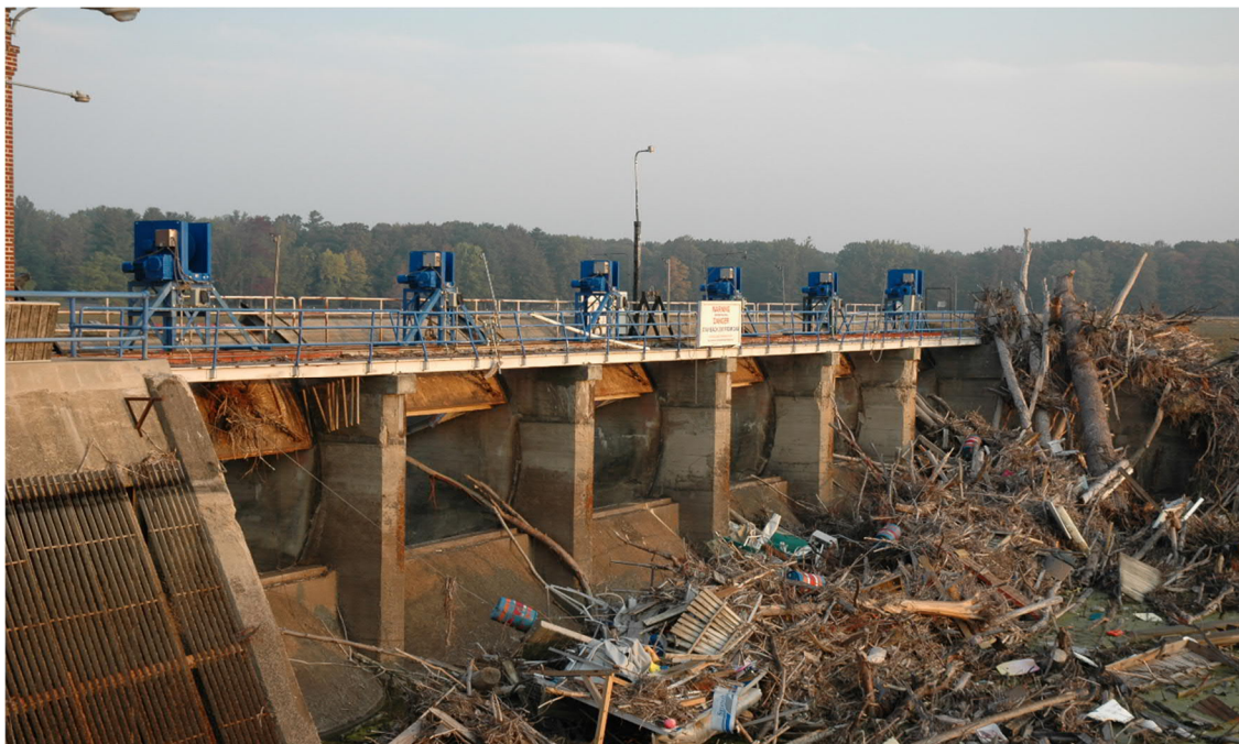
Figure F1-29: Sanford Spillway – September 2020
