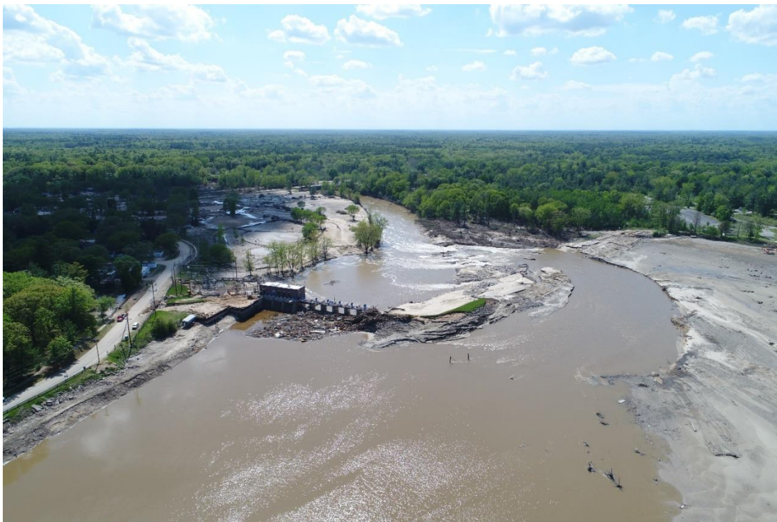
Figure 3-19: Sanford Dam Failure, Viewed from Upstream (photo courtesy of EGLE)
