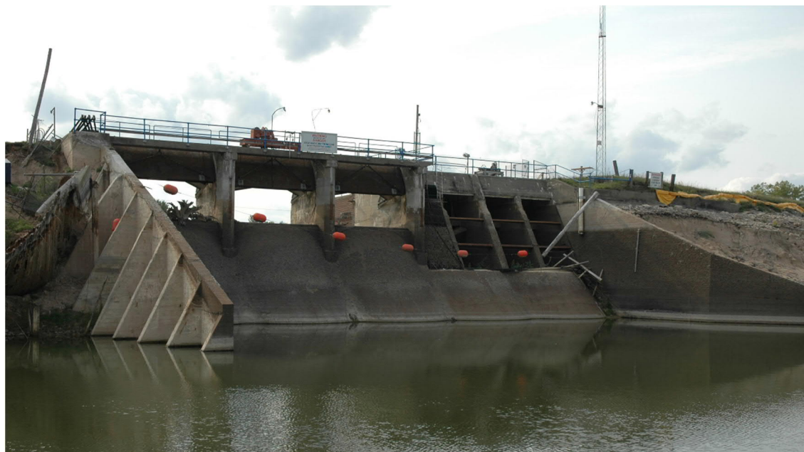
Figure F1-28: Edenville Spillway – September 2020
