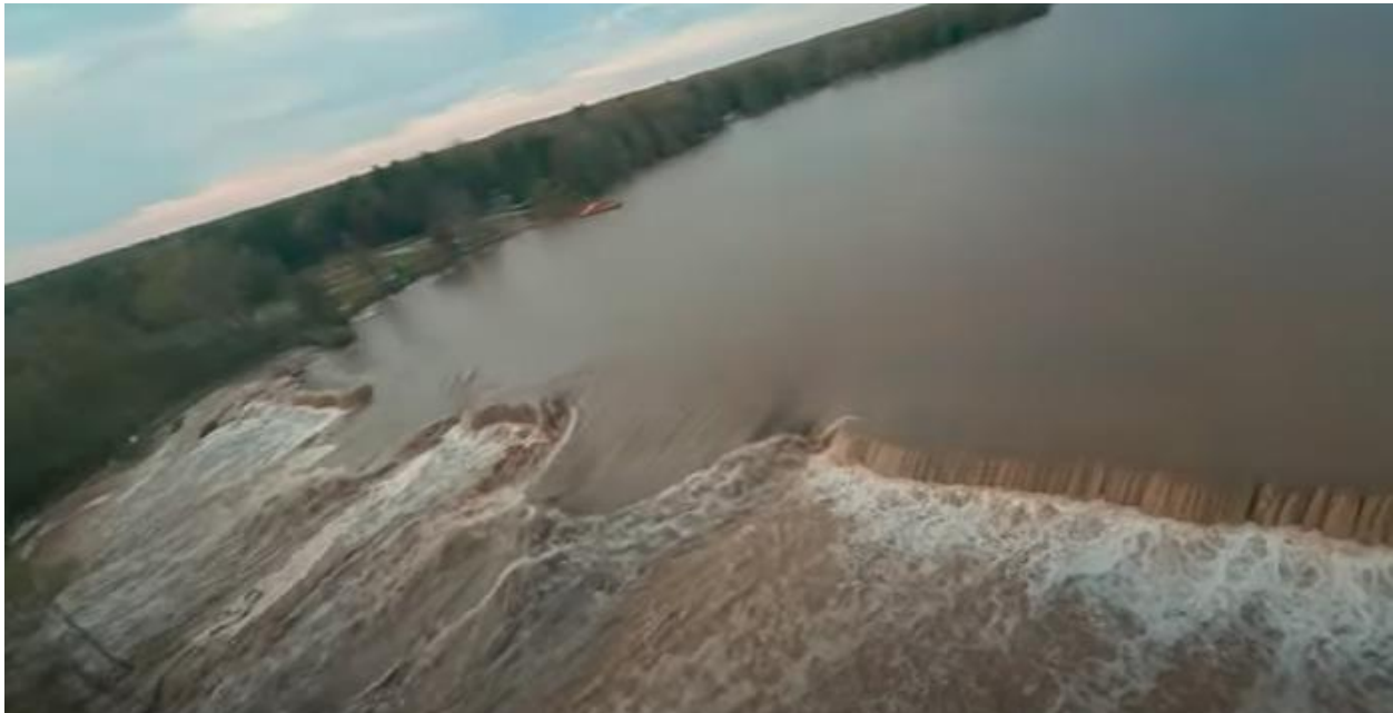
Figure 3-25: Still Image from Drone Video at Approximately 8:20 P.M. with Breach Beginning along Sections of Right Embankment.
