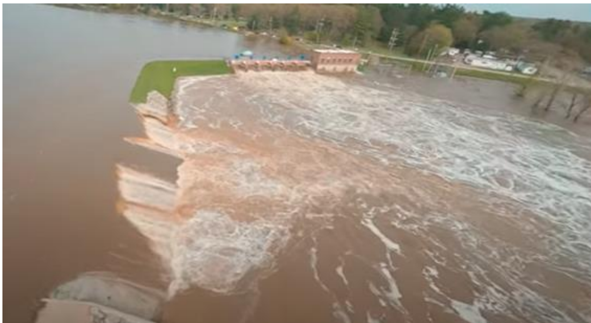
Figure 3-23: Still Image from Drone Video Approximately 7:46 P.M., Just Before the Initial Embankment Overtopping
