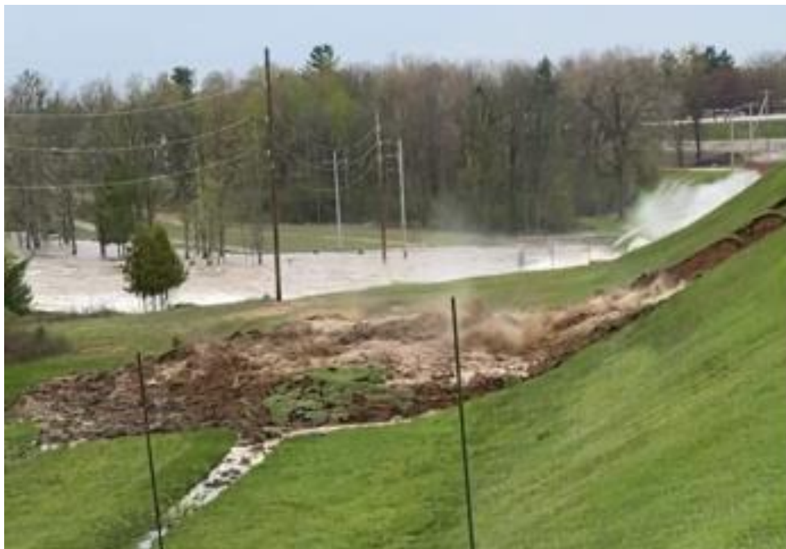
Figure 3-13: Enlarged Still Image from Dam Failure Video at 28 Seconds
