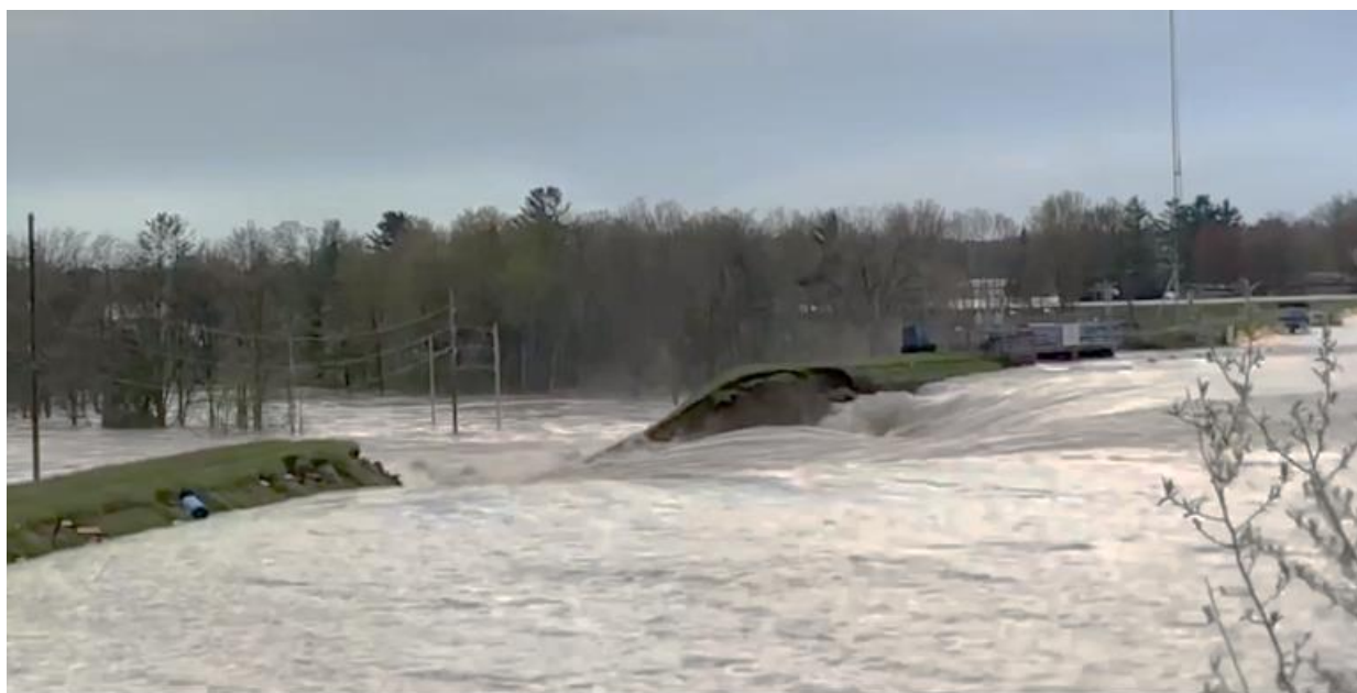
Figure 3-16: Edenville Left Embankment Breach at 6:24 P.M. on Tuesday, May 19, 2020
