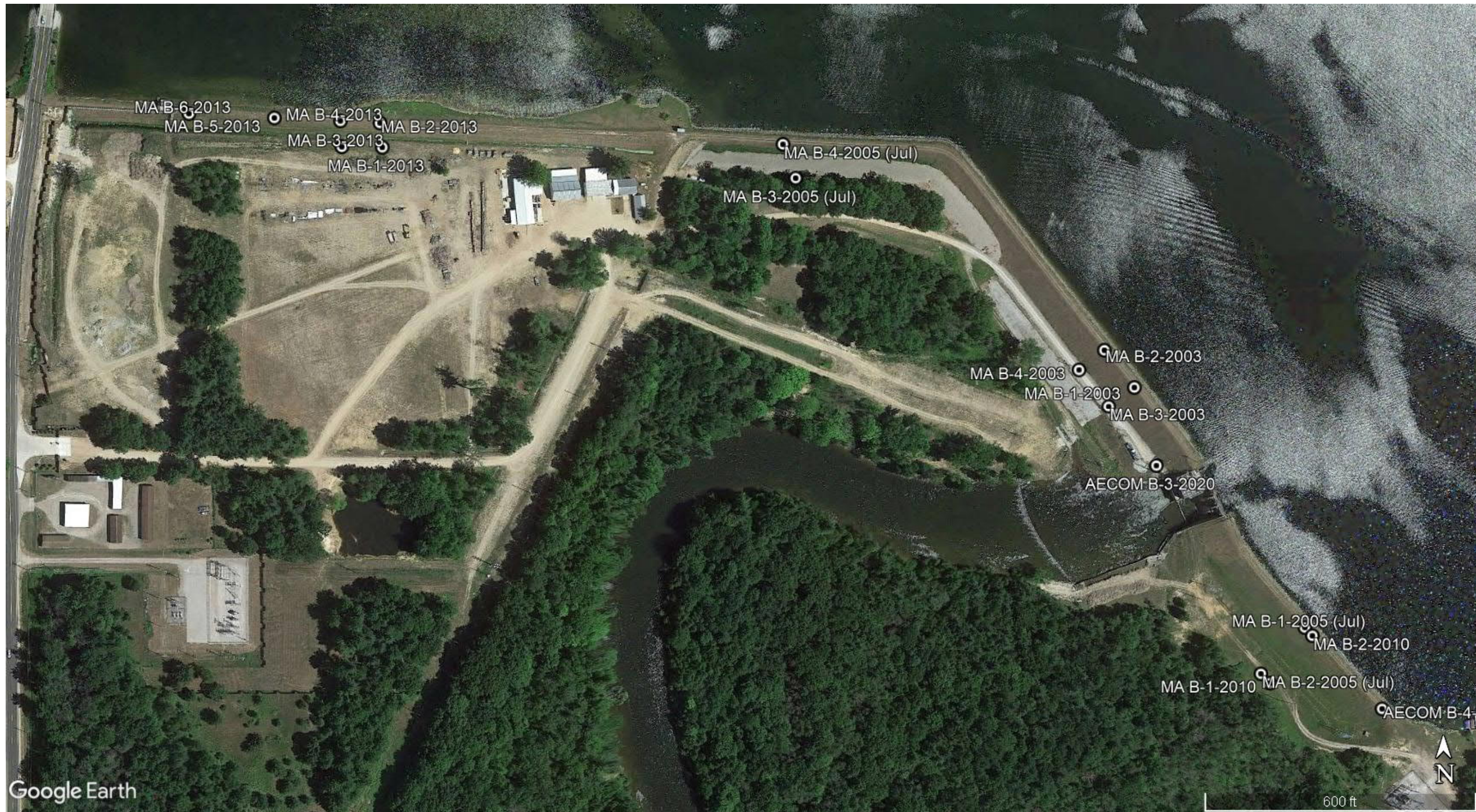
Figure B-3: Edenville Embankment – Historic Investigations
