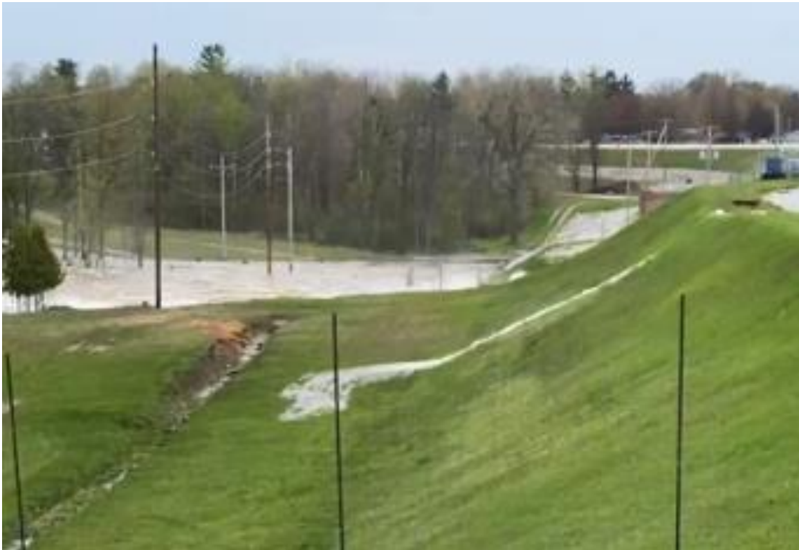
Figure 3-6: Enlarged Still Image from Dam Failure Video at 0 Seconds
