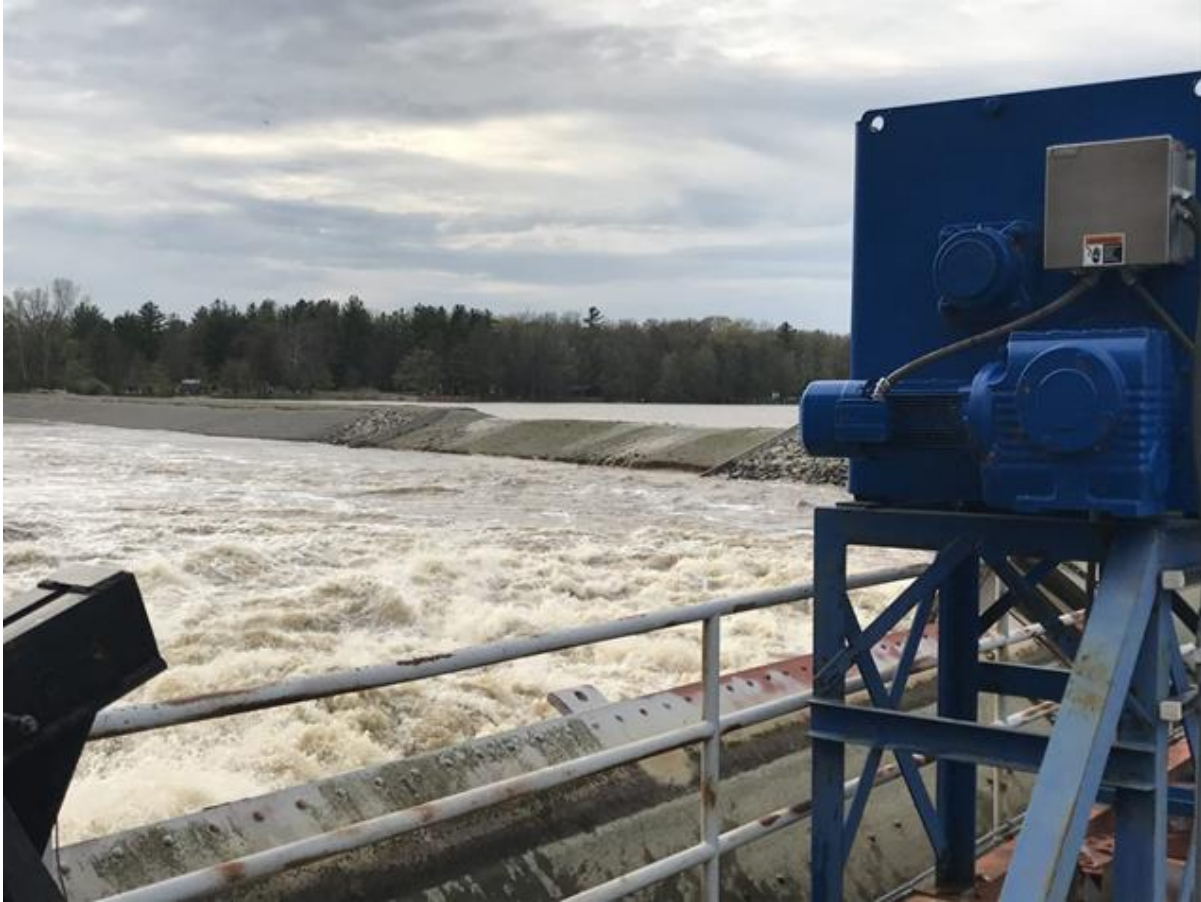
Figure 3-21: Initial Overtopping of Fuse Plug at about 7:19 P.M. (photo courtesy of EGLE)
