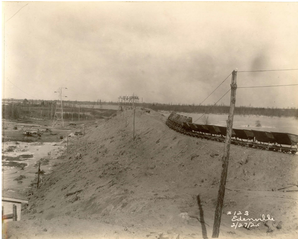
Fill placed in Edenville east (left) embankment near top-out elevation. Note what appears to be a slightly steeper slope near the top elevation. Note lake level in right background of photo. Note water along downstream toe (later construction memos [April 1925] will note that the downstream toe of this embankment is dry). (February 1925)
