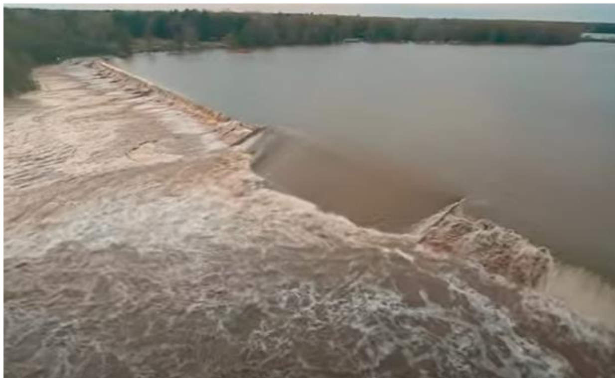
Figure 3-24: Still Image from Drone Video at Approximately 8:11 P.M. (Note almost complete washout of fuse plug and entire embankment being overtopped.)
