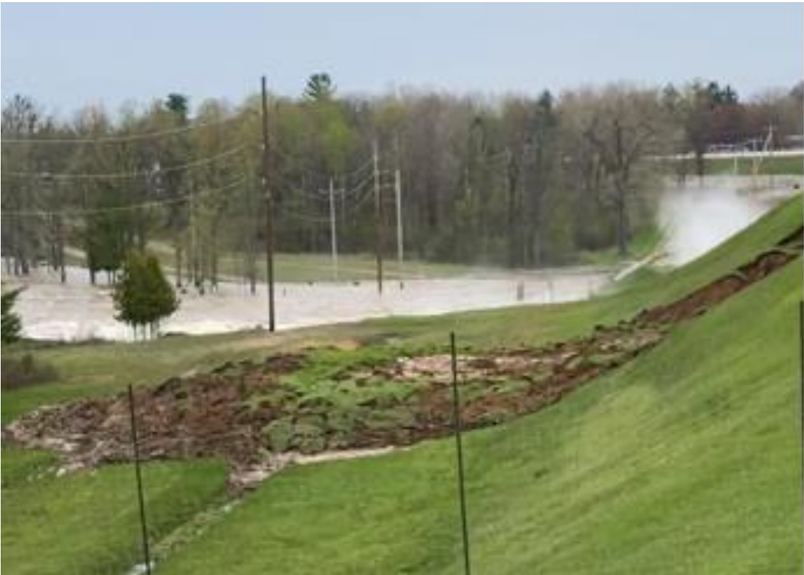
Figure 3-12: Enlarged Still Image from Dam Failure Video at 15 Seconds
