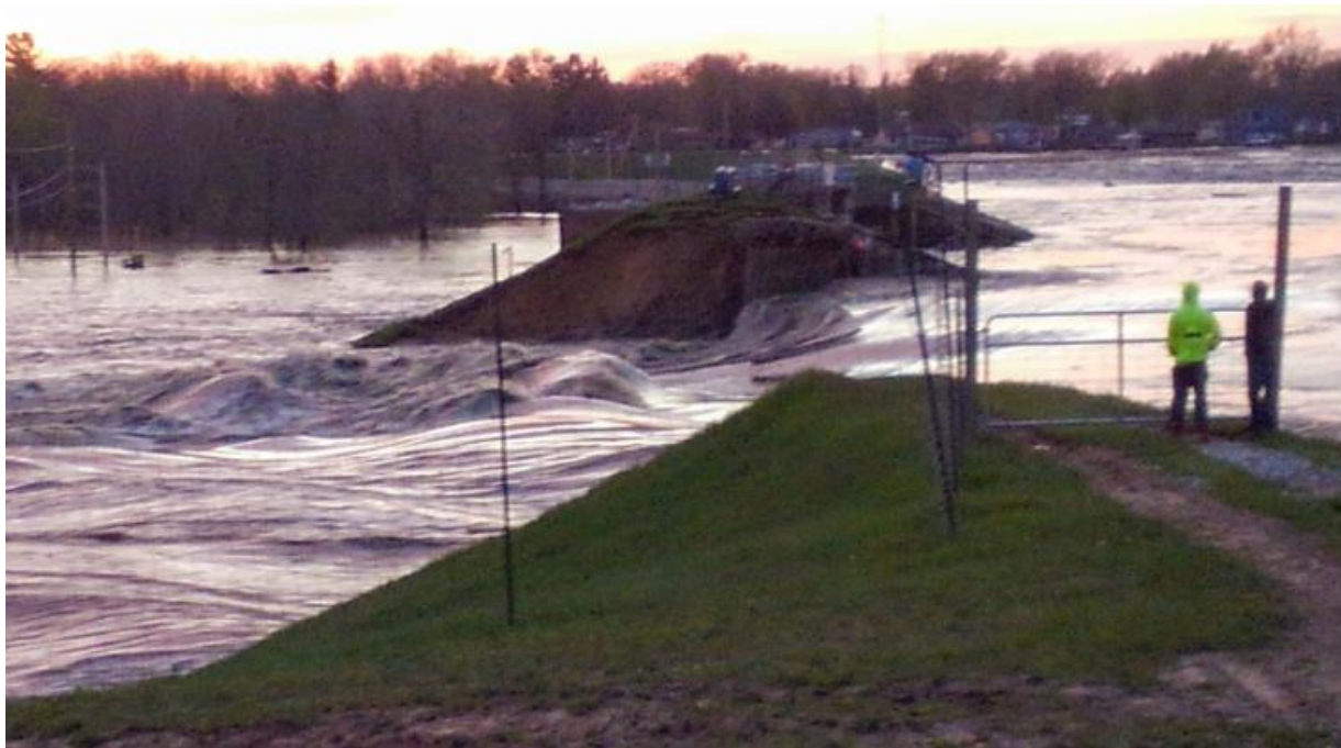
Figure 3-18: Edenville Left Embankment Breach at 9:04 P.M. on Tuesday, May 19, 2020
