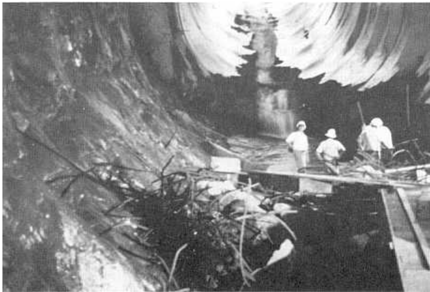
b. Right tunnel
