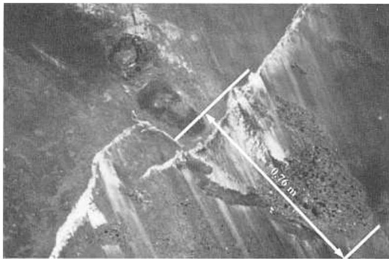
b. Damage observed on June 6, 1983
