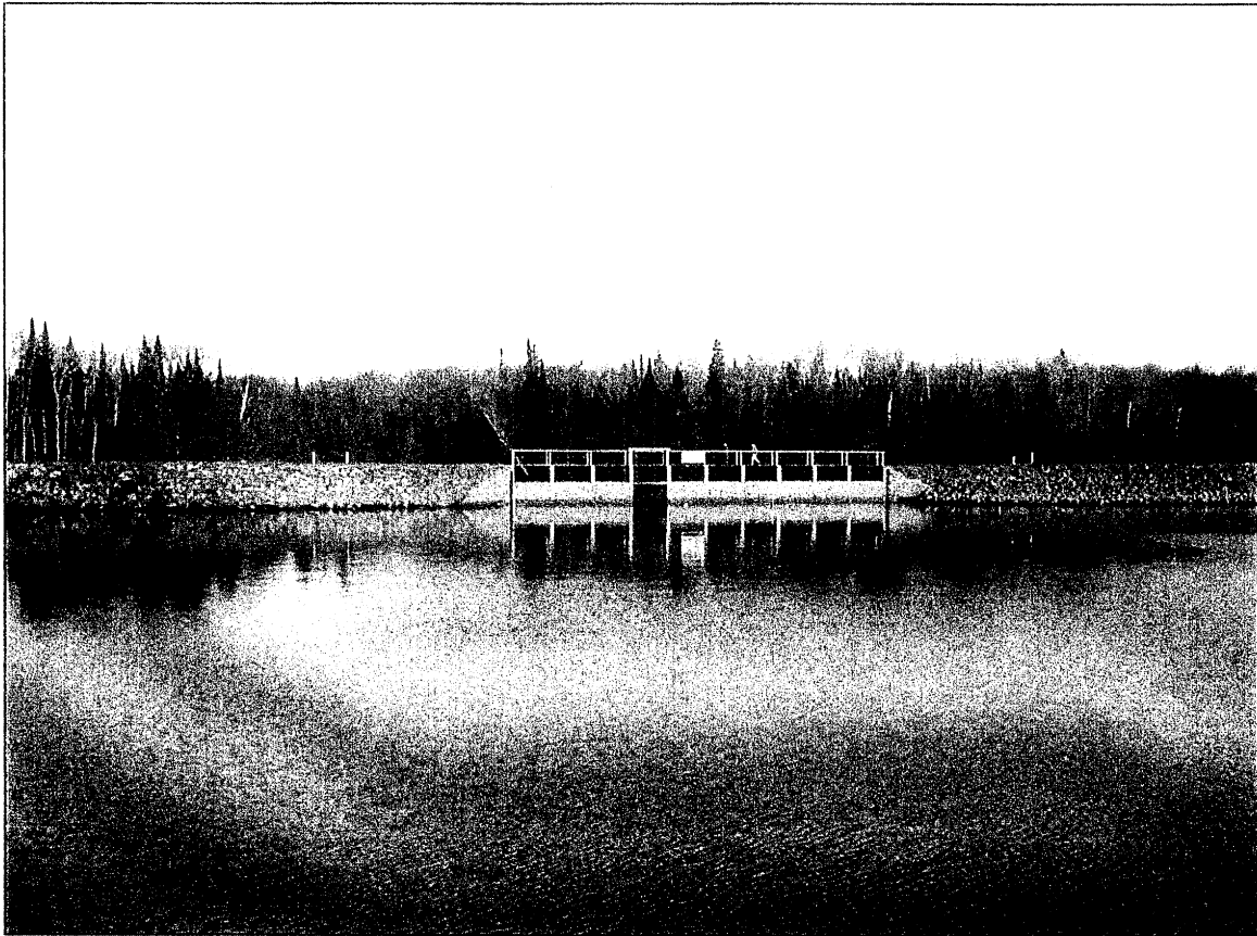
Figure 3.6.2-2 Upstream side of concrete spillway at about 8:30 PM, May 14, 2003
