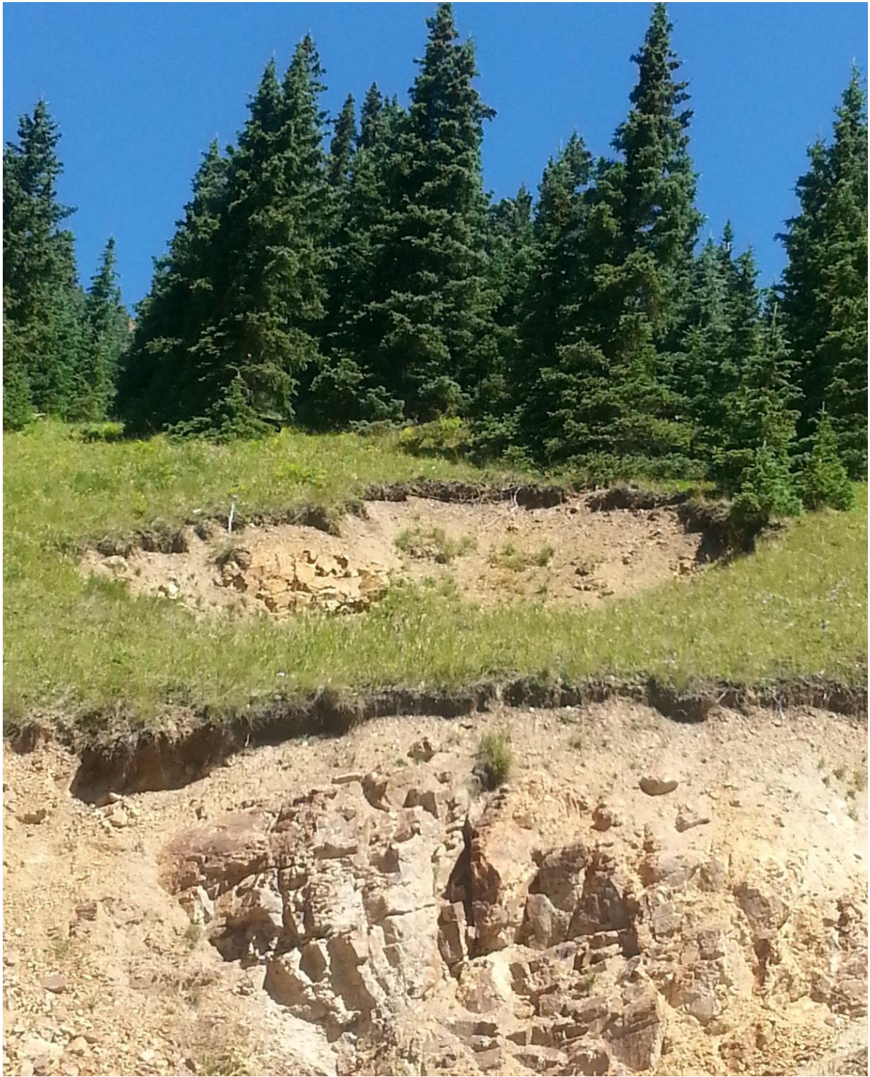
Photo 3 August 18, 2015 – Sink Hole and Slope above Gold King Mine Old Adit
