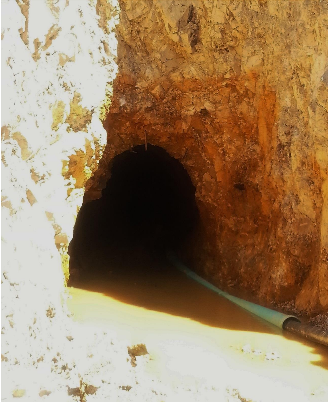
Photo 4 August 18, 2015 – Gold King Mine Level 7 Adit post-blowout
