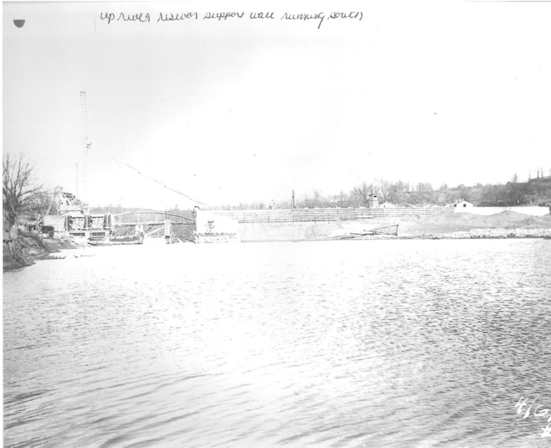
Photo II-1 Upstream side of dam during construction Note corewall and right embankment construction.
