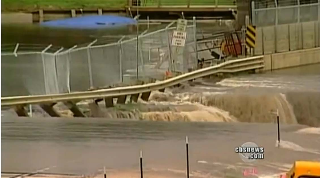
Photo IV-15 Developing breach along two fronts near gated spillway (photo from CBS news video).
