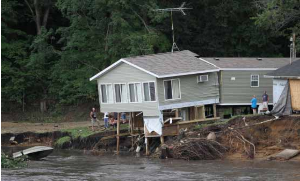
Photo VI-2 Damage and erosion immediately downstream of the dam after the breach 07/24/10
