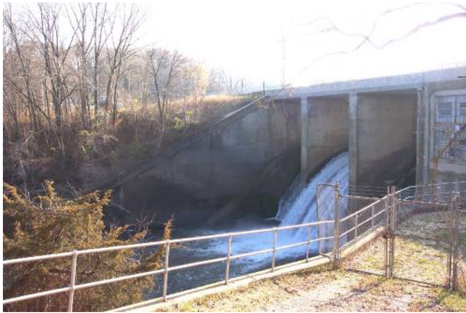
Photo II-5. Vegetation on the downstream embankment slope
