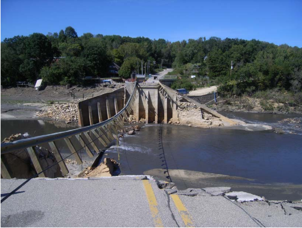
Photo IV-4 South wall of the gated spillway.
