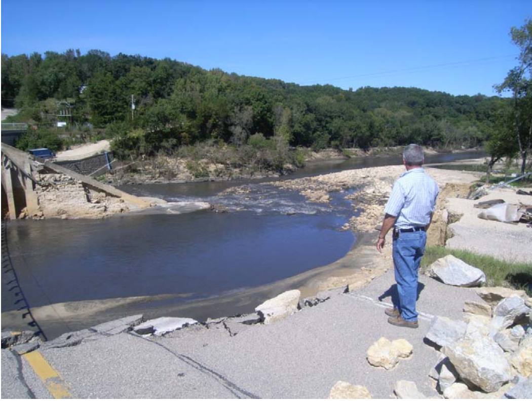
Photo IV-1. Bedrock outcroppings on left valley wall and in current channel.
