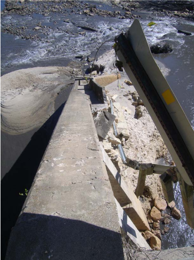
Photo IV-6 Close up of remaining fishway.
