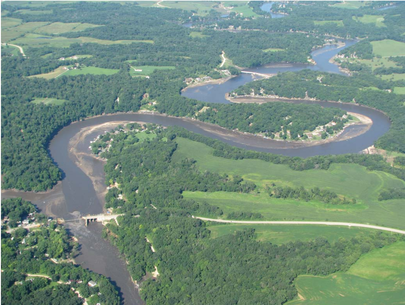
Photo V-1 – Aerial View of Breached Delhi Dam in Foreground and Upstream Bridge in Reservoir
