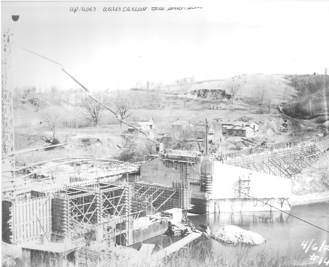
Photo II-2 Embankment core wall construction Note corewall and right embankment construction.
