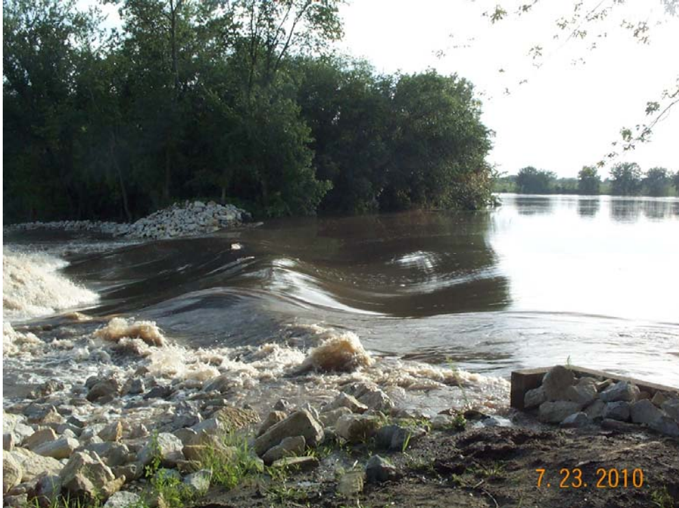
Photo III-2 Quaker Mill Rock Dike in Process of Breaching on 7/23/2010
