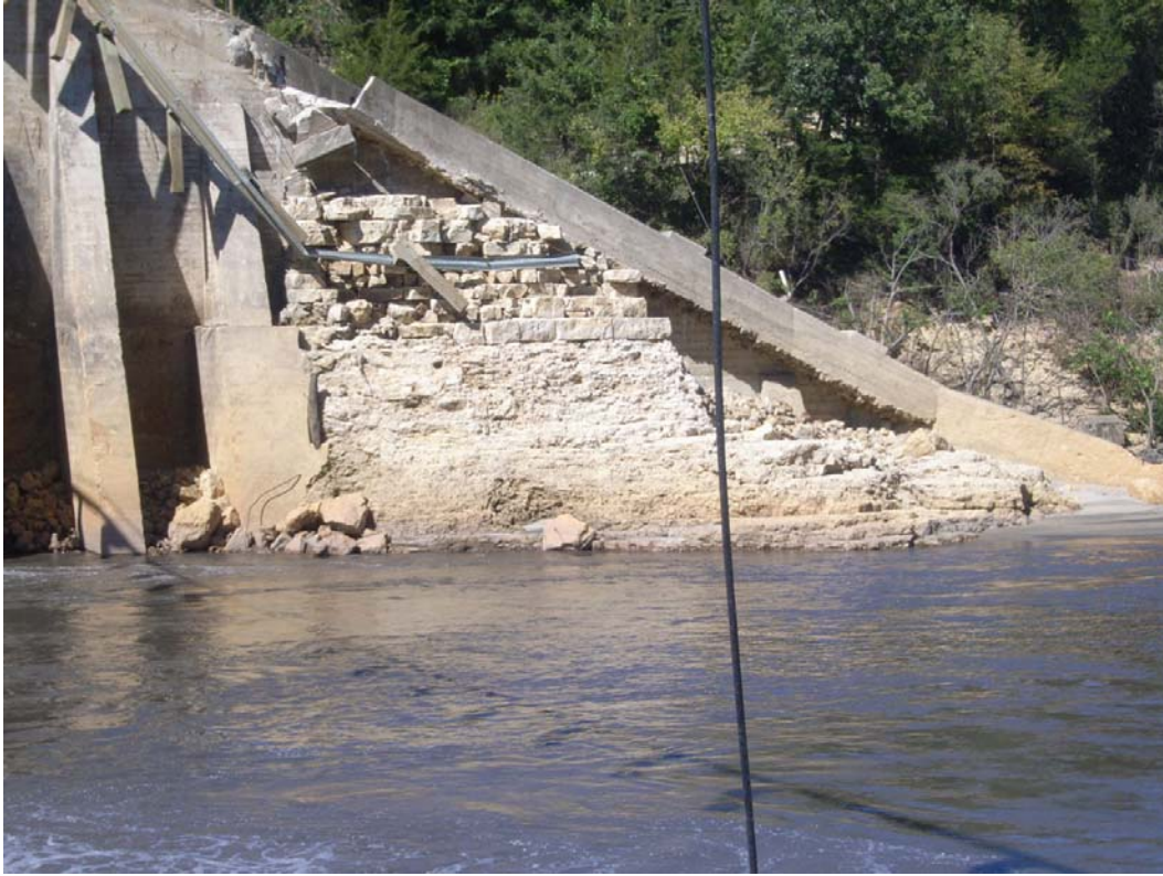
Photo IV-5 Close up of the old bridge pier and fishway remnant.
