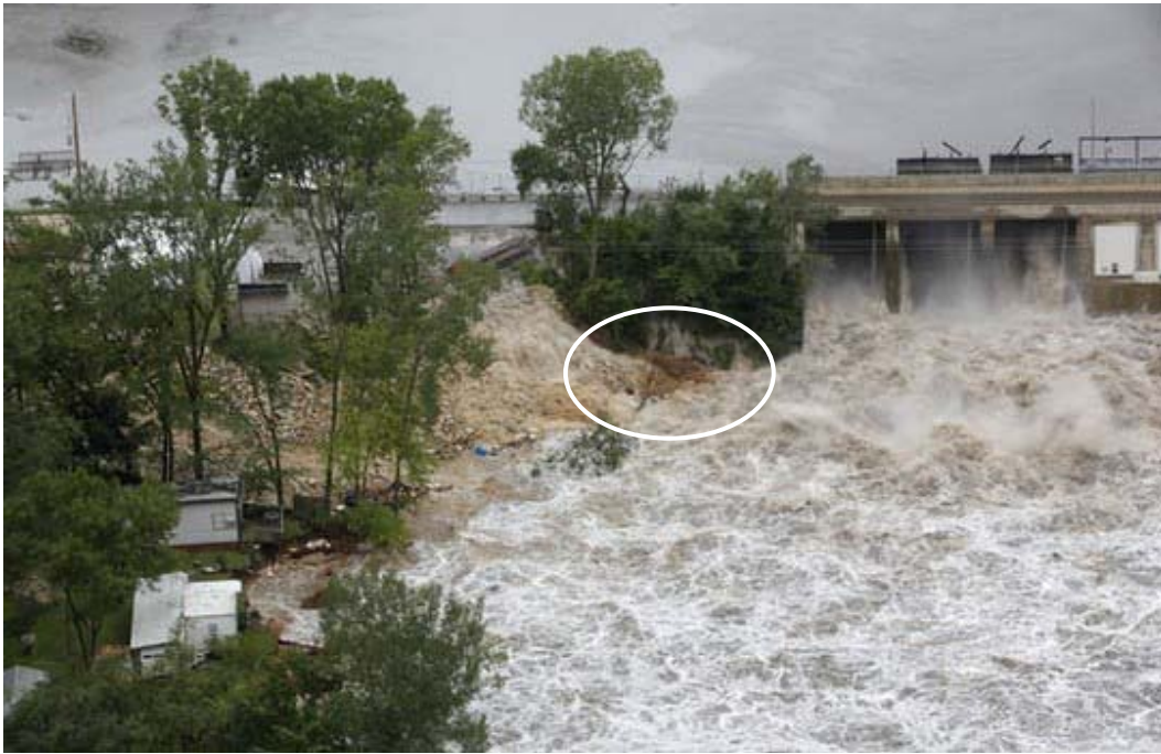
Photo IV-9 Discolored discharge emerging near toe (DesMoinesregister.com).
