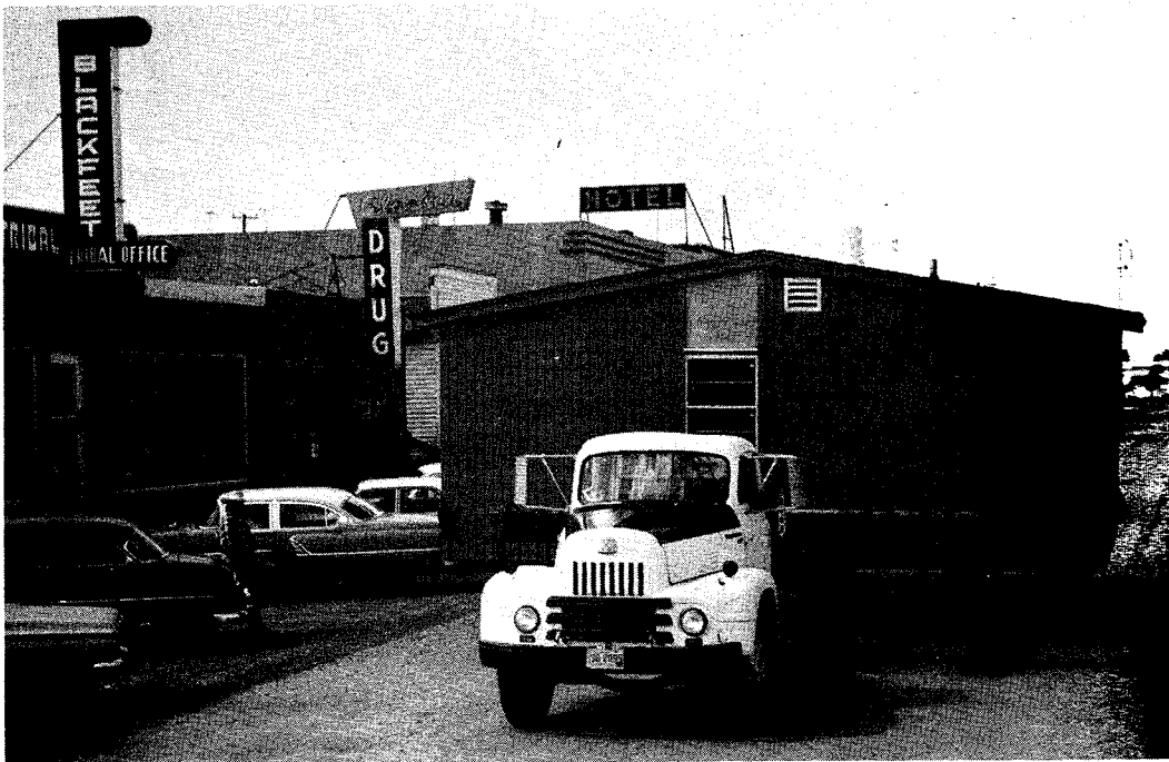
A NEW HOME for a flood refugee family is hauled down Browning's main street. More than 125 homes were destroyed or damaged beyond repair, and are being replaced.
