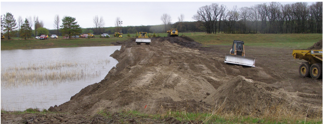
Figure 29: Construction of Temporary Fuse Plug across the Auxiliary Spillway Crest of Renwick Dam
