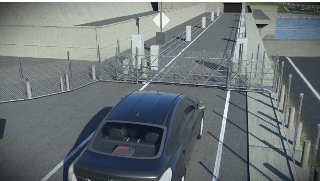
Figure C3: Inset 1 from Figure C2 (Active Vehicle Barrier)
