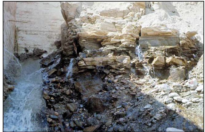
Figure 7B. Seepage emerging from the shale formation along the left side of the spillway chute, July 28, 1965.
