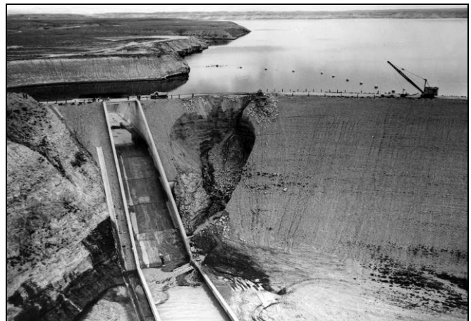
Figure 8B. A wider photo of the large unstable area on the left side of spillway chute, September 17, 1965.
