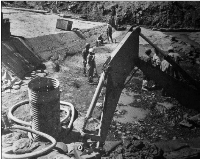
Figure 14A. Construction photo from Ririe showing dental concrete and foundation cleanup.
