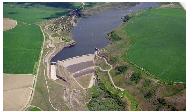
Figure 9B. Photo of Ririe Dam from 2006.
