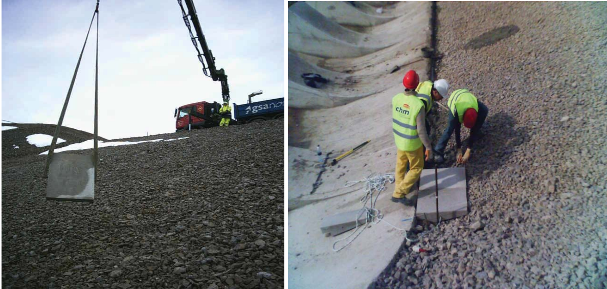
Figure Barriga-9.—Crane passing down a block and placement of the first block at the flip bucket (courtesy of Morán and Toledo, 2006, all rights reserved).
