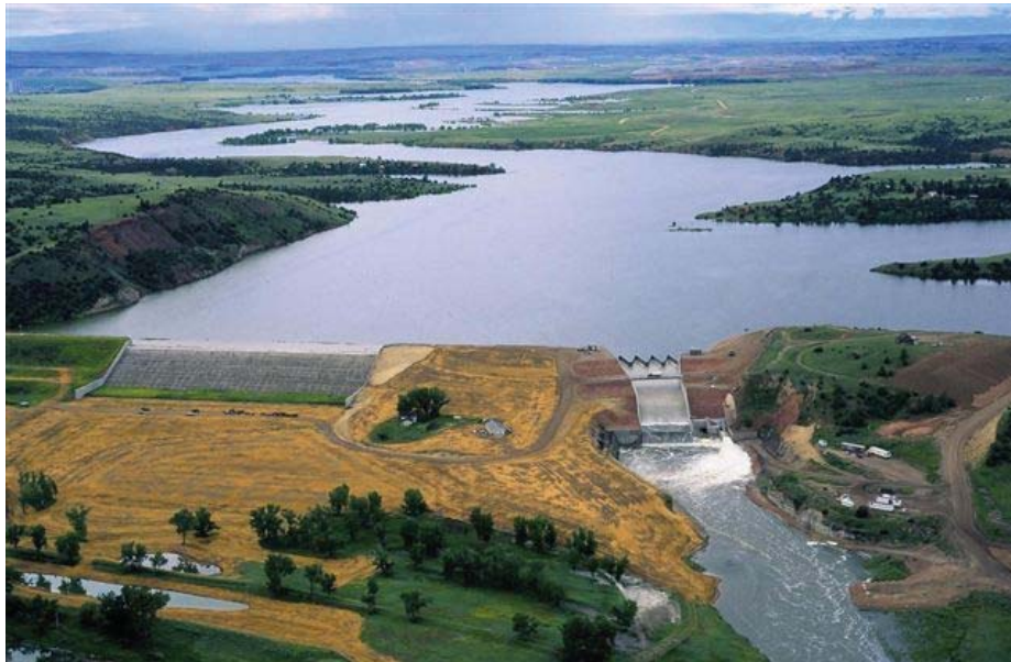
Figure Tongue-2.—Aerial view of Tongue River Dam in Montana, with service spillway shown at right and RCC overtopping protection shown at left. (Courtesy of Montana DNRC).
