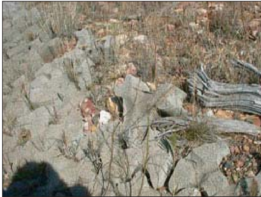
Figure Richmond Hill-4.—Typical sideslope termination with sides of mat anchored into the stockpile (Courtesy of Jacobs et al., 2004, all rights reserved).
