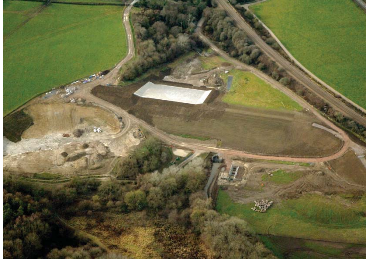
Figure Bruton- .—Aerial view of completed project.
