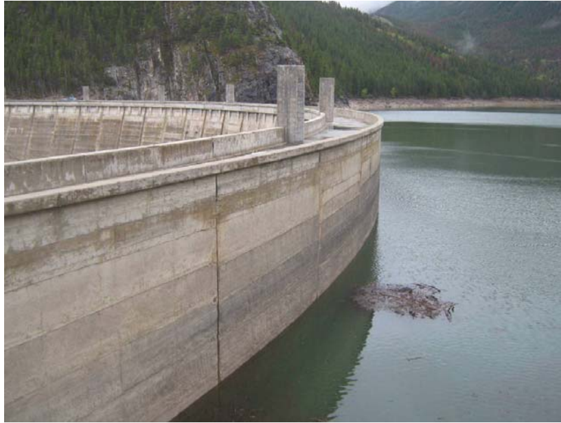
Figure 13-1.—Crest of concrete dam with splitter piers for overtopping flows (Reclamation).
