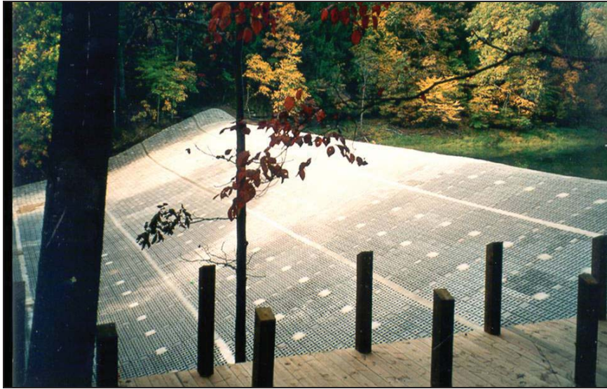
Figure Strahl-6.—Completed view of the cable-tied ACB system at Strahl Lake Dam for overtopping protection. Note all joints have been grouted (Courtesy of Contech Engineering Solutions, all rights reserved).
