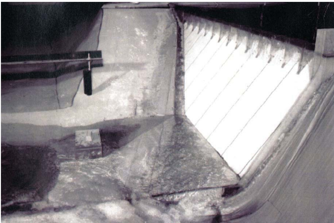
Figure Tygart-4 - Type 4 design, PMF overflow on right side of dam ( Q = 373,120 \text{ ft}^3/\text{s} ) (Courtesy of USACE, 1999)
