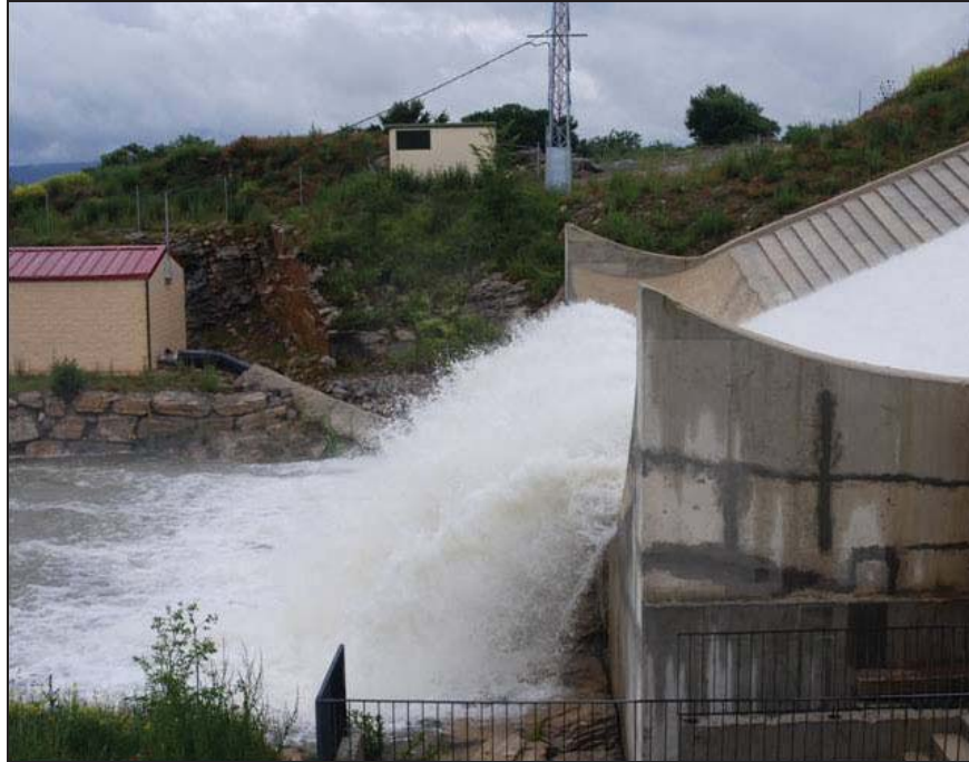
Figure Barriga-16.—Side view of the flip bucket operating (courtesy of Morán and Toledo, 2006, all rights reserved).
