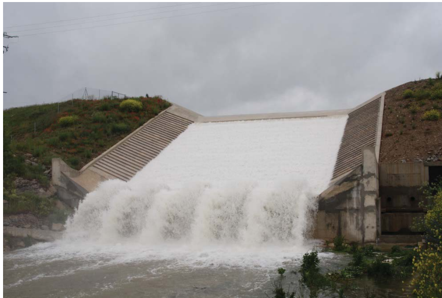
Figure Barriga-15.—Operation in May 2008 with estimated discharge of 350 - 530 ft 3 /s (courtesy of Morán and Toledo, 2006, all rights reserved).
