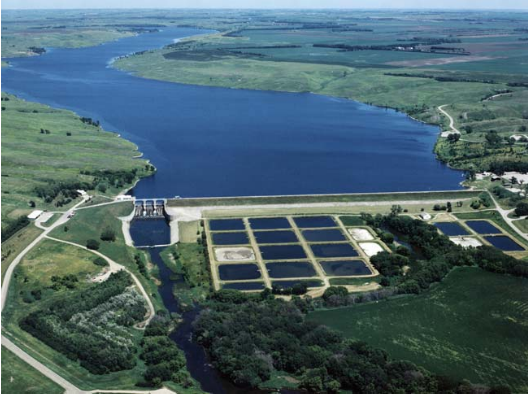
Figure Baldhill-1.—Baldhill Dam, with service spillway at the right end of the dam (looking downstream) and the uncontrolled auxiliary spillway on the downstream face of the dam (Courtesy of USACE).
