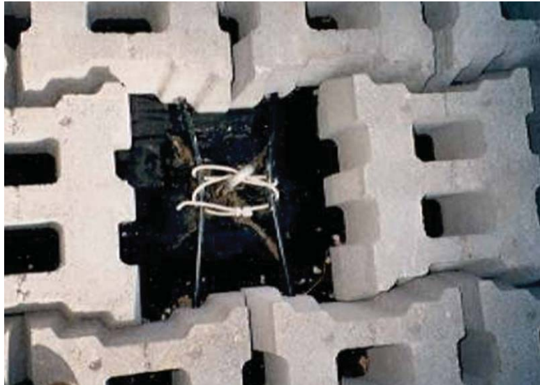
Figure Strahl-4.—Close up view of a typical tied joint prior to filling with grout (Courtesy of Contech Engineering Solutions, all rights reserved).
