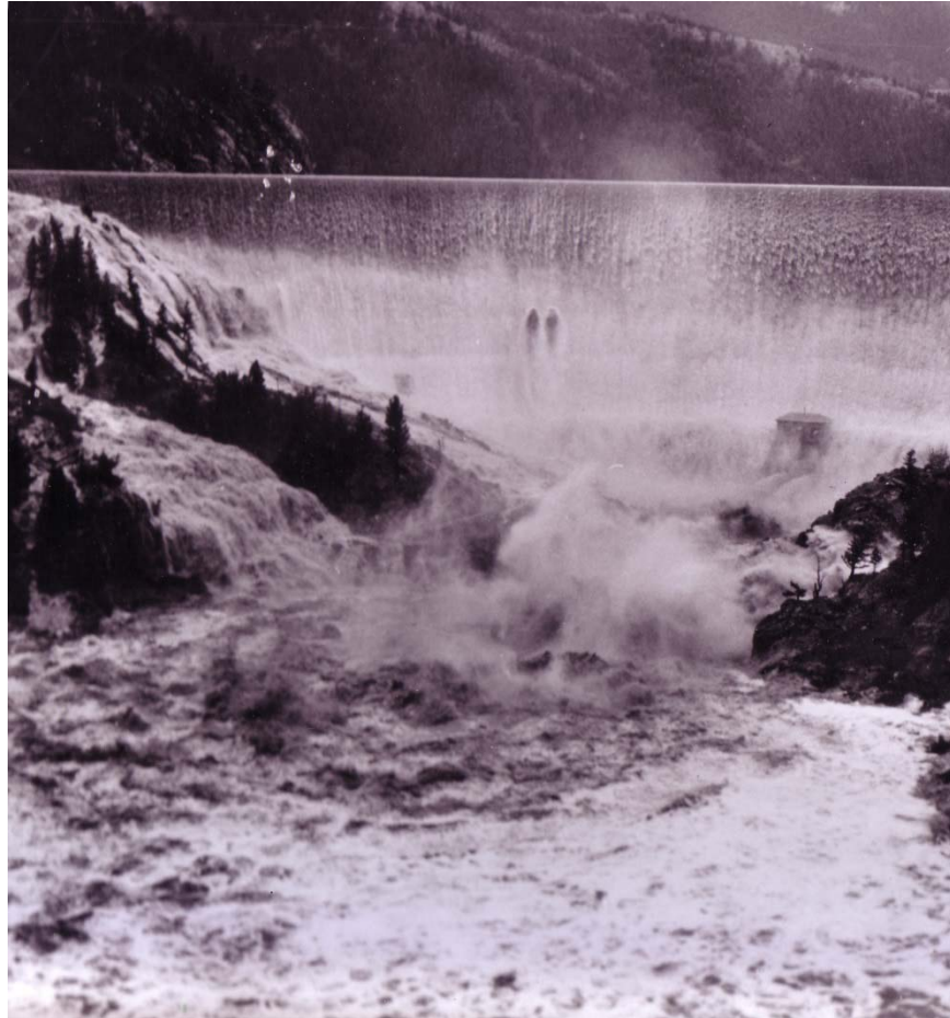
Figure 15-1.—Overtopping of Gibson Dam in 1964 by about 3 feet (Courtesy of the U.S. Geological Survey [USGS] and USFS).
