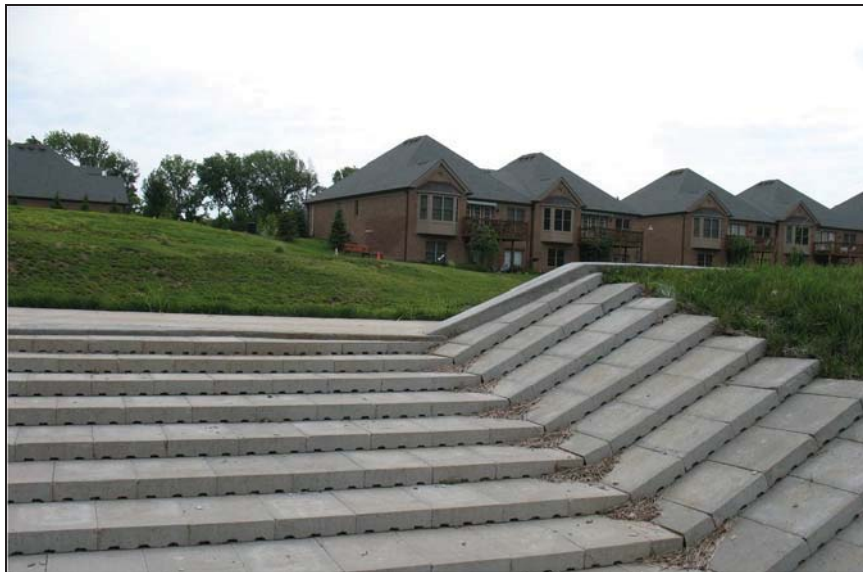
Figure Friendship Village-4.—View looking upstream toward the Friendship Village community and the finished top of spillway (courtesy of Contech Engineering Solutions, all rights reserved).
