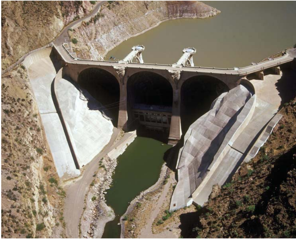
Figure Coolidge-10. —Aerial View of Overtopping Protection at Coolidge Dam (Reclamation).
