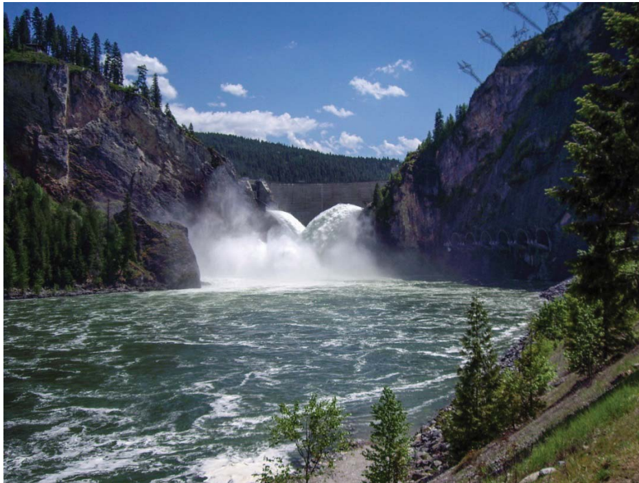
) U X U H % R X C G D U \ Test of spillway gates, May 18, 2006 (courtesy of the City of Seattle, Washington, all rights reserved).
