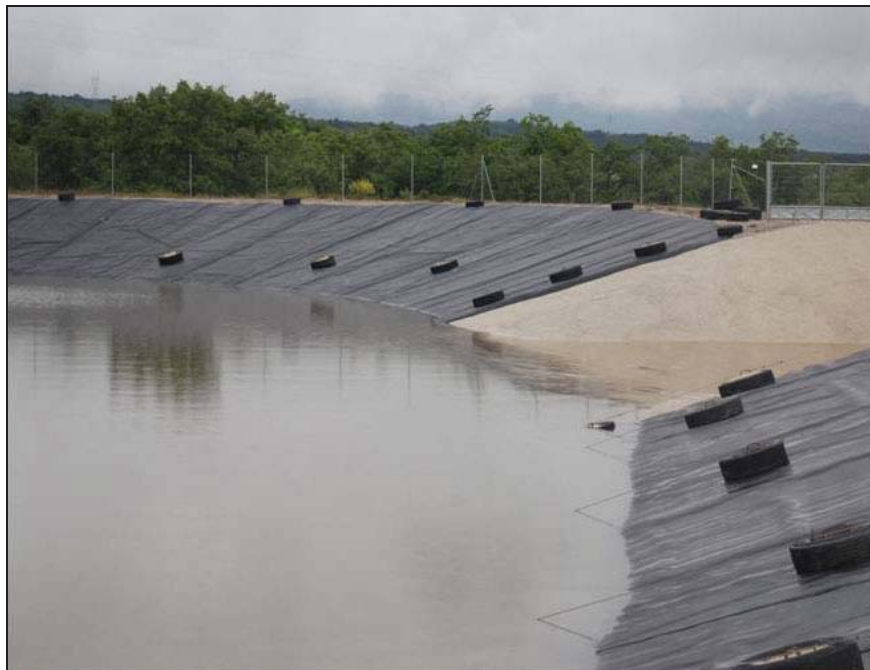
Figure Barriga-17.—View of the lined reservoir and approach conditions into the completed spillway (courtesy of Morán and Toledo, 2006, all rights reserved).
