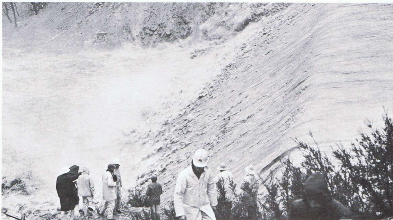
Figure Googong-1.—Overtopping of Googong Dam during construction, October 1976. (Courtesy of Engineering Heritage Canberra, all rights reserved).
