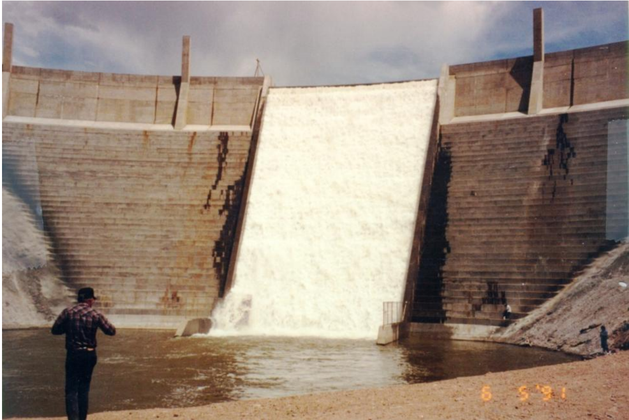
Figure 12-4.—Service spillway flows confined by training walls on stepped downstream face of Santa Cruz Dam (Reclamation).
