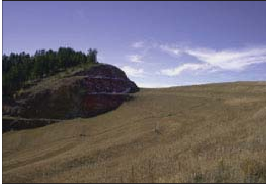
Figure Richmond Hill 1.—A downchute for conveying stormwater runoff from the Richmond Hill reclaimed overburden stockpile in the foreground (Courtesy of Jacobs et al., 2004, all rights reserved).
