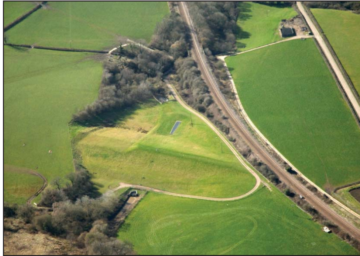
Figure Bruton-1.—Bruton Flood Storage Reservoir embankment prior to new wedge block spillway installation (Courtesy of Pether et al., 2009, all rights reserved).
