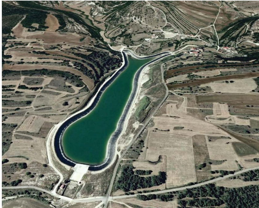
Figure Barriga-1. —Overall view of the completed Barriga Dam water storage project showing the membrane-lined reservoir and stepped block spillway in the lower left hand corner (courtesy of Rafael Morán, all rights reserved).
