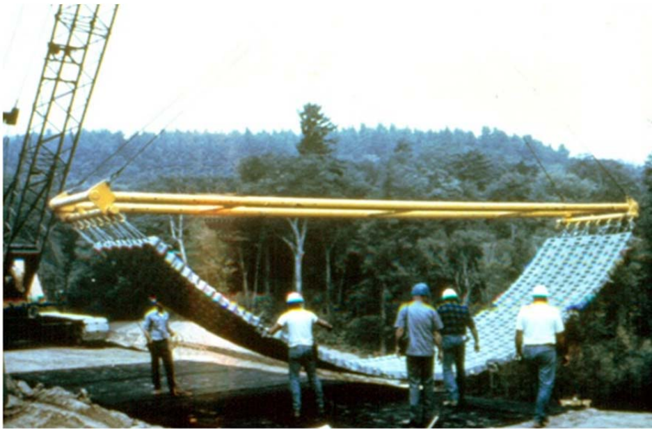
Figure 4-5.—Cabled ACB section being delivered and installed (Reclamation).
