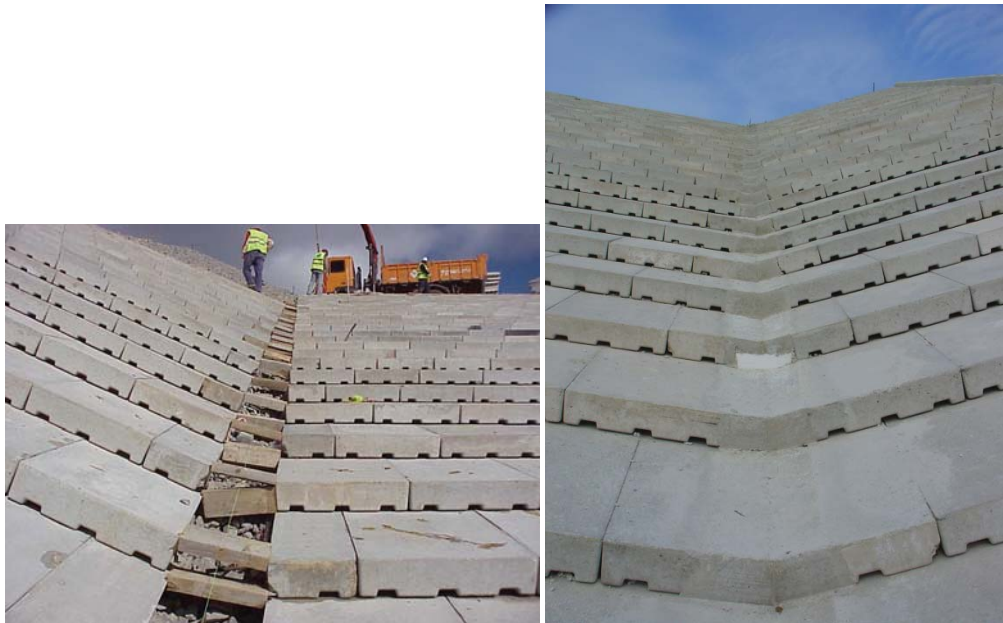
Figure Barriga-12—Views of shimmed joint on left and completed concrete transition on right between invert and side slope (courtesy of Morán and Toledo, 2006, all rights reserved).
