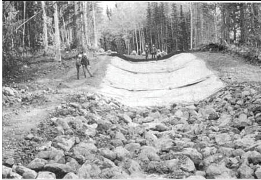
Figure Cottonwood-8.—Looking upstream at geomembrane-lined spillway (Reclamation figure republished in Timblin et al., 1988).
