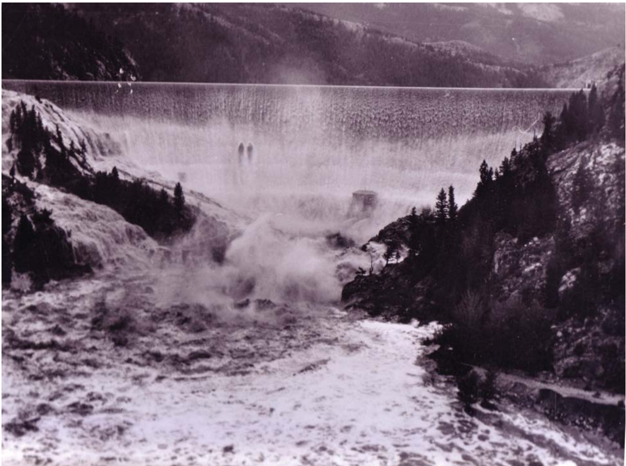
Figure Gibson-2.—Overtopping of on the Sun River, Montana, in June 1964 (Courtesy of USFS and USGS).
