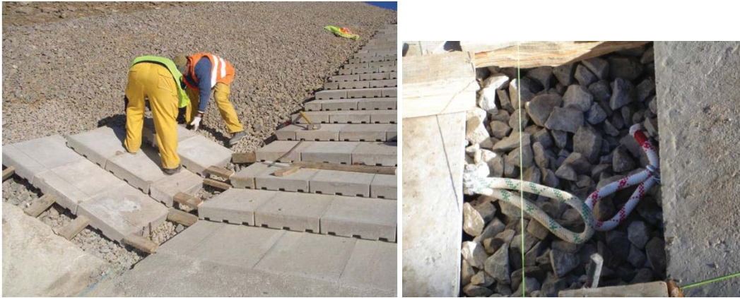
Figure Barriga-11.—View of block placement on side slope (left) and close up of rope in joint (right) (courtesy of Morán and Toledo, 2006, all rights reserved).
