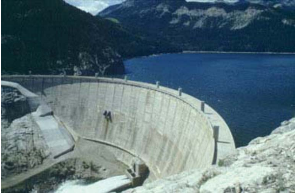
Figure Gibson-1.—Downstream face of Gibson Dam, Montana (Reclamation).
