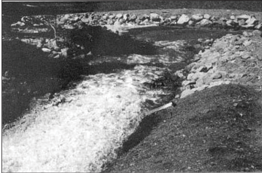
Figure Cottonwood-14.—Flow at the downstream end of the spillway as it entered the riprap basin (Reclamation figure republished in Timblin et al., 1988).
