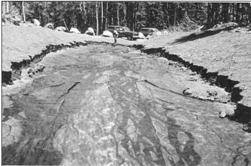
Figure Cottonwood-15.—View looking upstream at the channel after the conclusion of the test (Reclamation figure republished in Timblin et al., 1988).
