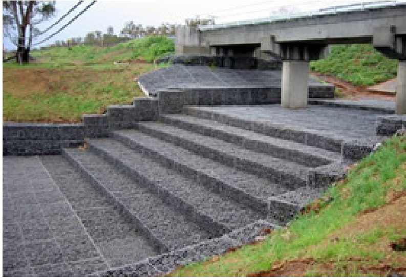
Figure 5-5.—Example of a gabion channel and drop structure. (Courtesy of Juntong Guanda, all rights reserved)
