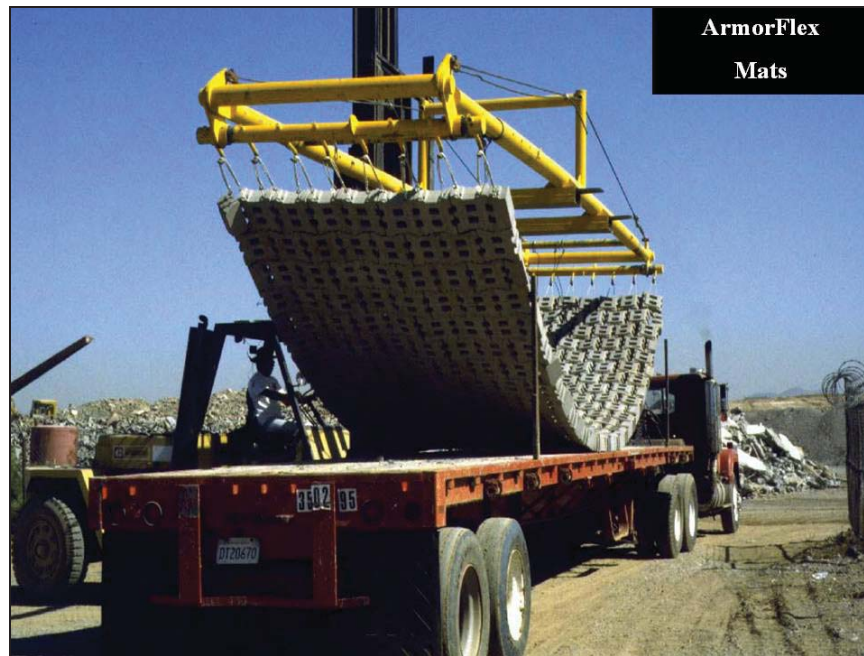
Figure Strahl 1.—Typical transport and stretcher bar, and crane, used for placing cable-tied block mats (Courtesy of Contech Engineering Solutions, all rights reserved).
