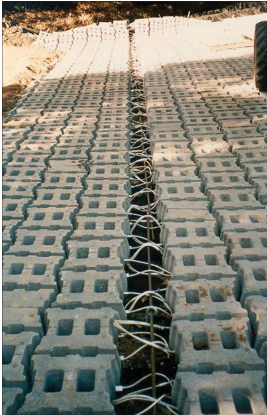
Figure Strahl-3.—View of a typical lateral joint between mats with the cables shown traversing the entire length of the system (Courtesy of Contech Engineering Solutions, all rights reserved).
