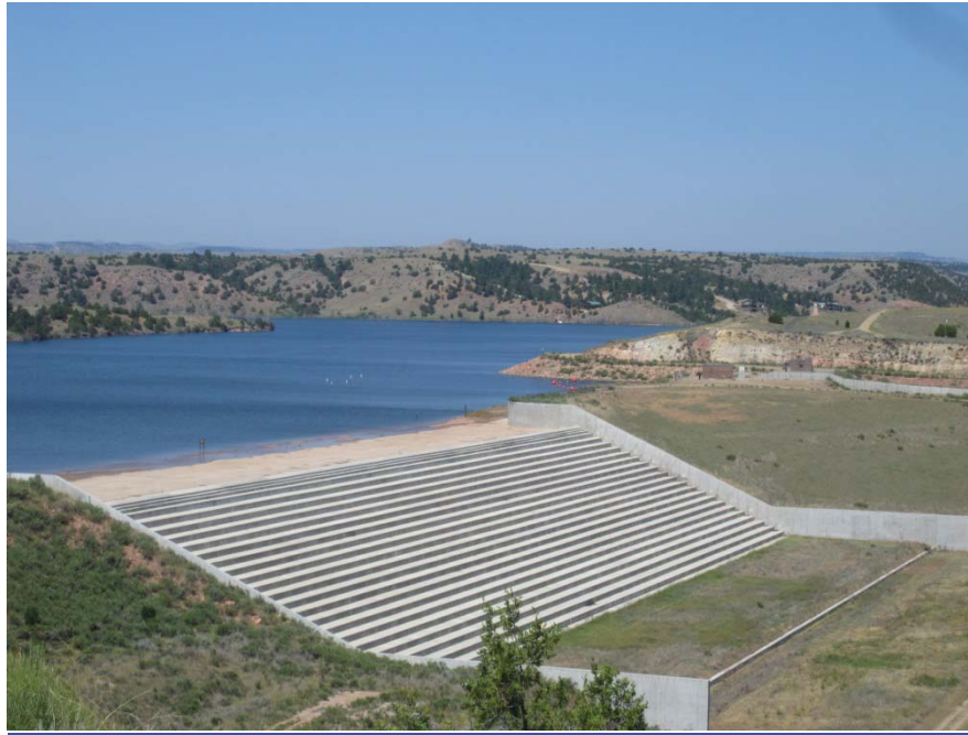
Figure Tongue-1.—Closeup view of RCC overtopping protection constructed on the downstream face of Tongue River Dam. (Courtesy of Montana Department of Natural Resources and Conservation [DNRC]).
