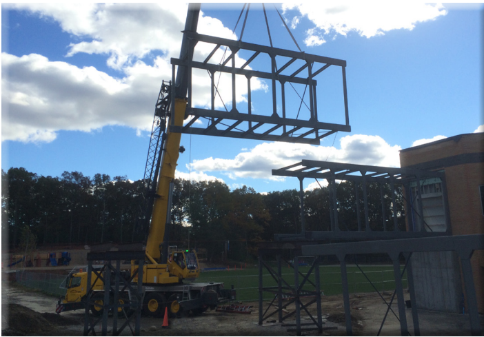
Constructing the connection bridge section by section
