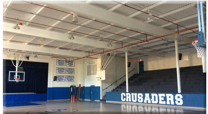
Whitinsville Christian School's existing gym/auditorium
