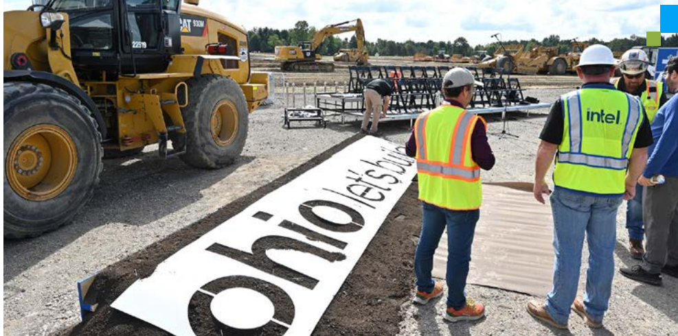
In September 2022, we celebrated our groundbreaking of two of the world’s most advanced chipmaking facilities, in Licking County, Ohio.
