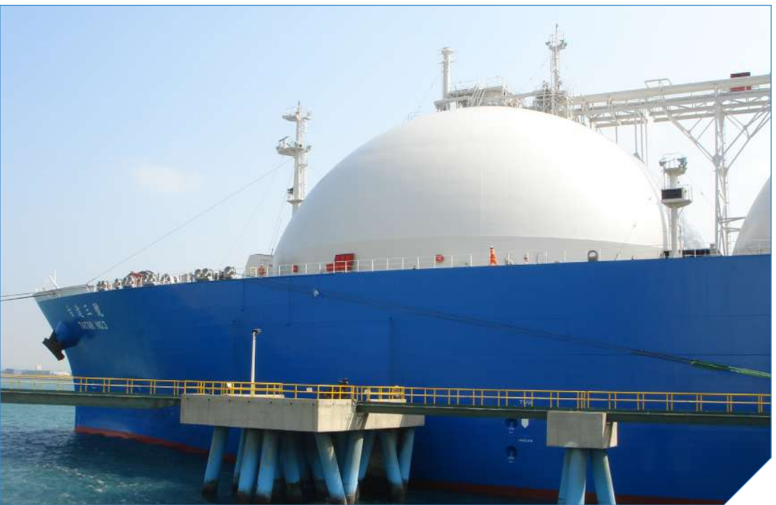
CPC Corporation LNG Taichung Receiving Station
