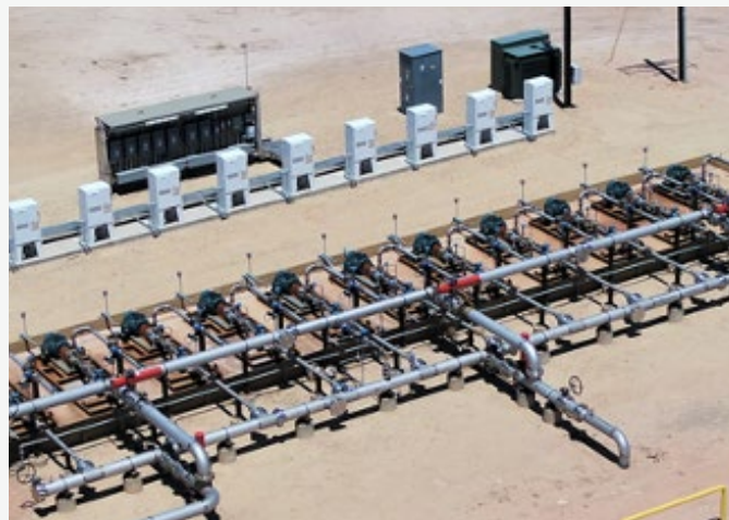
Booster Station: Part of Coterra's engineered access for water reuse
