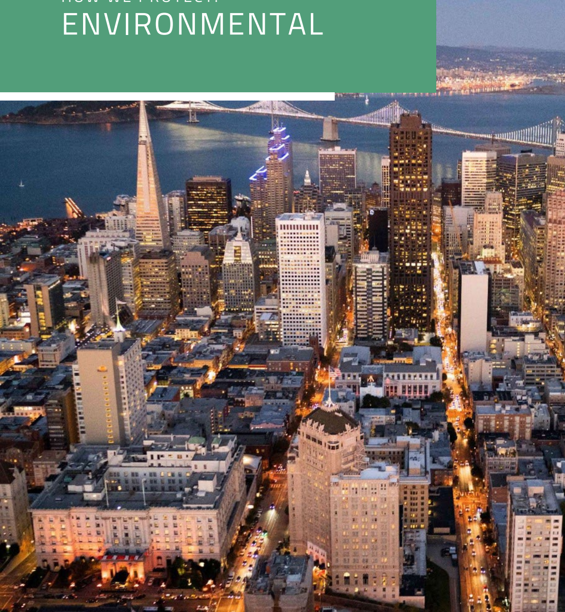
650 California Street centered within the San Francisco skyline.
