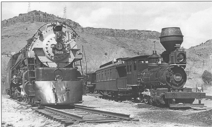
The 191 was displayed for many years in its partially restored condition beside Chicago Burlington & Quincy O5-A No. 5629 illustrating the sharp contrast between 1880s narrow gauge locomotives and the 1940s era standard gauge giant. The folio sheet below for No. 30 is the same for No. 31. When this sheet was drawn, No. 31 had been sold. The engine is black with yellow lettering. (Photo and folio sheet from Colorado Railroad Museum collection)
