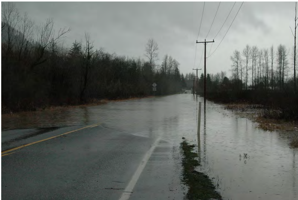
Photo credit Washington State Department of Transportation
